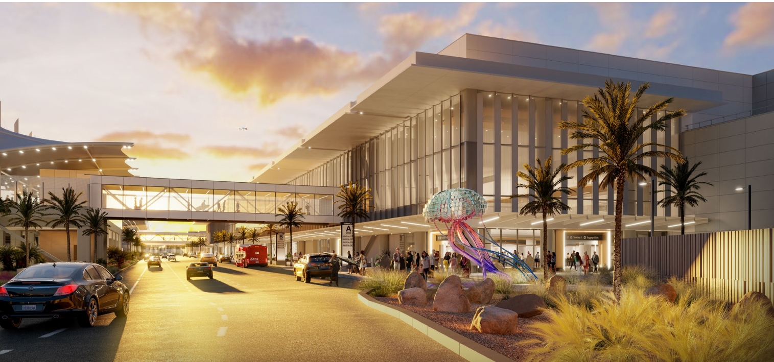
The New T1 will feature sustainable and resilient design features while contributing to operational efficiency and customer satisfaction.
