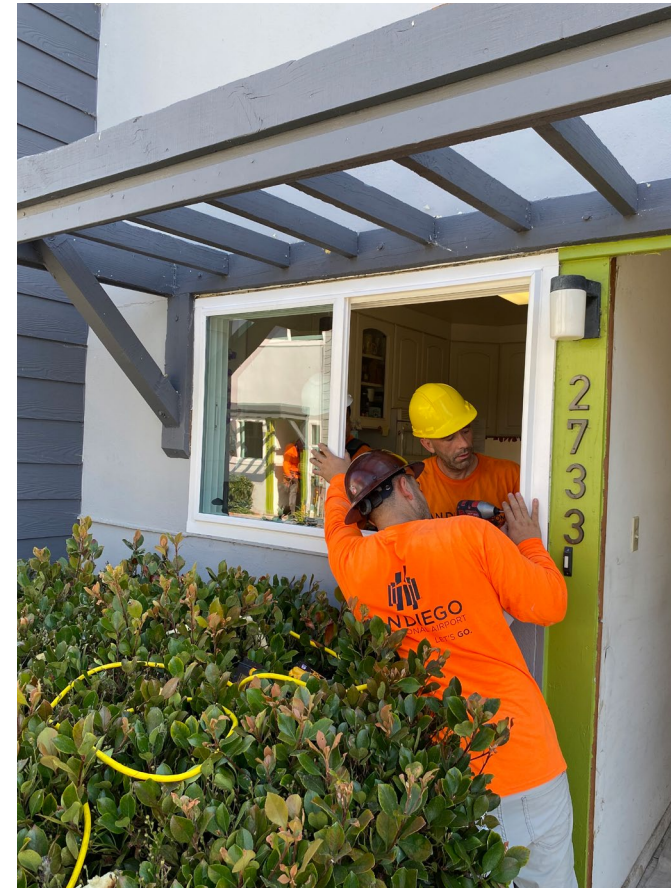
QHP contractors install new windows in a residence to reduce exposure to aircraft noise.
