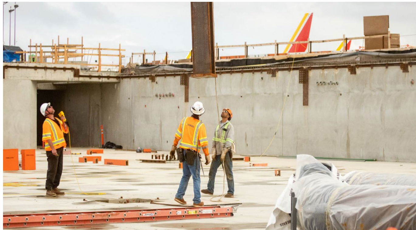
Contractors place steel structural elements of the New T1.
