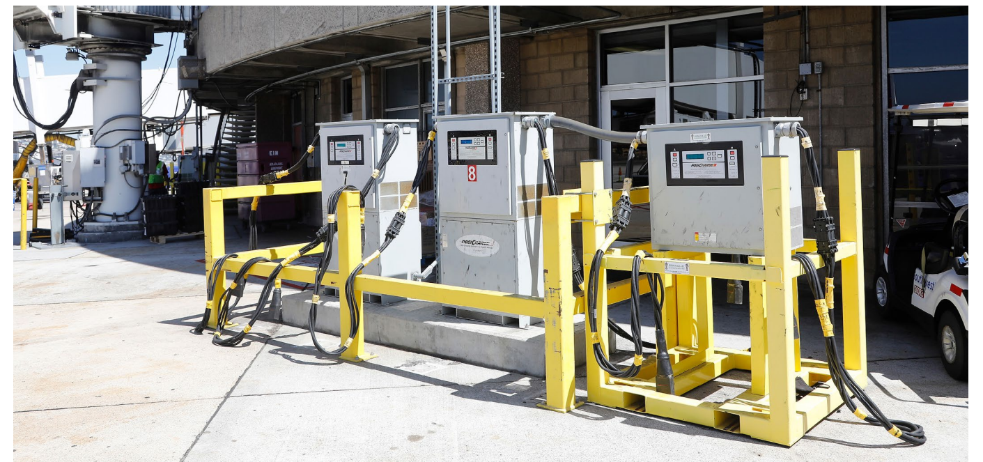
GSE chargers allow for the adoption of electric equipment that improves air quality.
