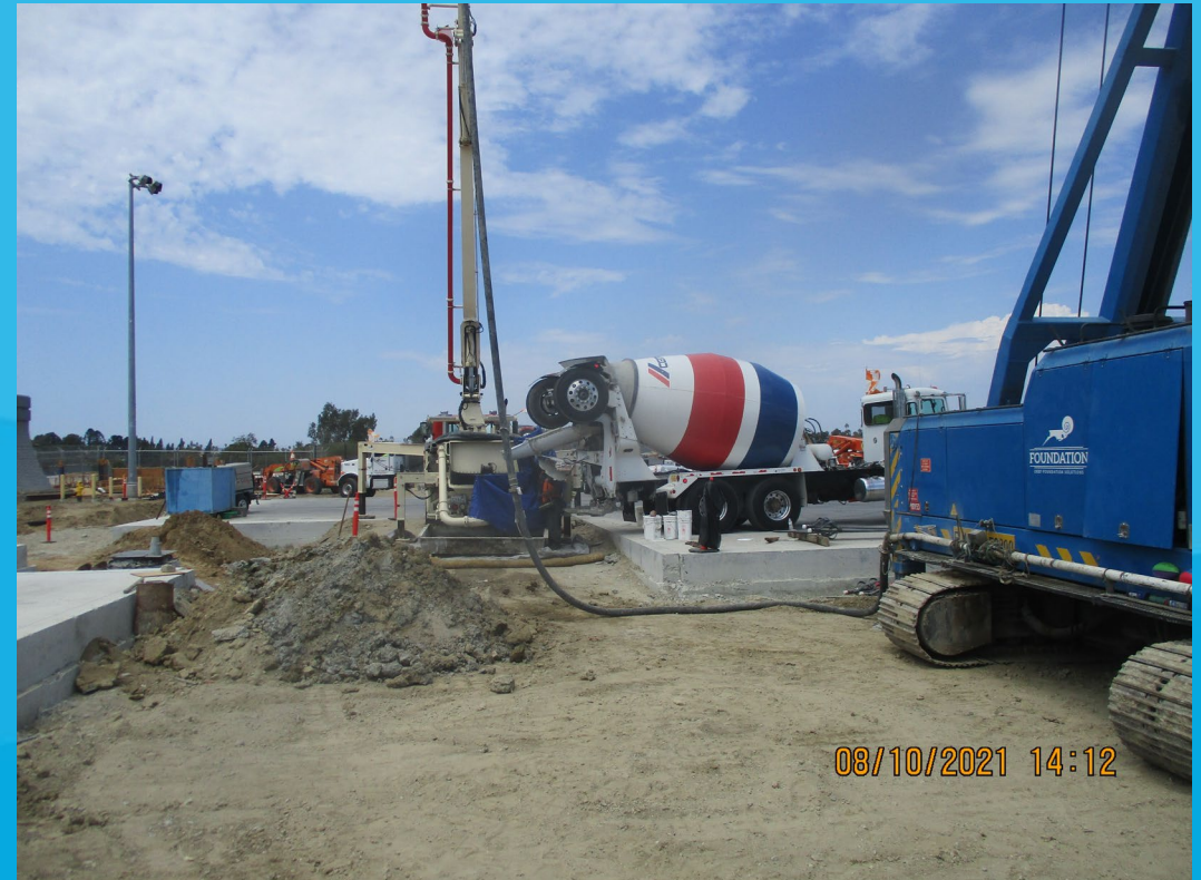
Grout Truck and Pump Truck
