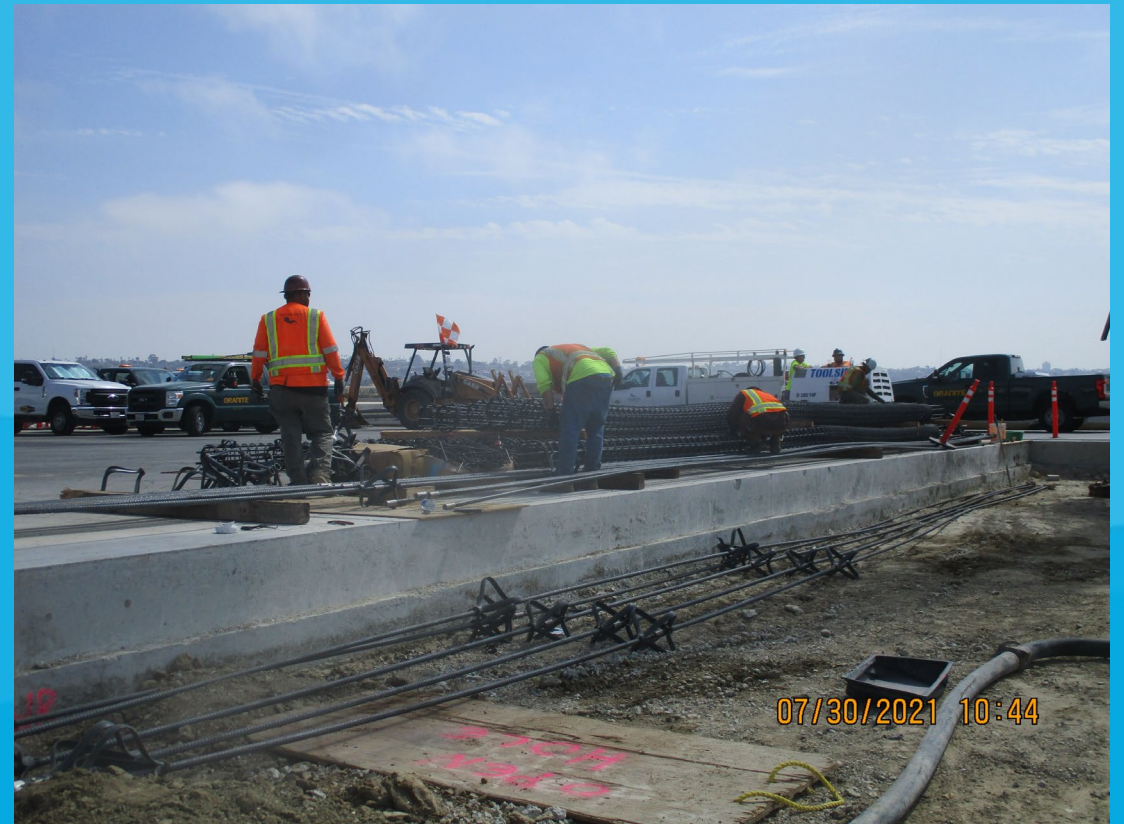
Preparing Steel Cages and Centering Rebar for Auger Cast Piles
