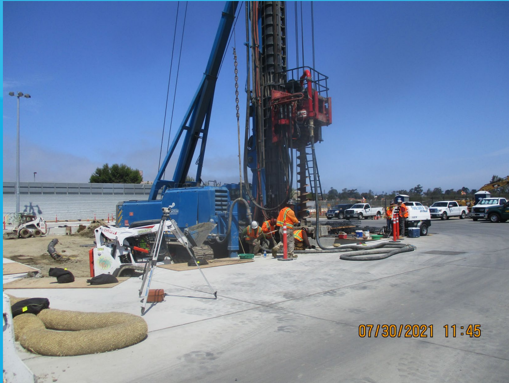
Drilling for Auger Cast Piles
