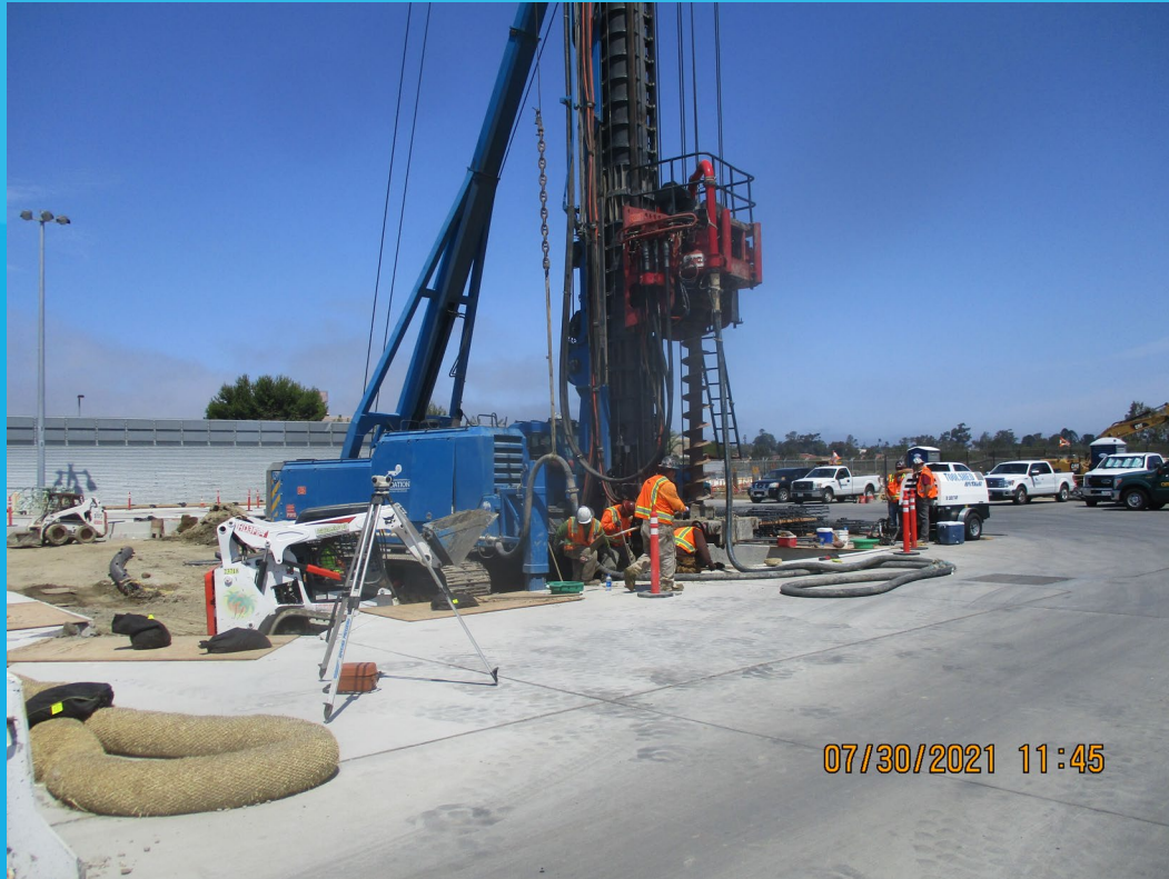
Drilling for Auger Cast Piles
