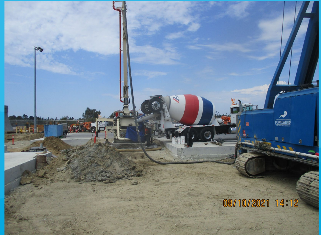
Grout Truck and Pump Truck
