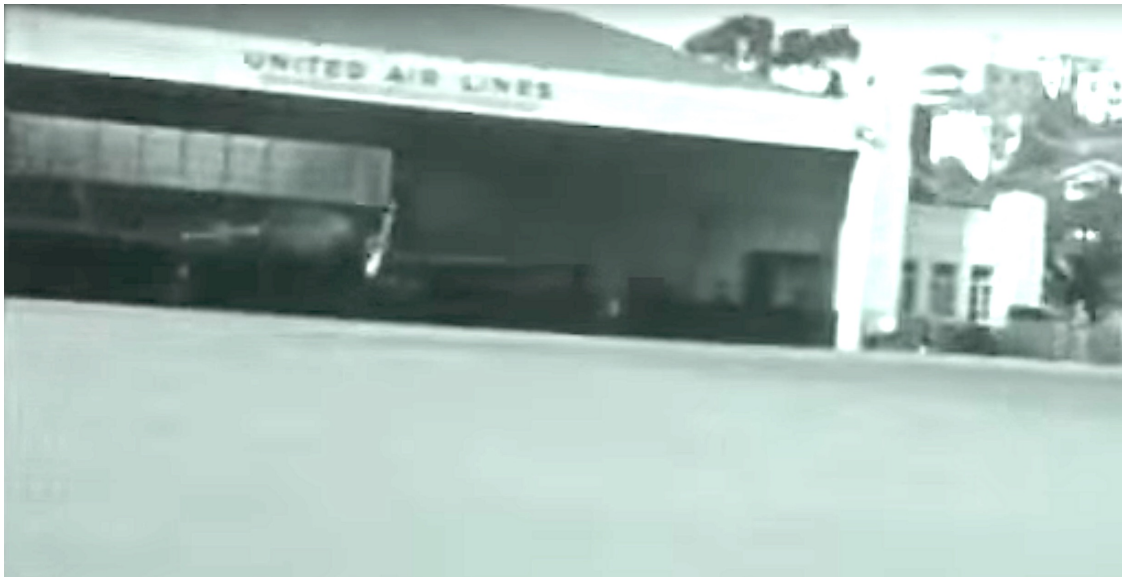
Plate 6.4–14: Circa 1931 to 1941 photograph of the interior of the UAHT building showing the attached terminal and two entrance doors on the right side. (Photograph courtesy of the San Diego Air and Space Museum)
