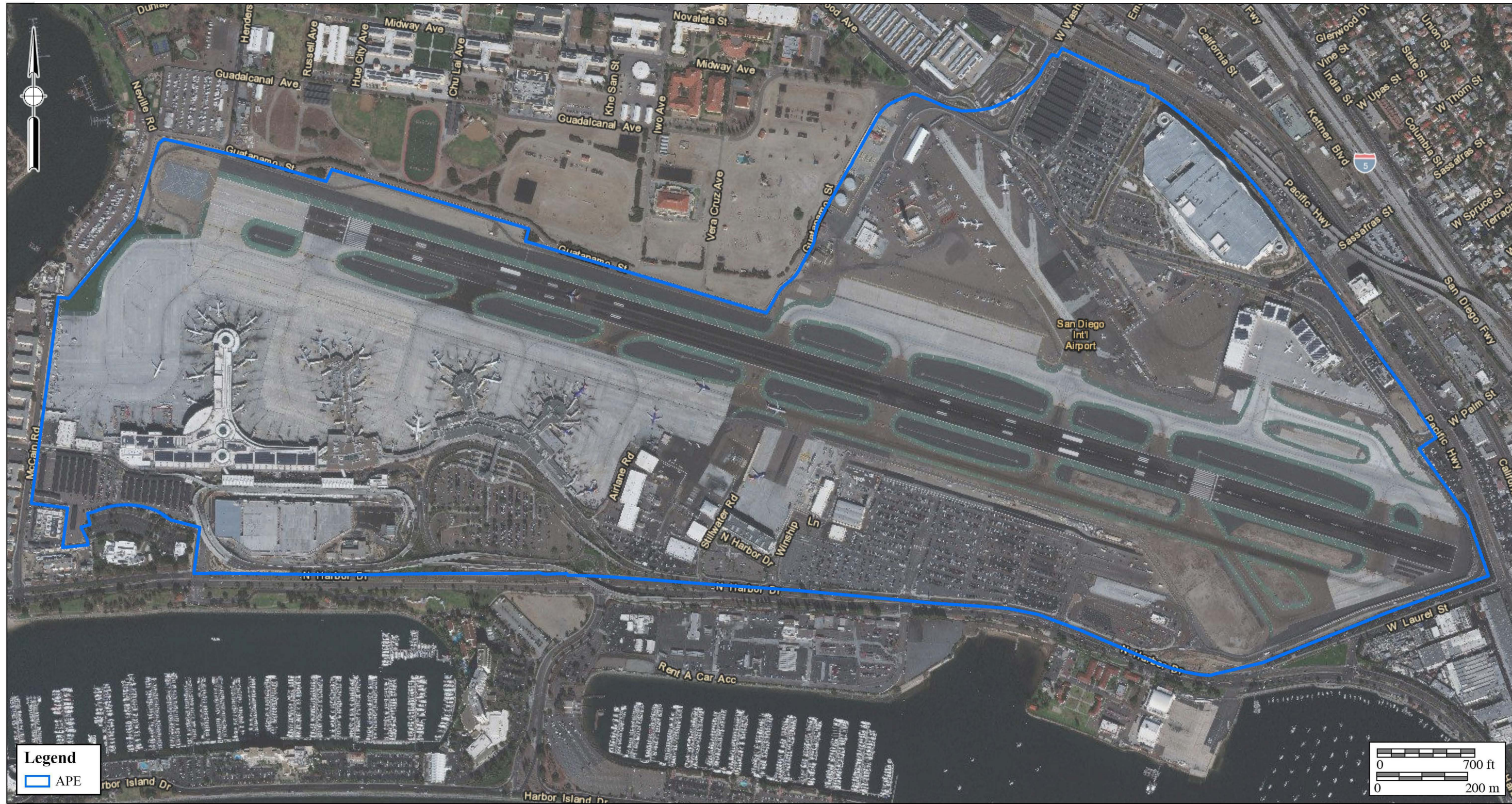
Figure 3.0-3 Area of Potential Effect The SAN Airfield Improvements and Terminal 1 Replacement Project
