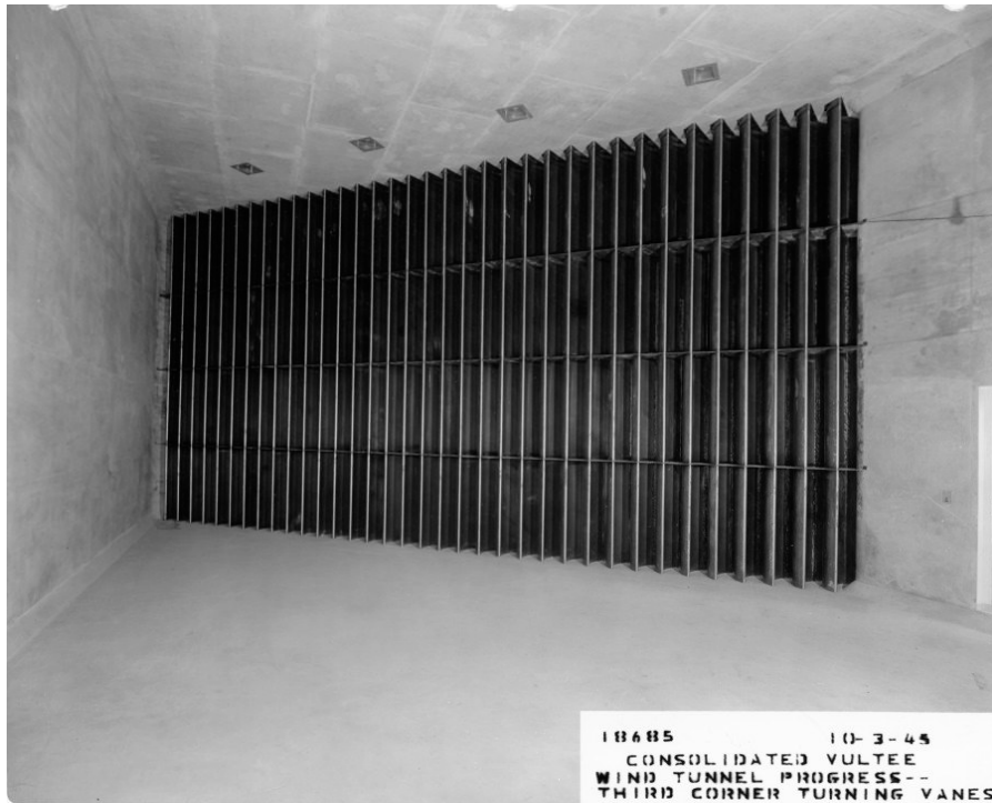
Plate 6.5-7: CWT building turning vanes in 1945. (Photograph courtesy of the San Diego Air and Space Museum)
