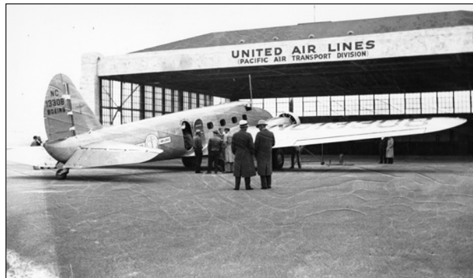
Plate 5.5–1: United Airlines hangar and terminal in 1934. (Photograph courtesy of the San Diego Air and Space Museum)
