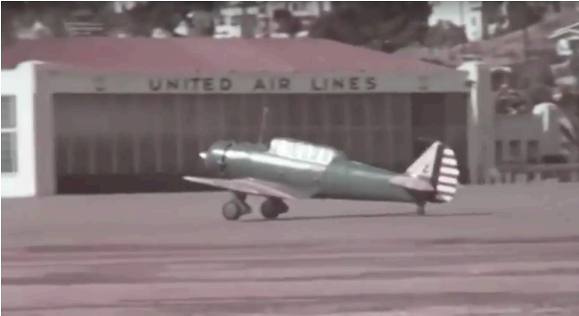
Plate 6.4–13: Circa 1931 to 1941 photograph of the UAHT building showing the terminal attached to the right side. (Photograph courtesy of the San Diego Air and Space Museum)
