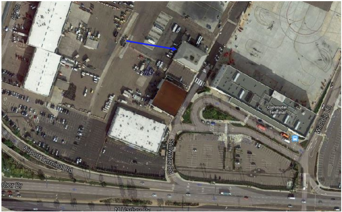
View of the Administration Building and the buildings along Stillwater Road. The blue arrow points to 2340 Stillwater Road.
