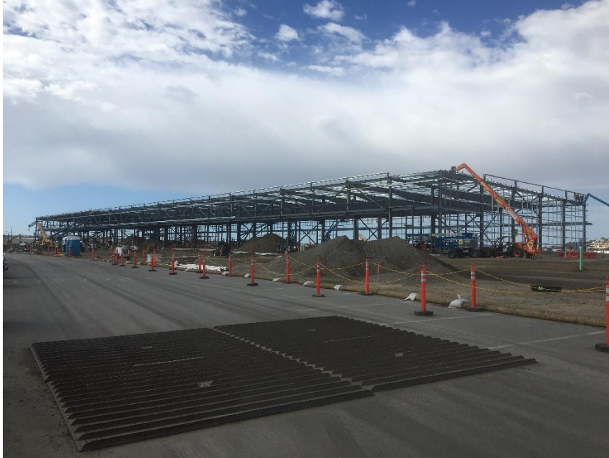
Construction progress as of March, 2020
