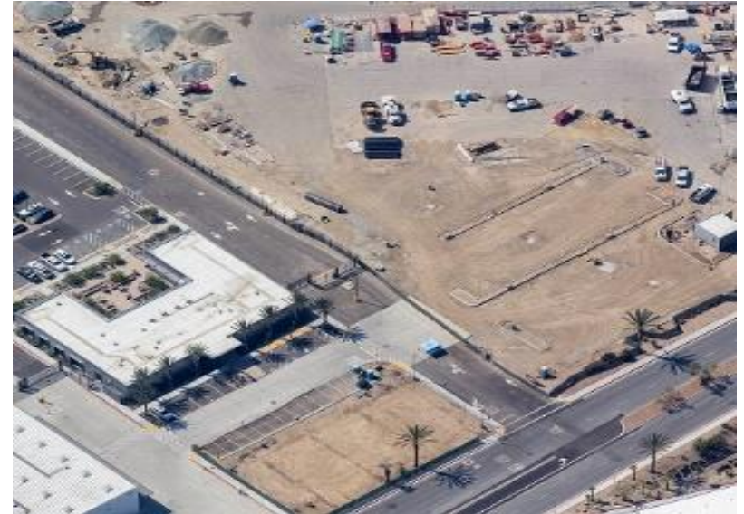
Construction progress as of October 2020
