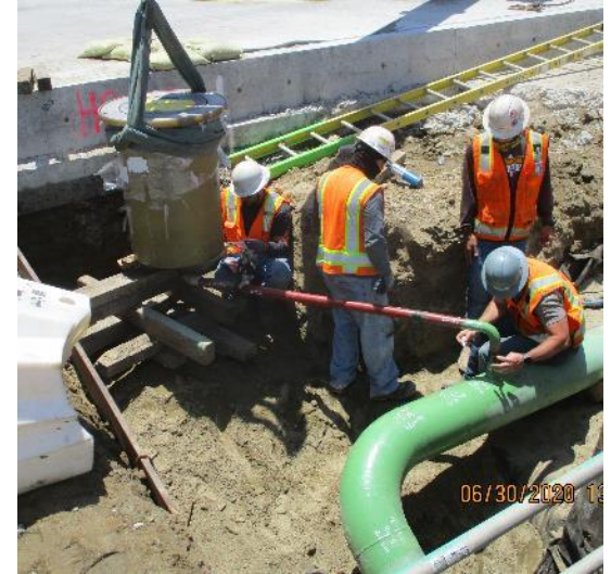
Installing High Point Vent Pit
