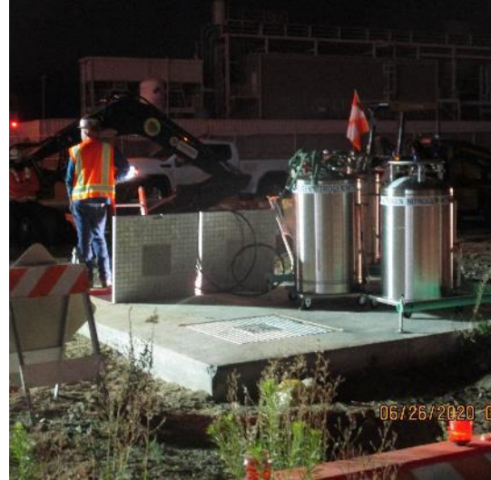
Filling Pipeline with Nitrogen for Testing
