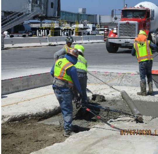
Power Screeding Low Strength Concrete
