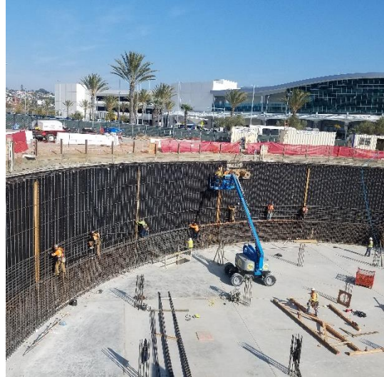
Work begins on the wall forms prior to concrete pours
