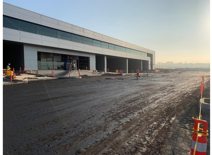
Construction progress as of October, 2020
