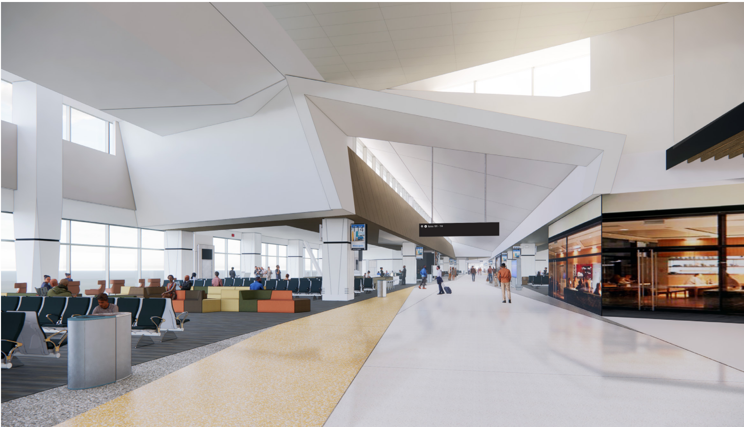
fig. 2.5.4 View of Concourse at New Terminal 1
