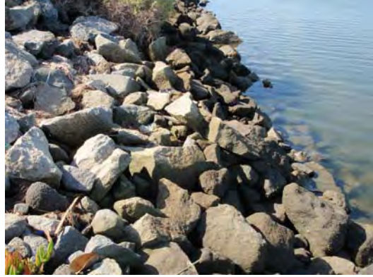
Supratidal and intertidal riprap habitat at the Project outfall site
