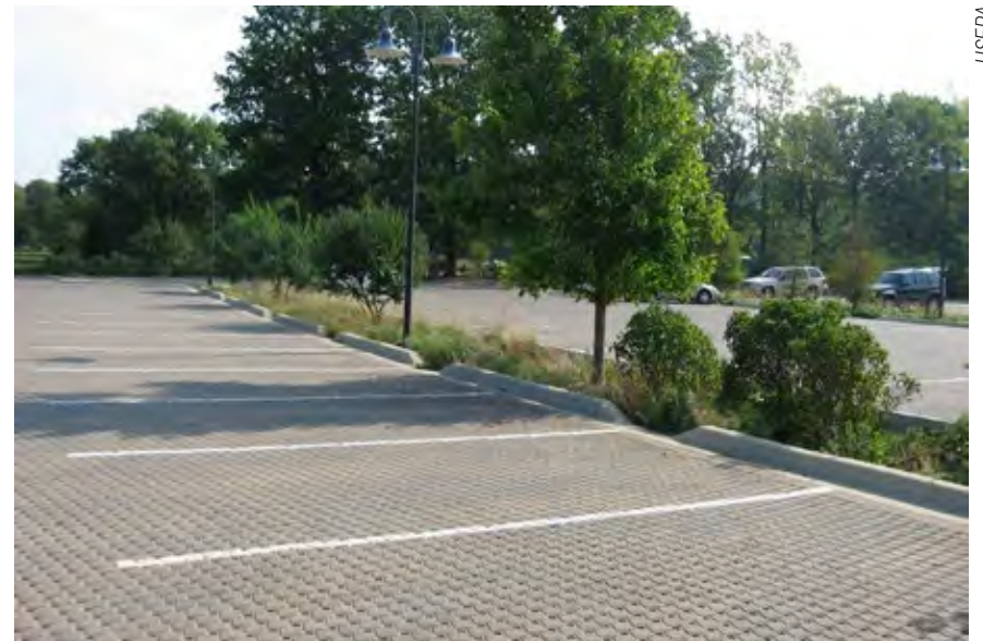
Figure 4-24. Vegetated swales were installed adjacent to a permeable parking lot in Chicago, IL, to provide overflow control and back-up infiltration as needed.
