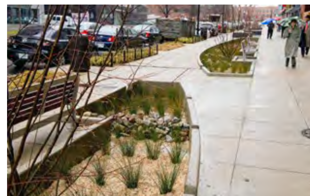
Bioretention cell in sidewalk with seating along a commercial corridor in Washington, DC.
