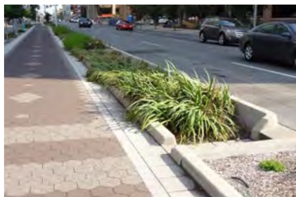
Bioswale separates sidewalks from bike lanes and vehicular traffic in Indianapolis, IN.
