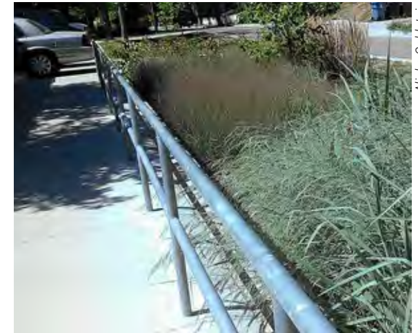
Figure 4-34. Fence protects pedestrians from the drop in grade in the adjacent bioretention feature in Minneapolis, MN.
