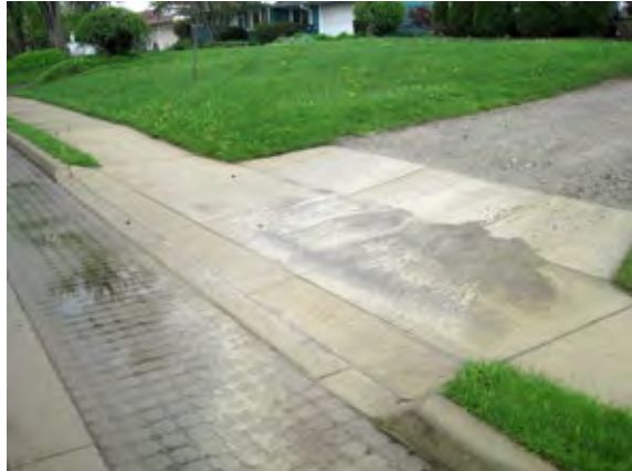
These permeable pavers received runoff from a gravel driveway and became clogged with sediment.
