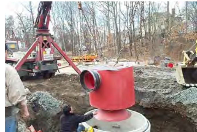
Vortex separator being installed.
