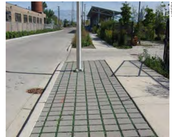
Figure 4-32. Tumbled green glass fills the spaces between permeable pavers in a sidewalk area in Chicago, IL.
