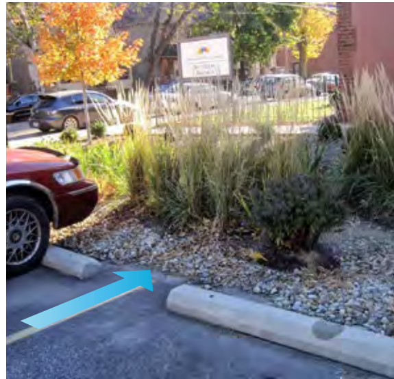
Figure 4-5. The space between adjacent wheel stops allows stormwater runoff to enter a vegetated swale in a parking lot in Cleveland, OH.
