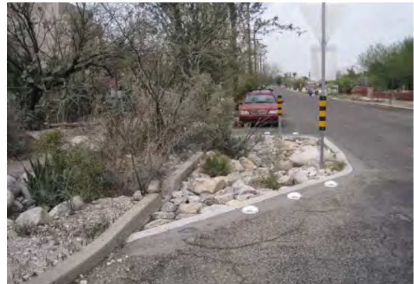
Black and yellow-striped bollards placed around a stormwater curb extension ensures safety for motorists in Tucson, AZ.
