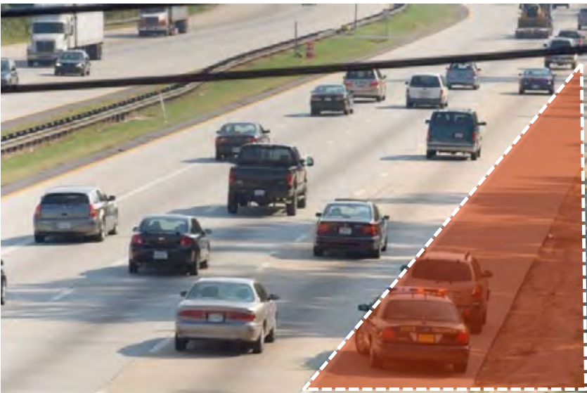
Figure 2-8. Green elements such as a swale, permeable pavement or a permeable friction overlay can be added in the verge area (roadside zone).
