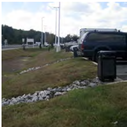
These trash cans, installed in front of stormwater inlets, block flow.
