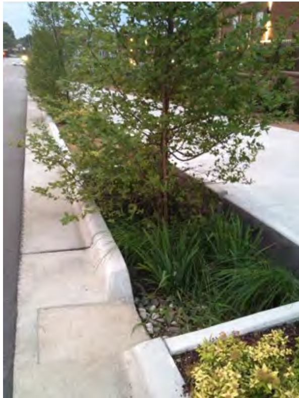
Roadside bioswale with curb-cut inlet in Greensboro, NC.
