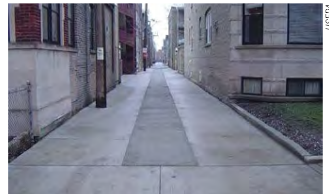
Pervious concrete trench in the center of an alley, Chicago, IL.
