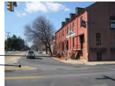
Figure 2-15. This simple road diet shows how two travel lanes are removed and replaced with one turn lane and two areas that could support green infrastructure practices.
