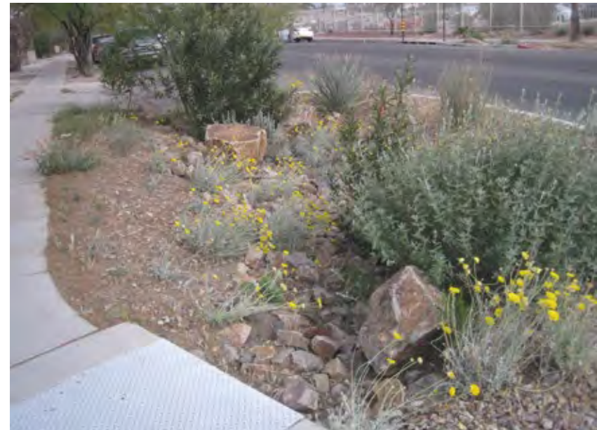
Bioswale designed with drought-tolerant plants in arid Tucson, AZ.
