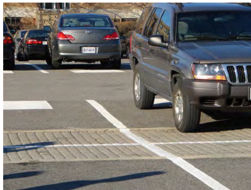
Permeable pavers installed at the downgradient end of parking bays collect surface runoff and allow it to infiltrate.
