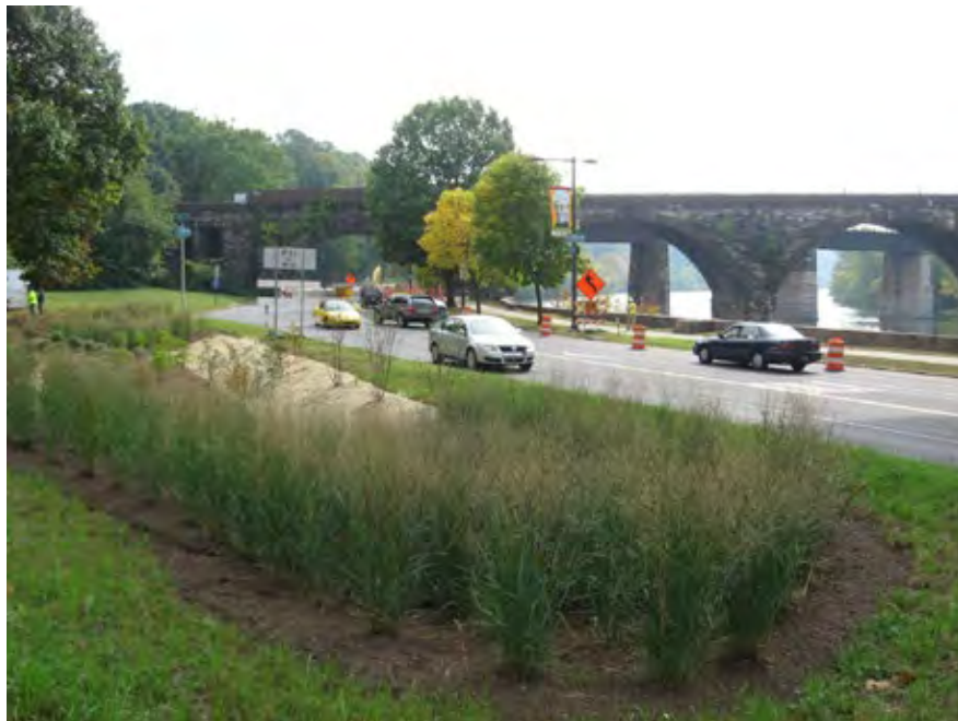
A bioretention area is located adjacent to an arterial road along the Schuylkill River in Philadelphia, PA.
