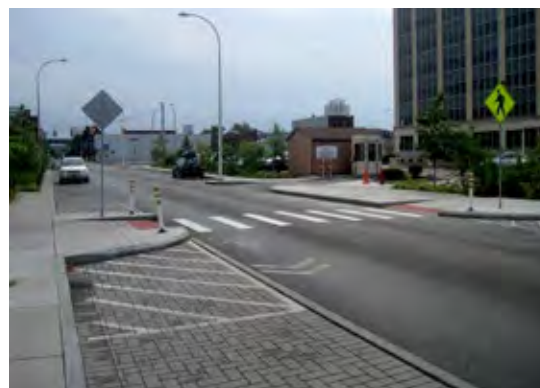
Permeable pavement parking lane in downtown Syracuse, NY.
