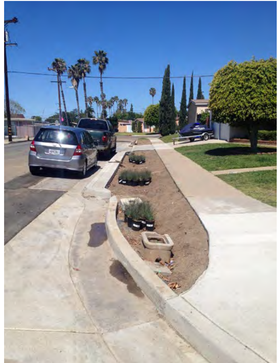
In preparation for planting local native vegetation, a soil media mix was chosen and backfilled into this roadside bioretention area in San Diego, CA.
