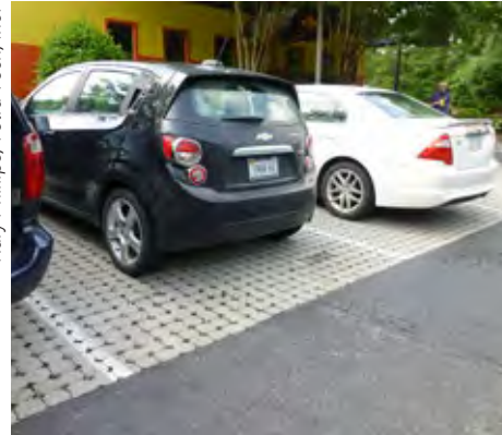
Permeable pavement in parking stalls in Williamsburg, VA.
