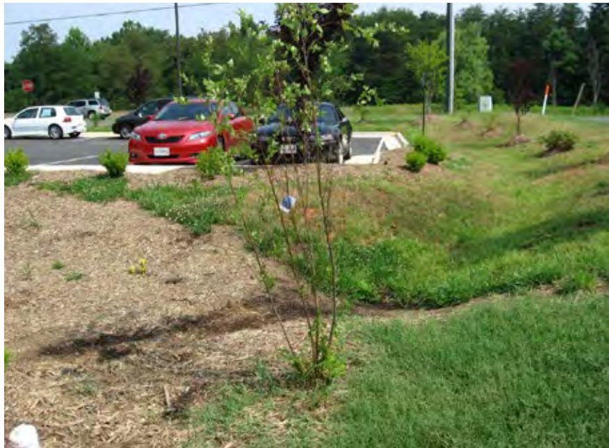
A pretreatment bioswale conveys and treats runoff from a parking lot and road in Stafford, VA.
