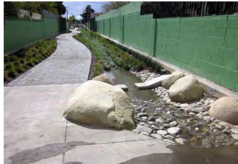
Figure 4-14. A sediment forebay with weir helps trap sediment and control flow volume in an alleyway bioswale in Los Angeles, CA.
