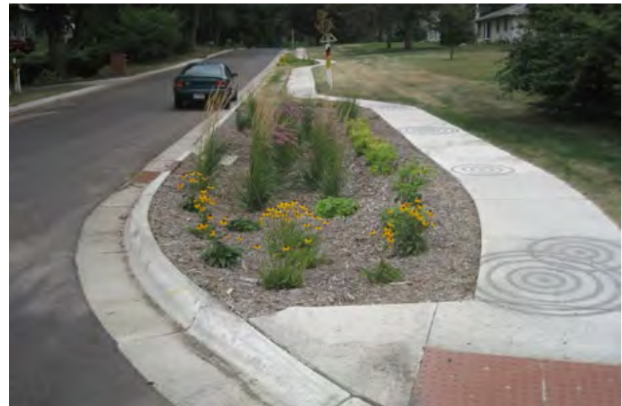
Stormwater curb extension installed with a sidewalk project in Maplewood, MN.
