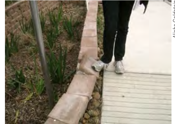
These unsecured blocks installed next to a bioretention area pose a safety risk.
