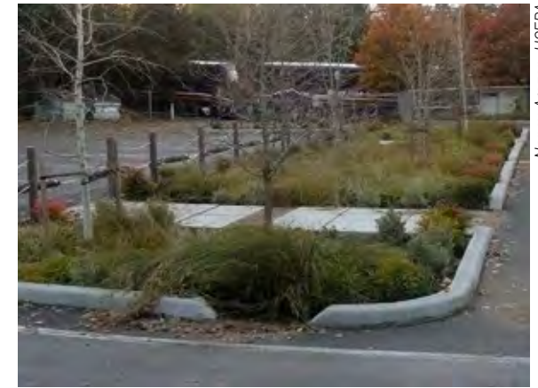
Figure 4-30. Walkway built across vegetated swale to allow users to access their cars in Portland, OR.
