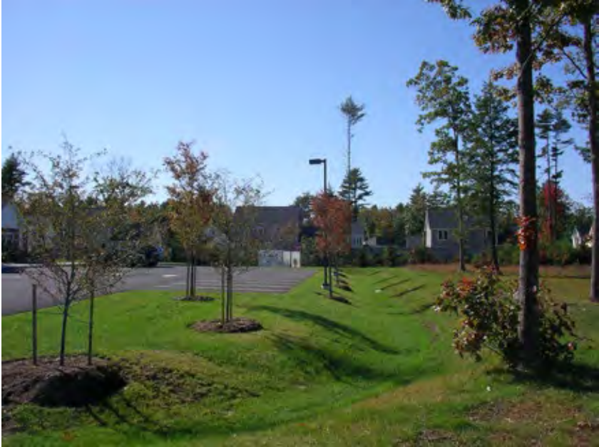
Grassed bioswale in New Hampshire.
