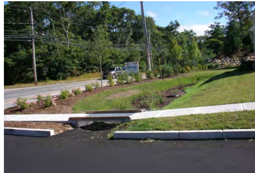
Roadside bioretention area includes a sidewalk bridge over the inlet to avoid obstructing pedestrian flow.
