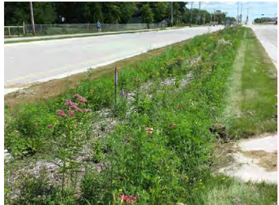
A bioretention area located in the median of an arterial road captures runoff in the Great Lakes region.
