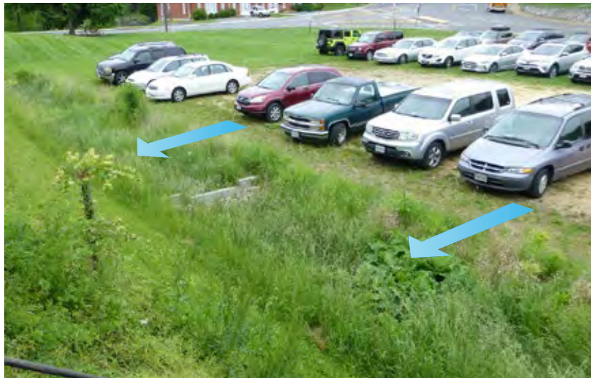
Figure 4-11. A curbsless grassed and gravel parking lot allows sheetflow stormwater runoff to enter a vegetated swale in Staunton, VA.
