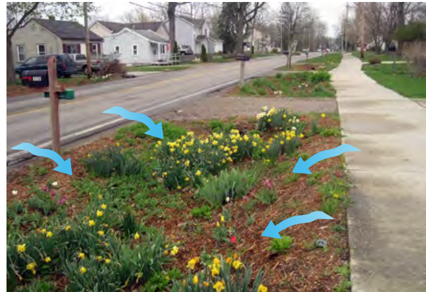
Figure 4-10. A curbsless street allows sheetflow stormwater runoff to enter the vegetated swale in Lansing, MI.
