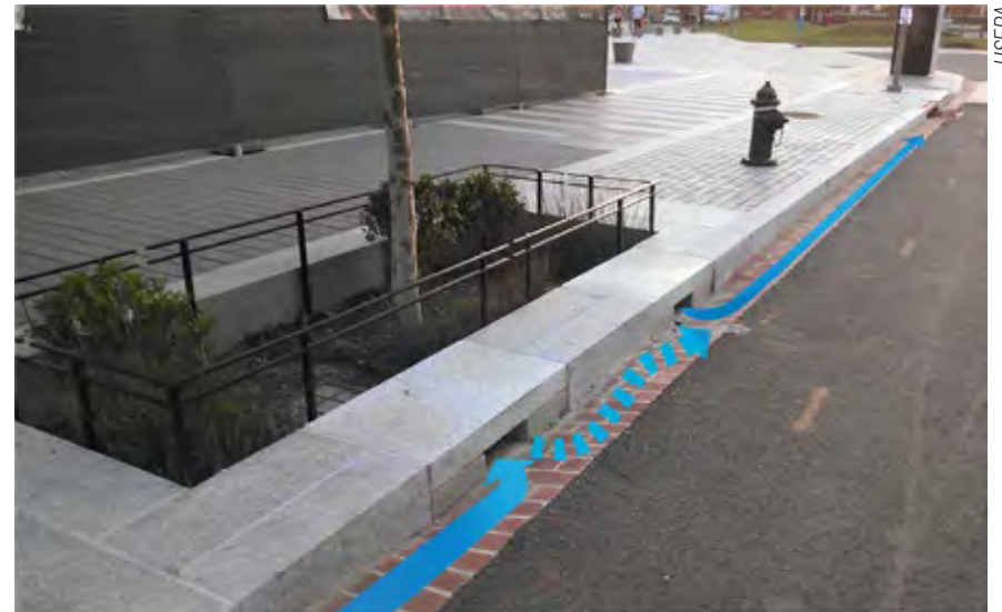
Figure 4-23. In this tree pit bypass system in Washington, DC, curb cuts allow stormwater to enter until the practice is filled, at which point additional flow bypasses the system and continues down the street to the storm drain.
