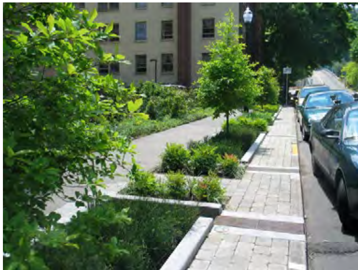
Sidewalk planters are equipped with bridges to provide access to parking areas in Seattle, WA.
