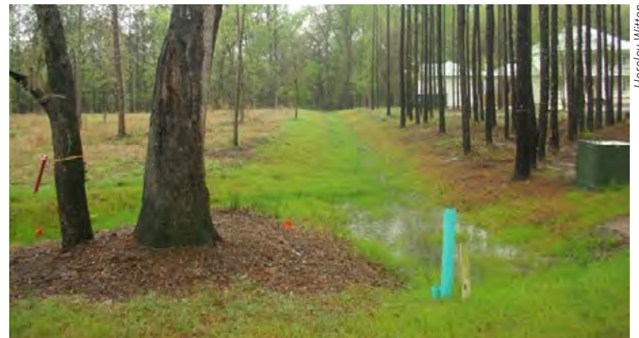
Infiltration trench with grass cover.
