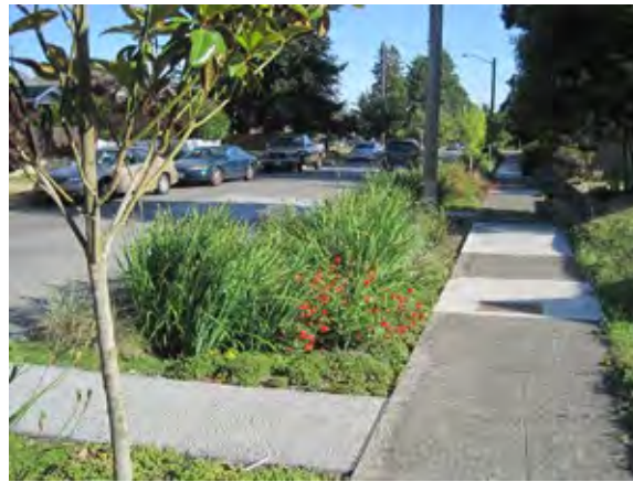
Figure 4-29. Permeable pavement walkways provide access to on-street parking in Seattle, WA.
