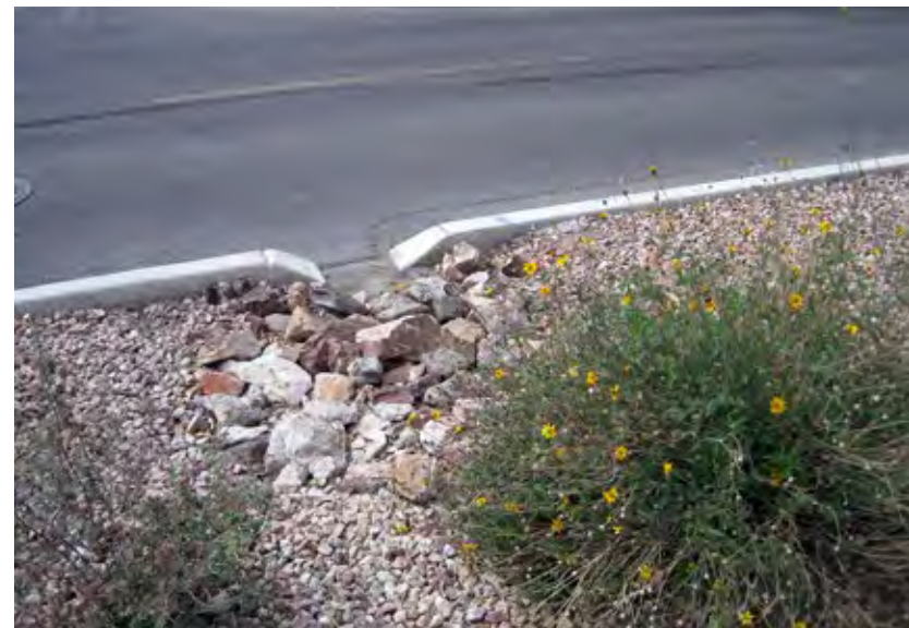
Figure 4-13. A sediment forebay slows the concentrated flow to allow sediment to drop out of suspension in Tucson, AZ.
