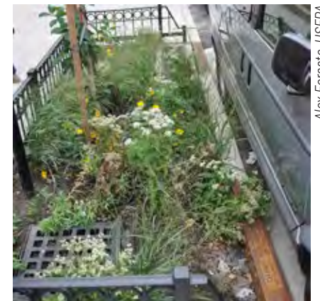
This stormwater planter does not provide space for passenger exit.
