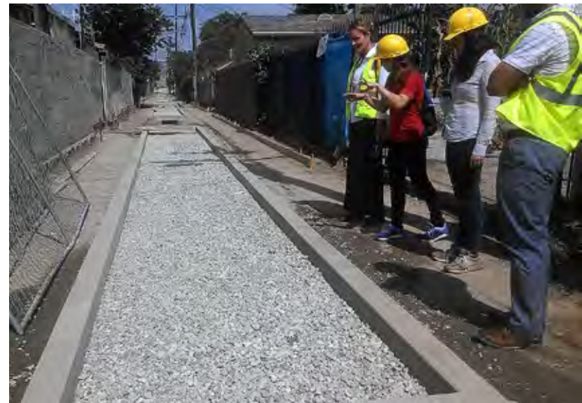
Permeable paving in an alley in the Avalon neighborhood in Los Angeles, CA.
