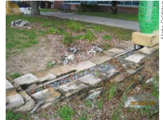
Figure 4-16. A piled stone weir/gravel filter combination slows the water flowing through this bioretention feature in Gainesville, FL.
