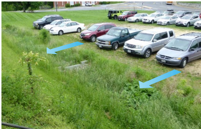
Figure 4-11. A curbless grassed and gravel parking lot allows sheetflow stormwater runoff to enter a vegetated swale in Staunton, VA.
