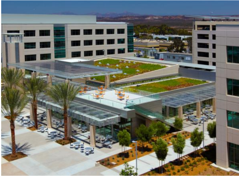
Location: County of San Diego Operations Center, San Diego, California
