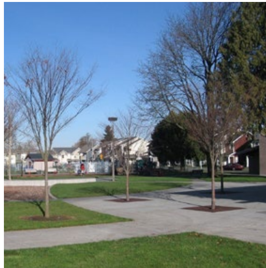
Tree pits treat stormwater runoff at a park in Portland, OR.
