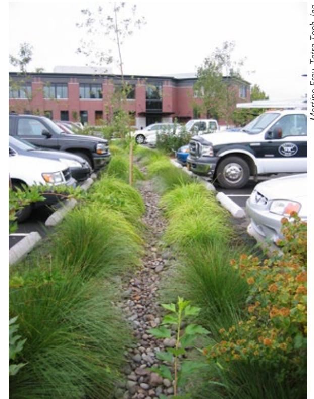
Parking lot bioswale conveys runoff from a parking lot in Wilsonville, OR.
