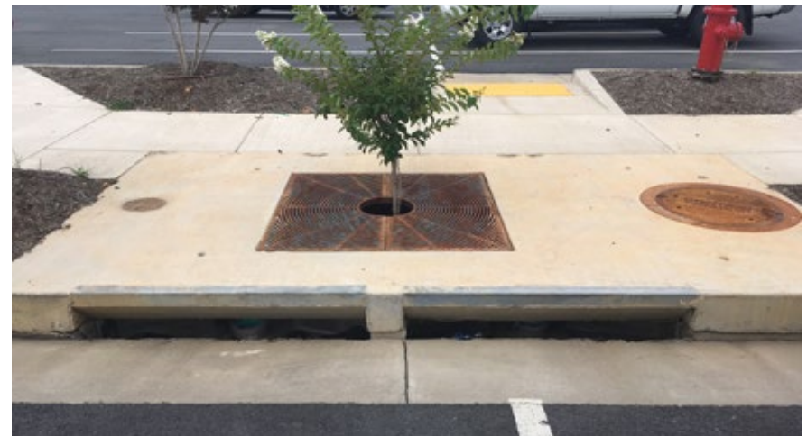
Stormwater catch basin tree pit, Charlottesville, VA.
