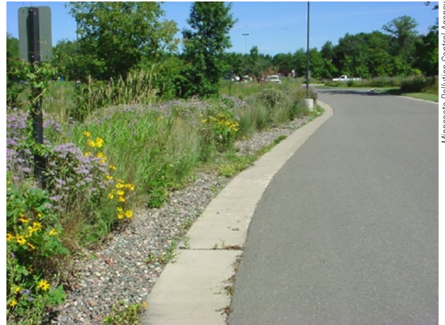
Infiltration trench adjacent to a Minnesota roadway.
