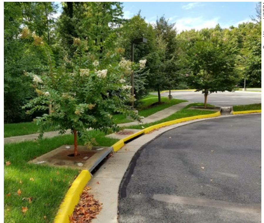
Stormwater tree pits in a parking lot, Reston, VA.
