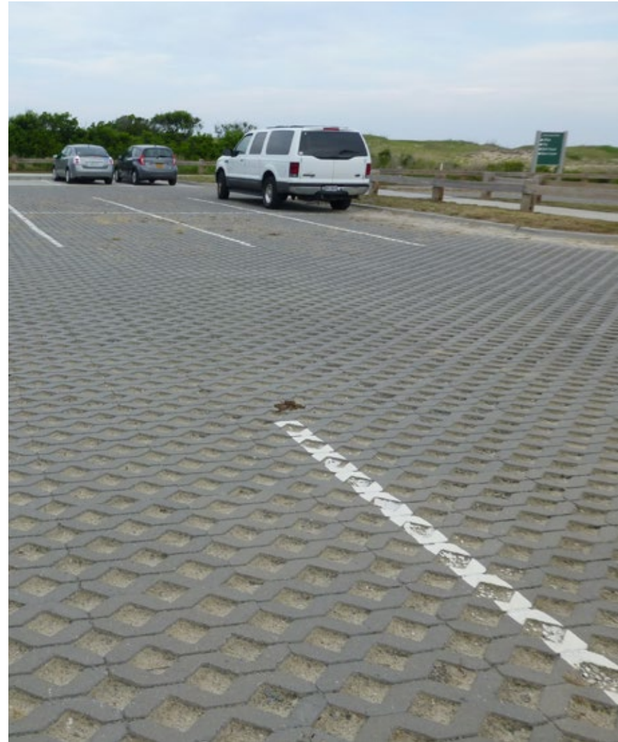
Sand-filled permeable pavers allow rainfall to infiltrate instead of generating erosive runoff in a sensitive coastal area in Virginia Beach, VA.
