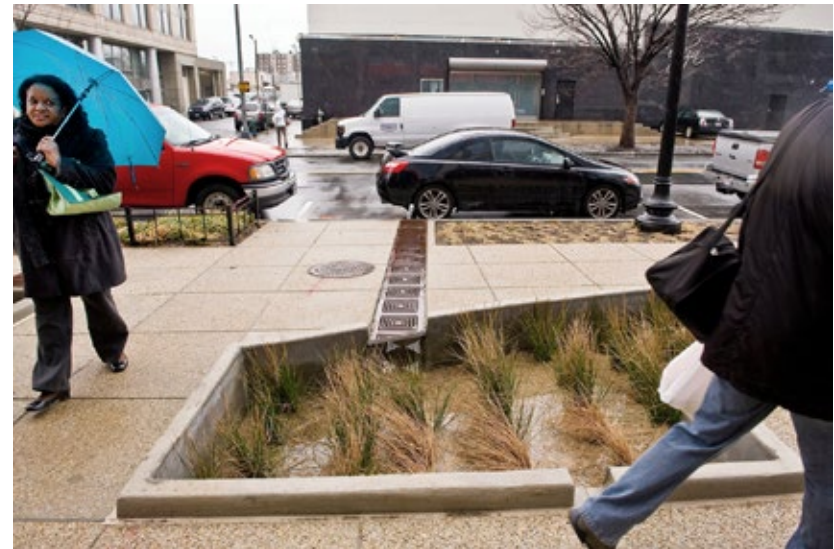
Trench drain conveys street runoff into bioretention cells in Washington, DC.
