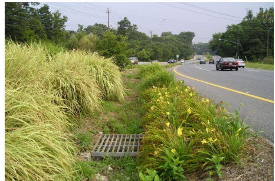
Road runoff will be treated by this bioswale in the median of Adelphi Road, an arterial road in Maryland.
