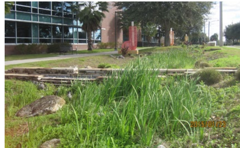
Bioretention area outside the recreation center at the University of Florida, Gainesville, FL.
