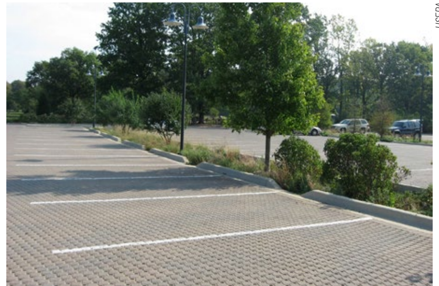
Figure 4-24. Vegetated swales were installed adjacent to a permeable parking lot in Chicago, IL, to provide overflow control and back-up infiltration as needed.
