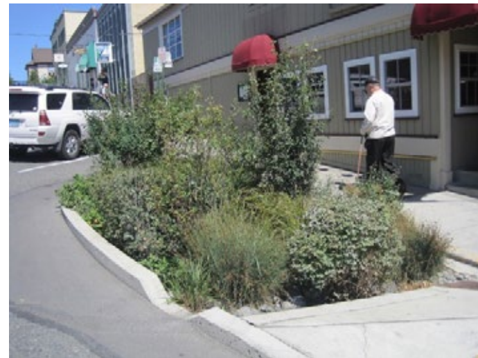
Figure 1-3. Soil and plants absorb and filter out excess nutrients and other pollutants from runoff, while microbes in the soil help break down the chemical compounds.
