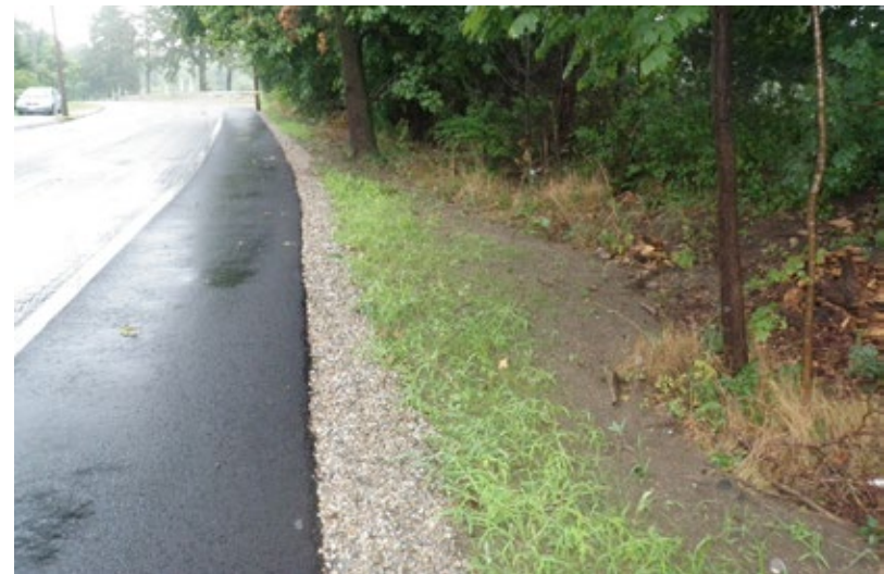
Infiltration trench (gravel) adjacent to a roadway.
