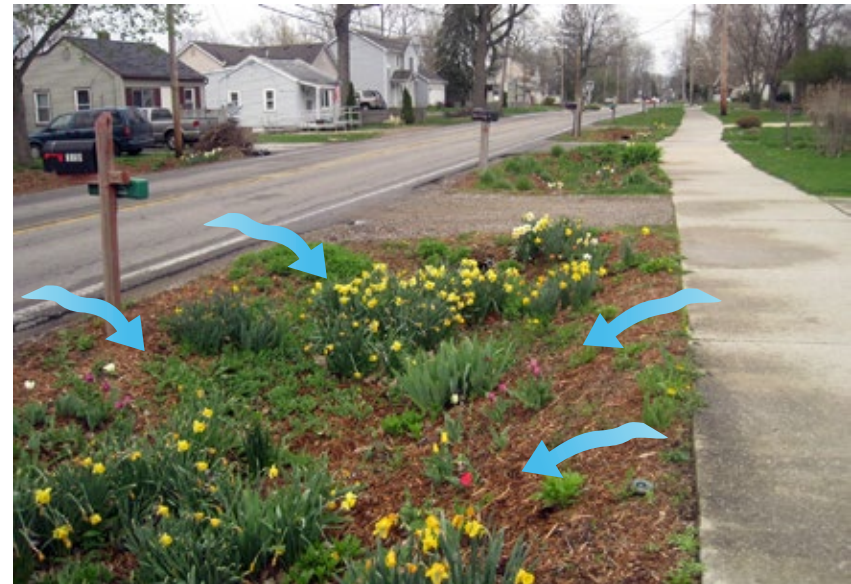
Figure 4-10. A curbless street allows sheetflow stormwater runoff to enter the vegetated swale in Lansing, MI.
