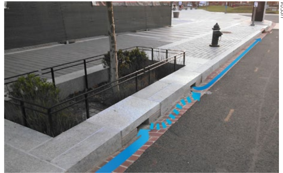
Figure 4-23. In this tree pit bypass system in Washington, DC, curb cuts allow stormwater to enter until the practice is filled, at which point additional flow bypasses the system and continues down the street to the storm drain.
