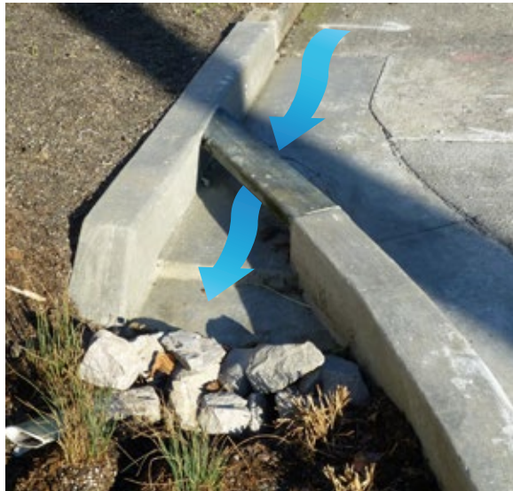
Figure 4-4. Metal extension inlet structure provides a wide opening for stormwater flow to enter the stormwater feature.
