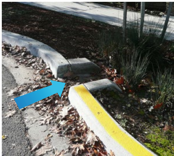
Figure 4-7. A curb cut with wings retains the side slope grade and directs street runoff into a bioretention feature in Portland, OR.
