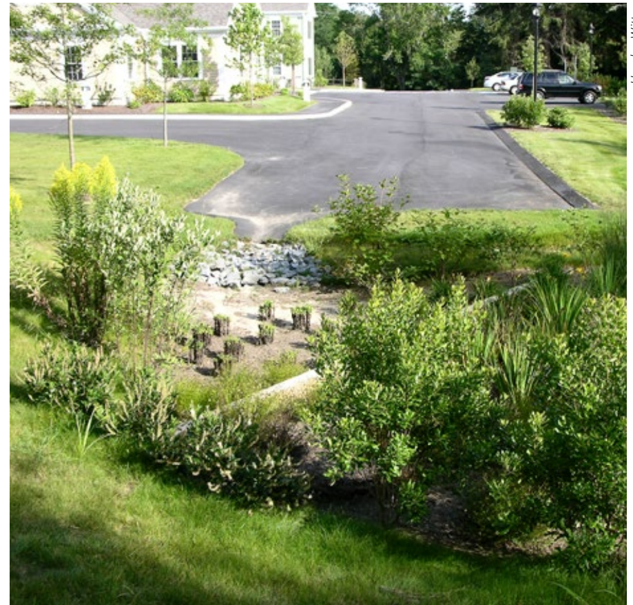
A sediment forebay provides pretreatment for a bioretention cell in Barnstable, MA.
