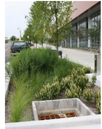
Figure 4-20. Concrete band structure constructed around the outflow allows ponding in Nashville, TN.
