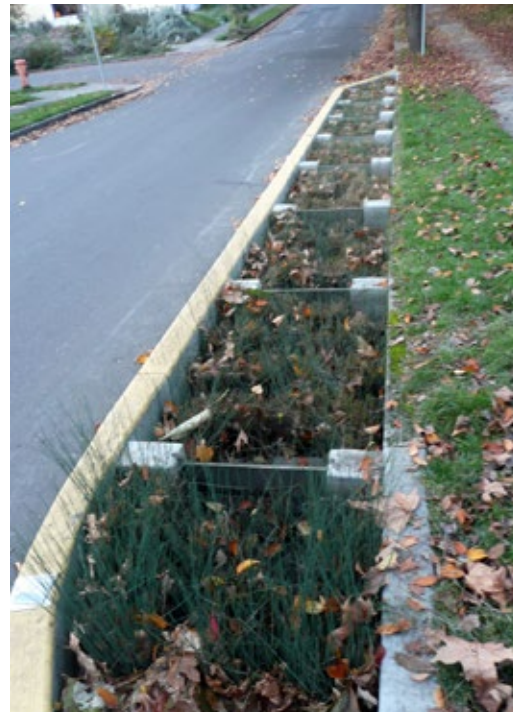
Figure 4-17. Concrete check dams slow flow in a stormwater curb extension with a 4.2% slope in Portland, OR.
