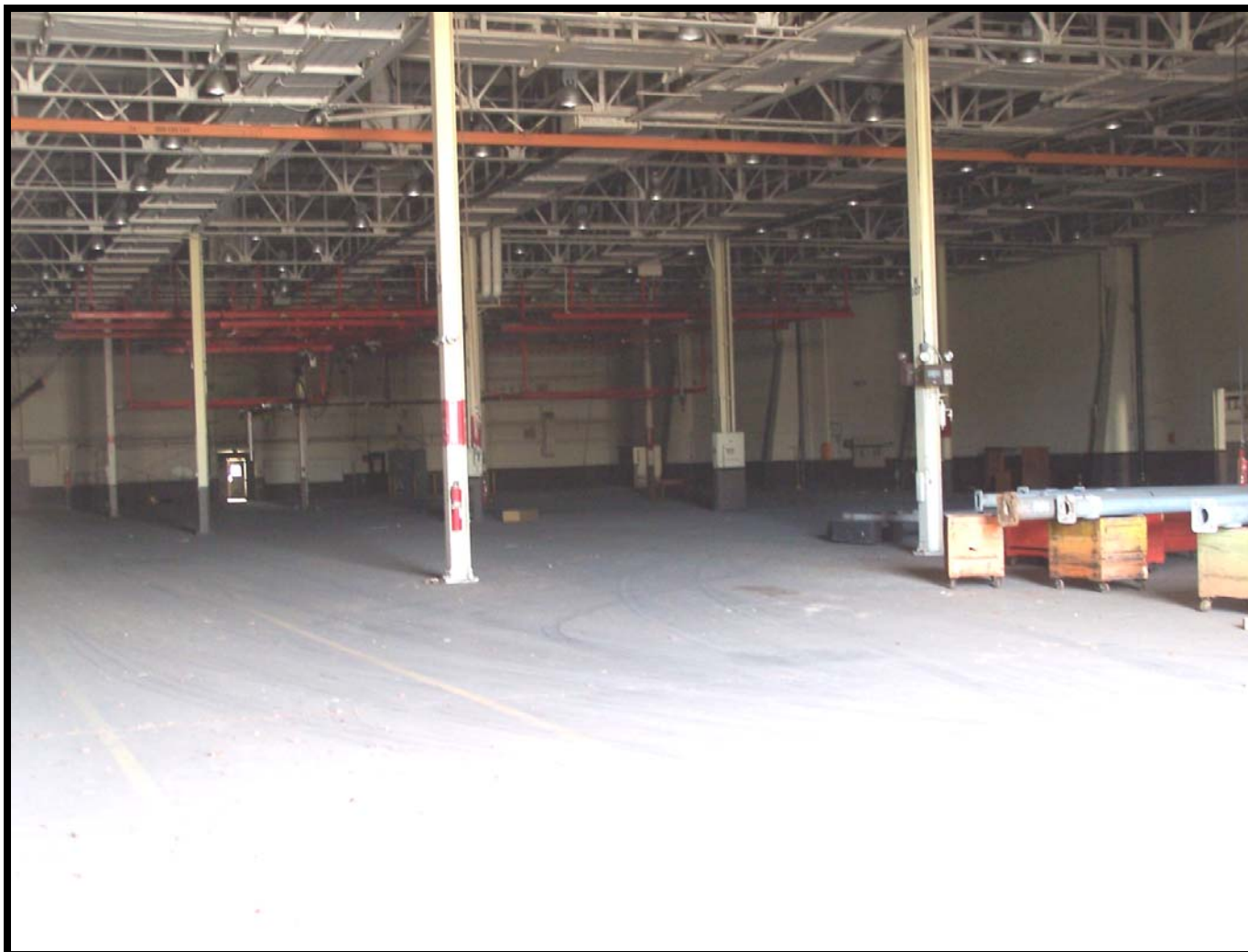
Figure 23: Large open manufacturing plant interior in the north half of Building 146.
