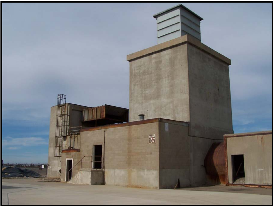
Figure 60: Building 157, a non-contributing element.
