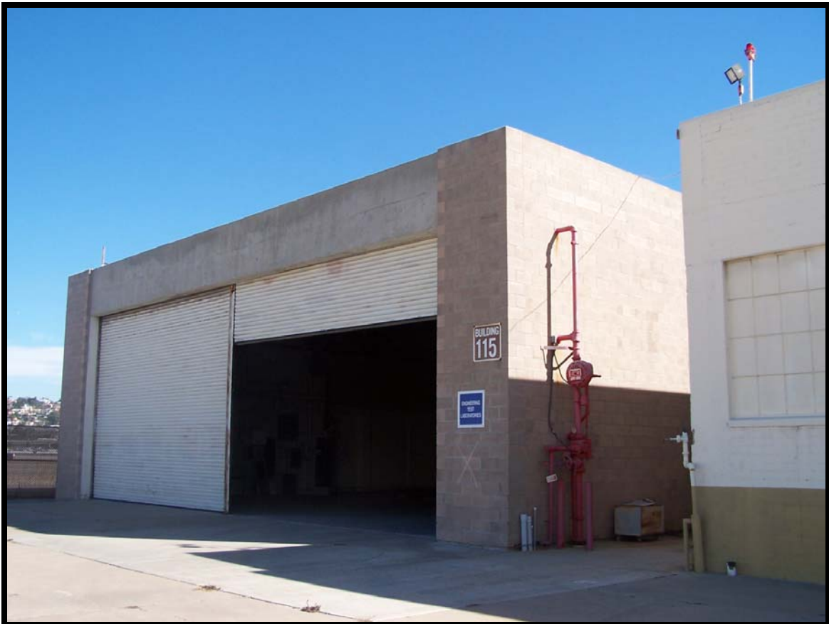
Figure 46: Building 115, a non-contributing element.
