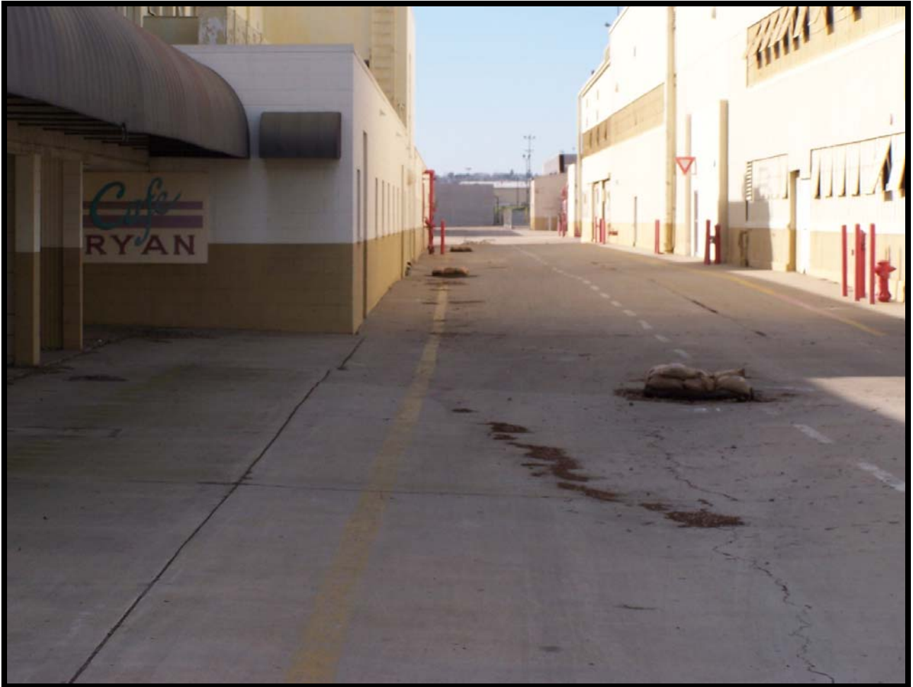
Figure 40: This narrow paved passage between Buildings 102 and 146 characterizes the setting in the eastern portion of the Ryan Aeronautical company complex.
