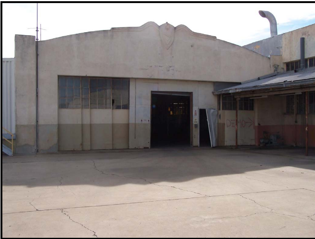
Figure 37: The front (north) side of the east wing addition of Building 180. This was the small hangar built at the Pacific Highway facility around 1935. Note the shield at the crest of the roofline.
