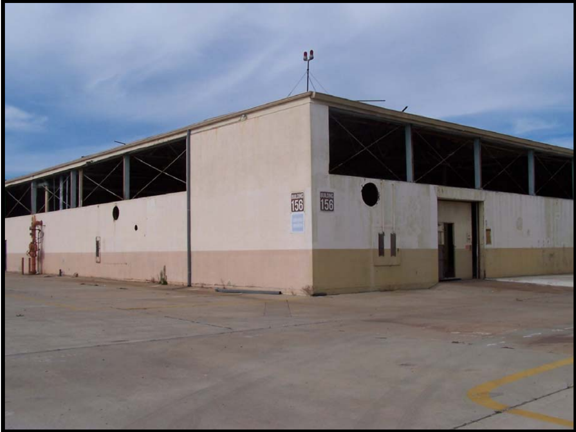
Figure 26: The southwest corner of Building 156. The rows of steel framed windows have been removed.
