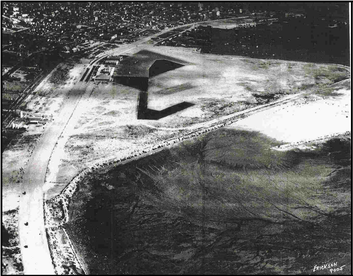
Figure 21: Newly paved surfaces can be seen in this circa 1933- 1934 aerial photograph of Lindbergh Field. Pacific Highway on the left of the airport is graded but not paved (San Diego Aerospace Museum).
