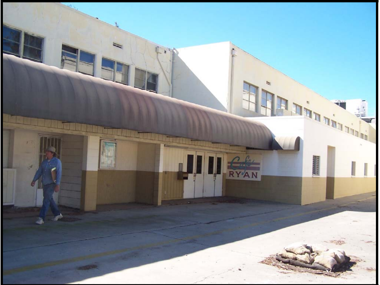
Figure 6: The back (north) side of Building 102, showing the variety of window and doorway placements.
