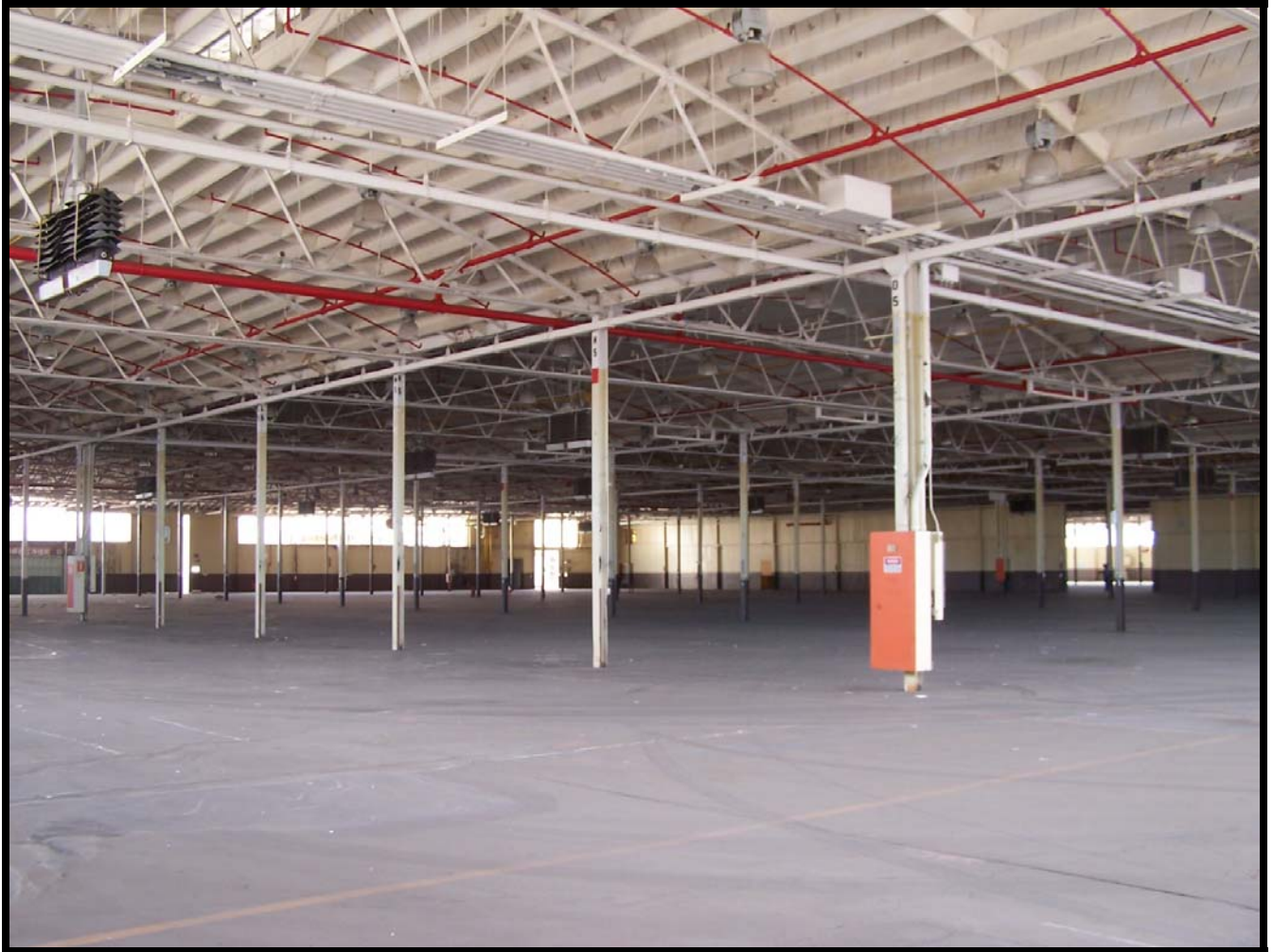
Figure 25: The large open interior of Building 152. Note the steel arched roof trusses supported by "I" beam posts.
