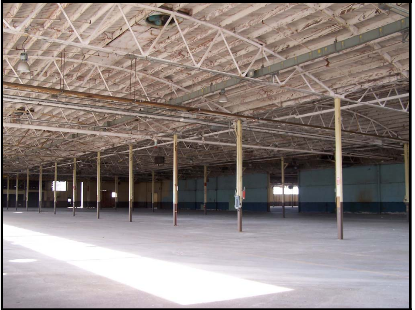
Figure 27: The large open interior of Building 156 showing the arched steel roof trusses supported by steel "I" beam posts. The opening near the far center of the photo leads to Building 152.
