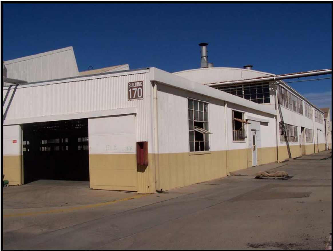
Figure 68: Building 170, a non-contributing element.
