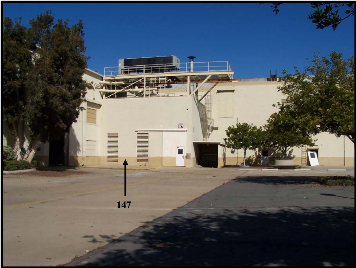
Figure 1: Building 147, a non-contributing element.
