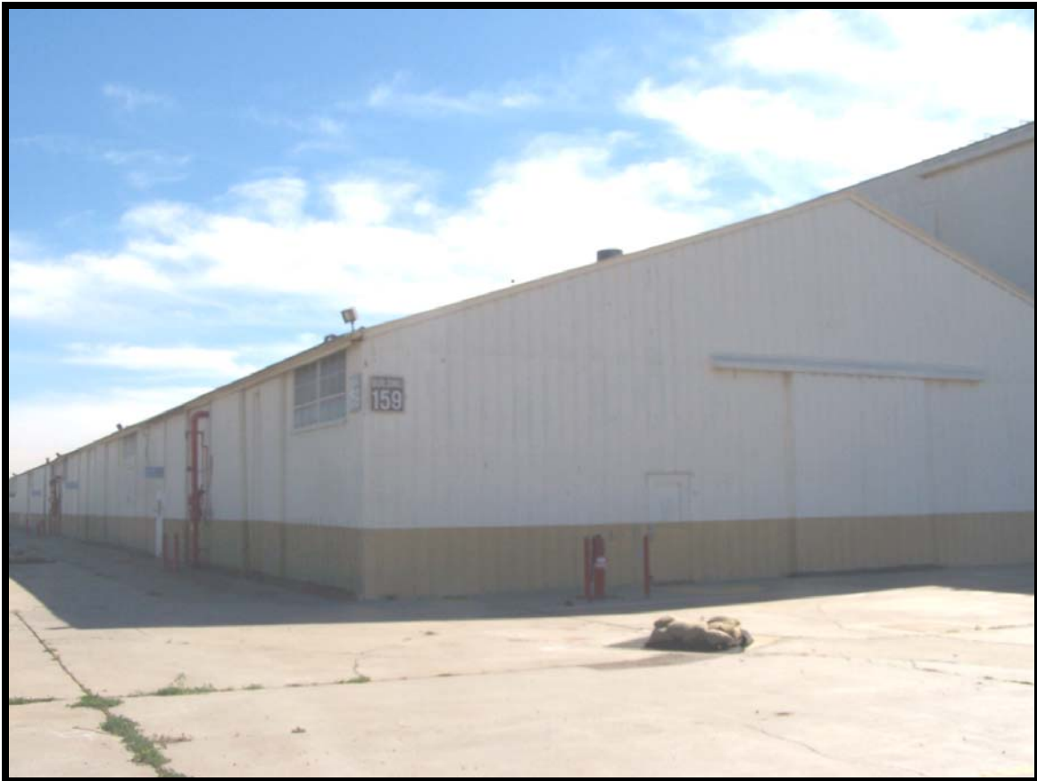
Figure 62: Building 159, a non-contributing element.
