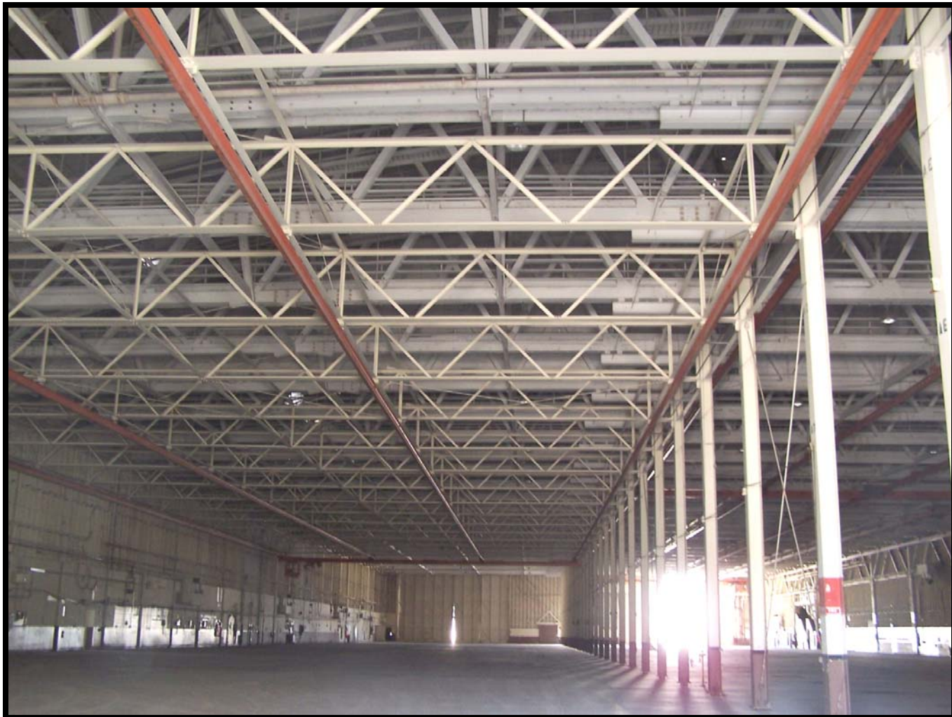
Figure 20: The large open interior of Building 140 from the east end looking west.
