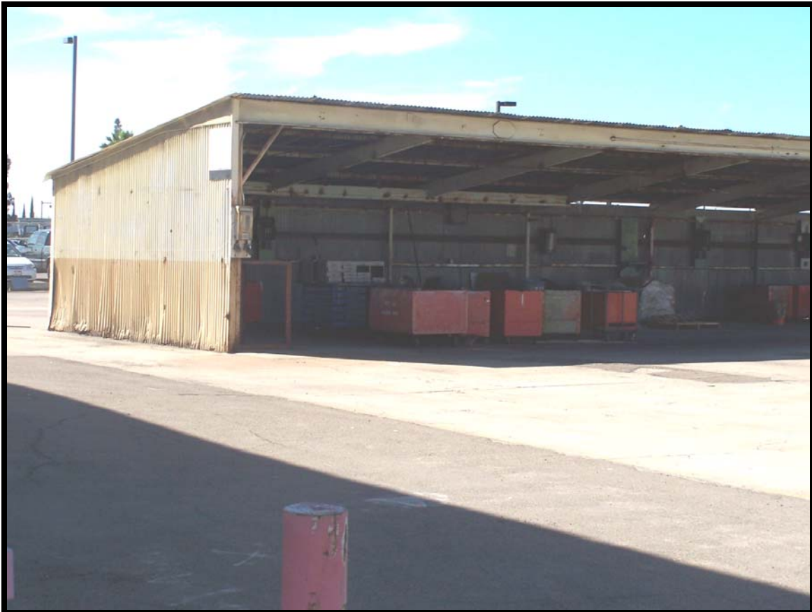
Figure 74: Building 242, a non-contributing element.
