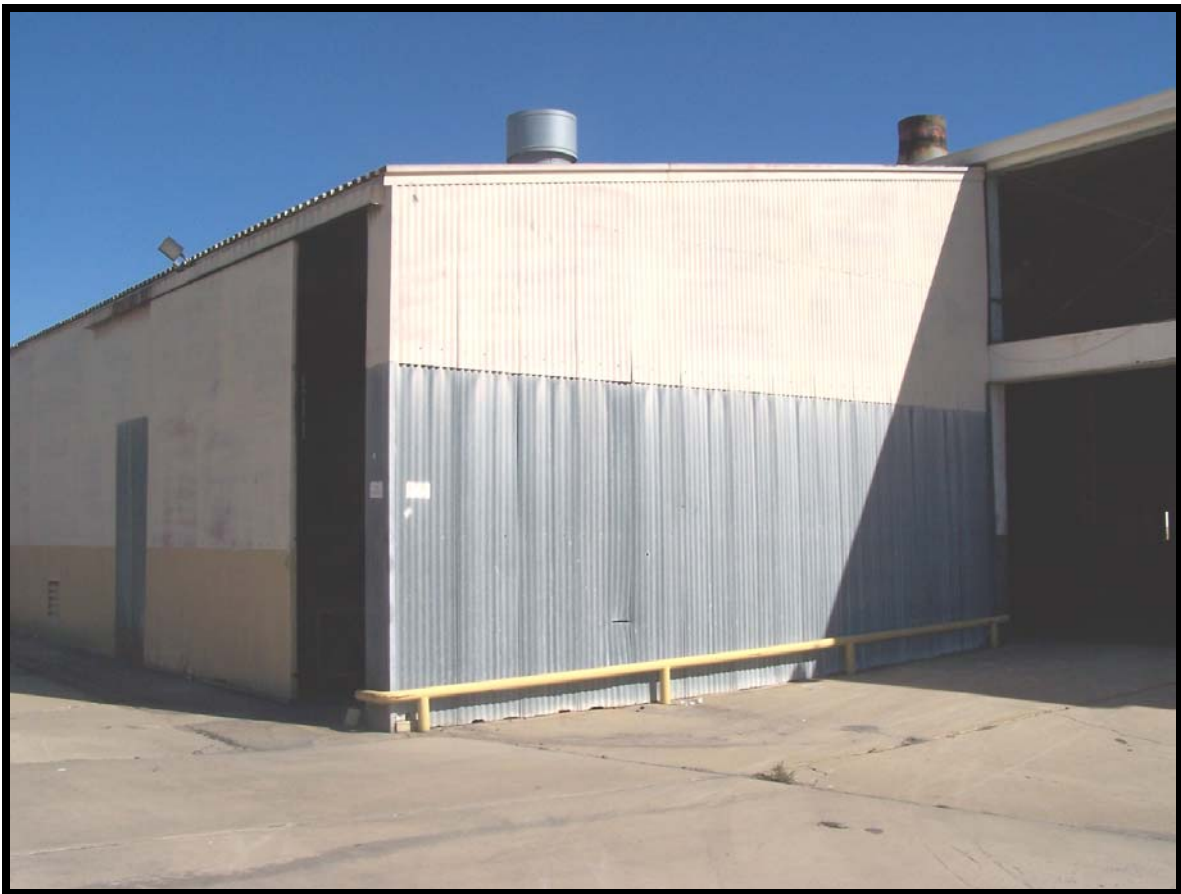
Figure 75: Building 513, a non-contributing element.
