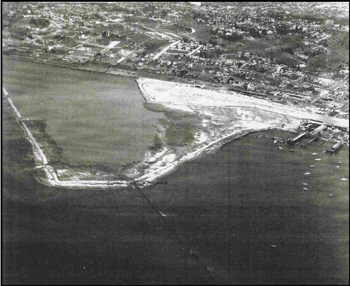
Figure 9: This March 1929 photograph shows dredging operations continuing to reclaim tidelands on the west side of the airport (San Diego Aerospace Museum).
