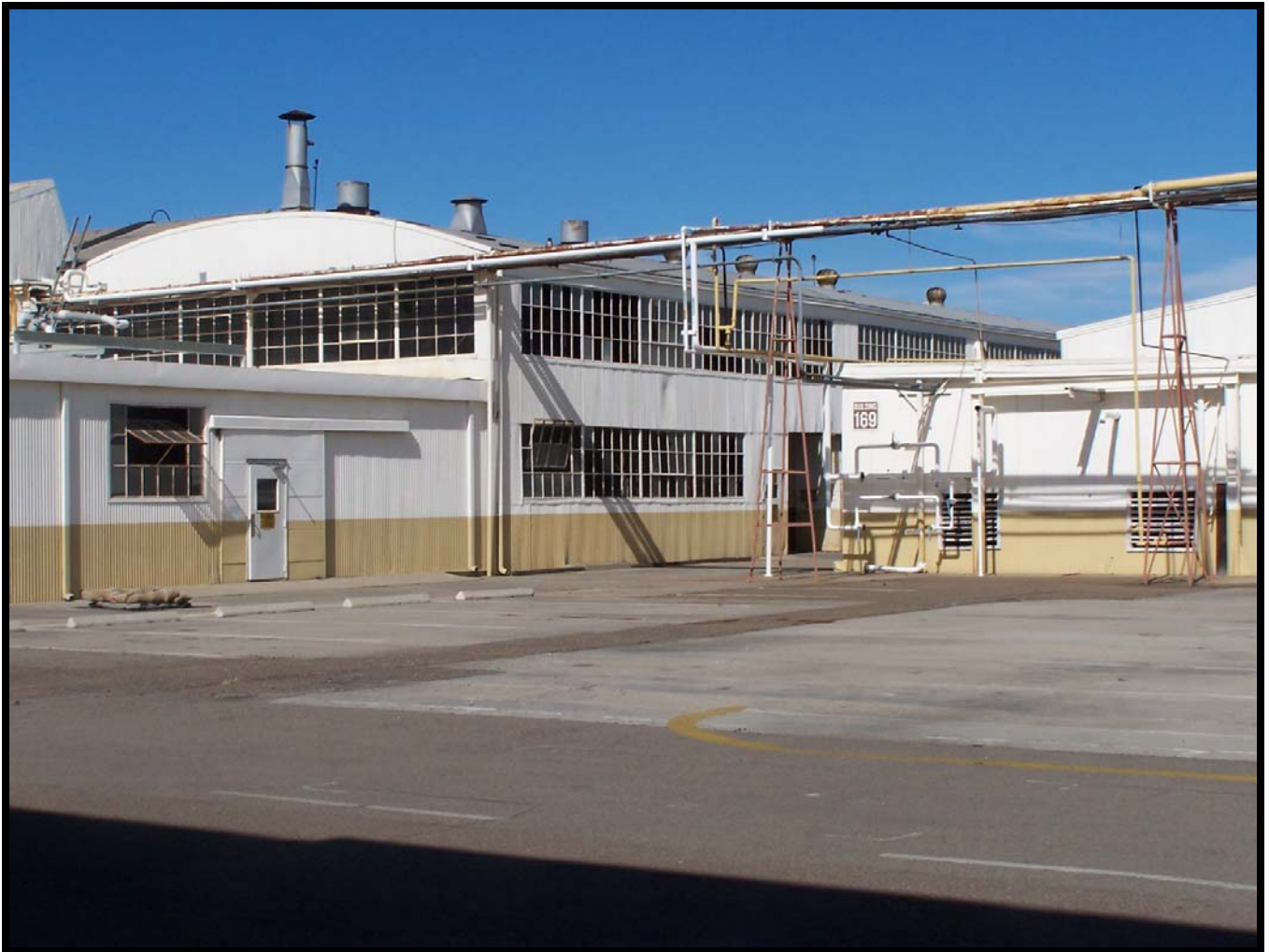
Figure 9: The southeast corner of Buildings 110/112 (122), showing the continuous rows of windows and arched roofline that is typical of aircraft factory buildings from the World War II era. The flat roofed Building 170 in the foreground and Building 169 to the left are not contributing elements to the district.
