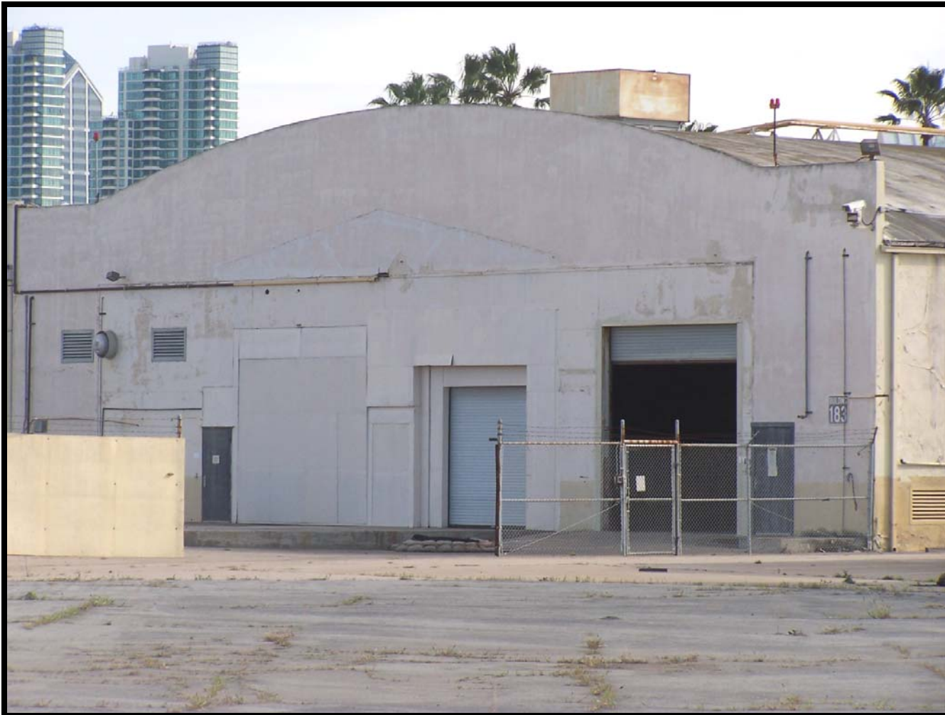
Figure 39: The front (north) side of Building 183.
