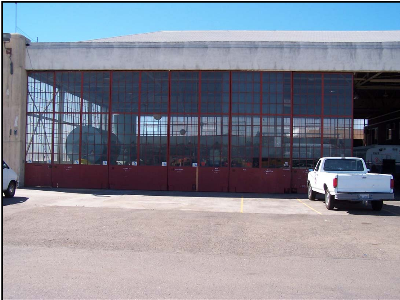
Current (2005) view of the front (north) side of the 1931 United Airlines Hangar, showing the sliding glass curtain wall hangar doors.
