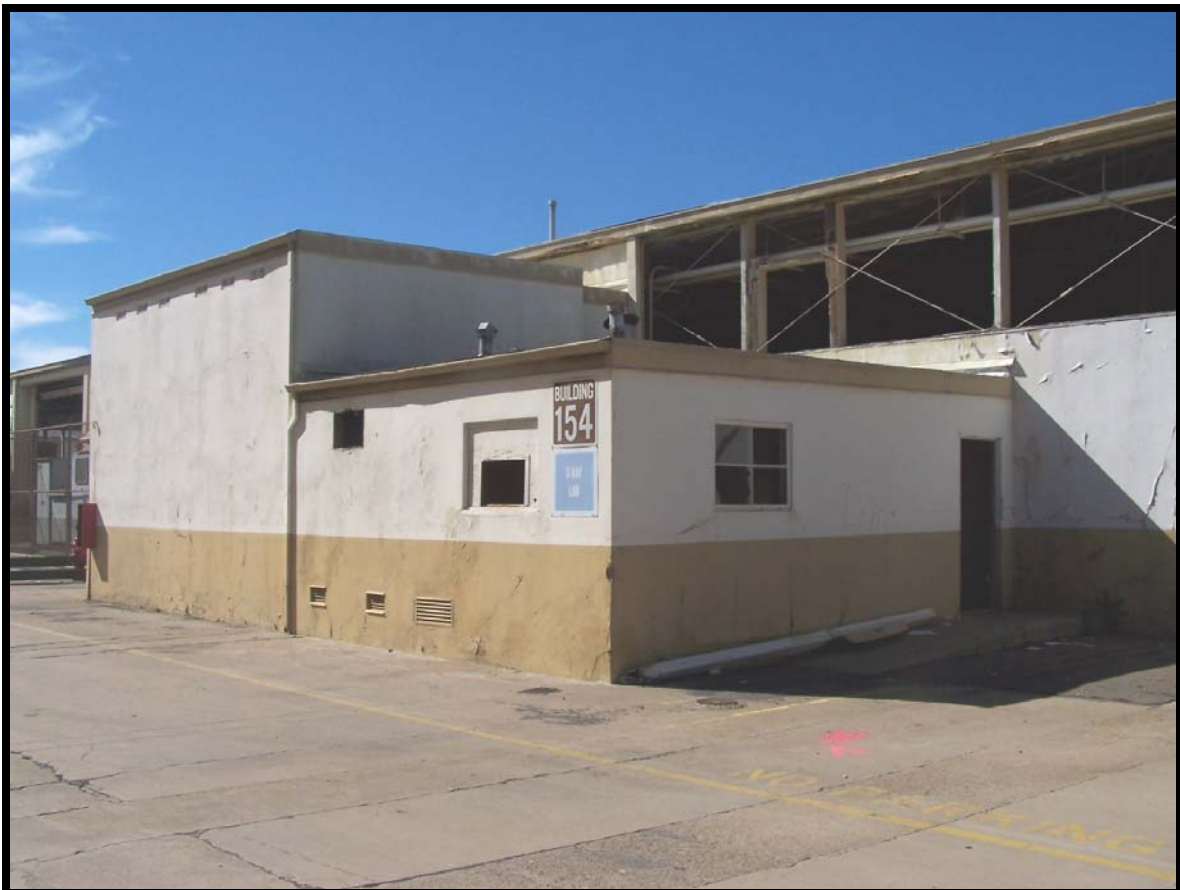
Figure 59: Building 154, a non-contributing element.
