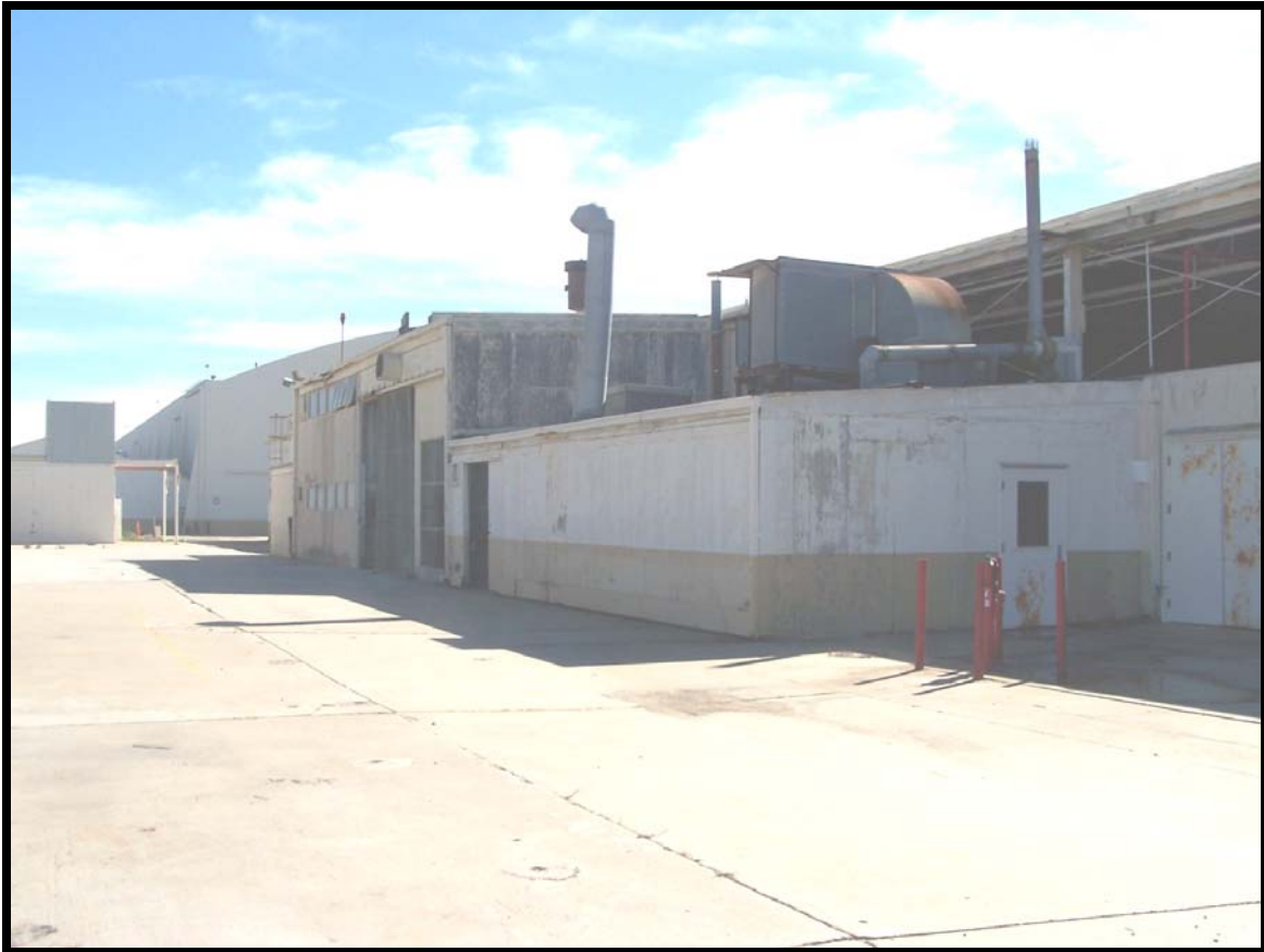
Figure 71: Both of these units constitute Building 230, a non-contributing element.
