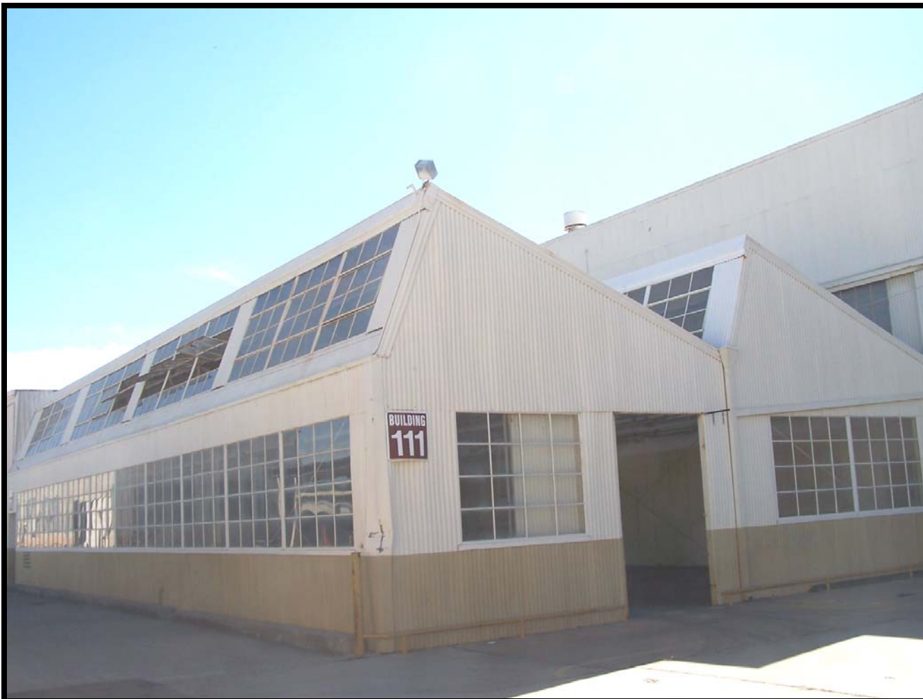
Figure 10: The northeast corner of Building 111, showing the character defining saw tooth roof profile and continuous rows of multi-paned windows.
