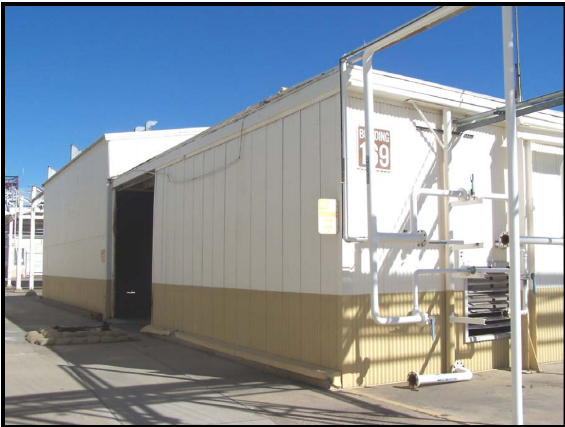
Figure 67: Building 169, a non-contributing element.
