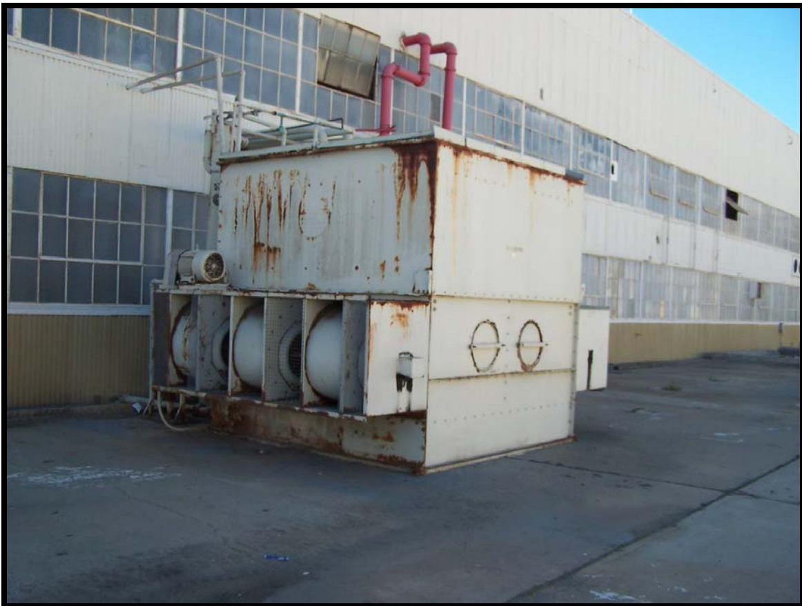
Figure 73: Facility 240, a non-contributing element.
