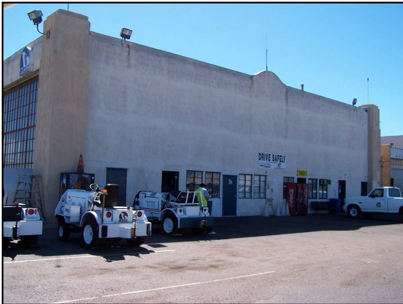
Current (2005) view of the west façade of the 1931 United Airlines Hangar and Terminal, looking southeast.
