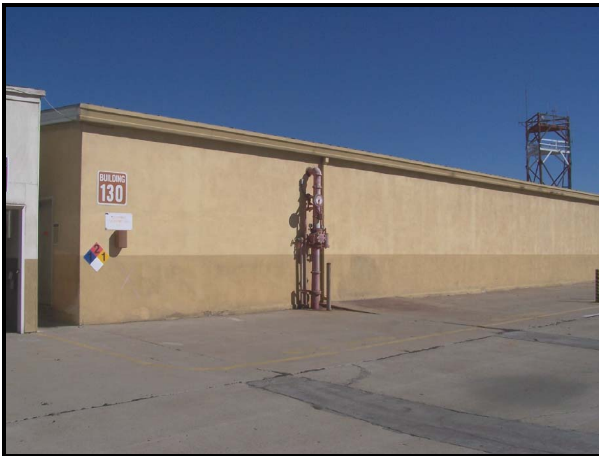
Figure 53: Building 130, a non-contributing element.
