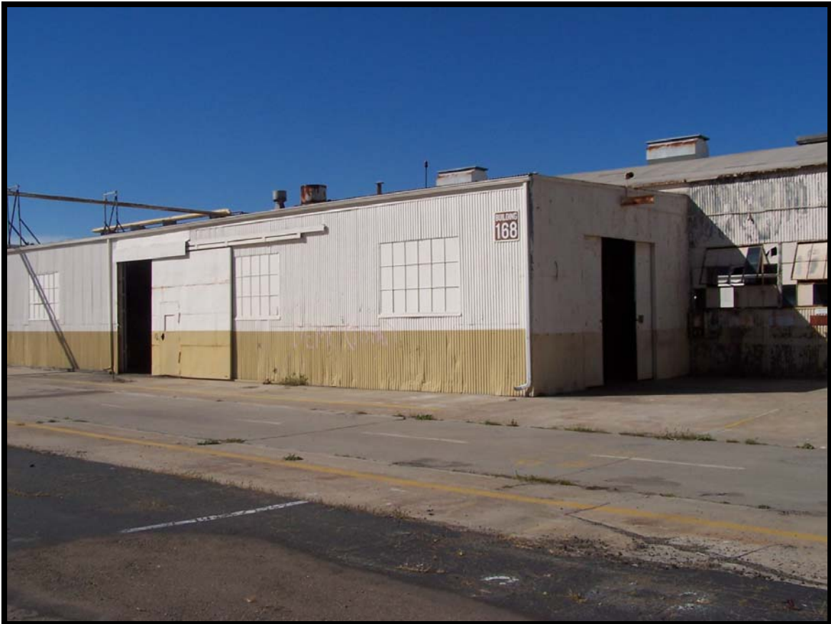
Figure 66: Building 168, a non-contributing element.
