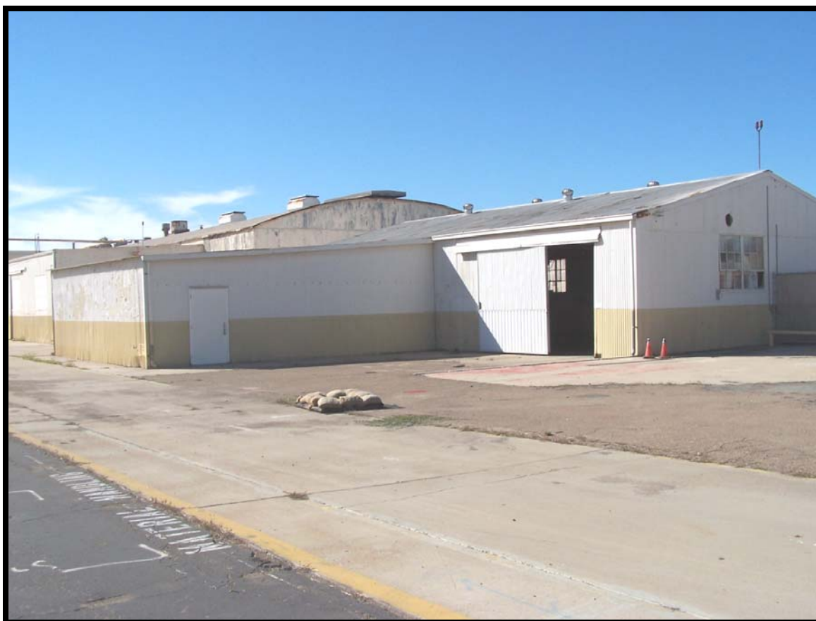
Figure 63: Building 161, a non-contributing element.
