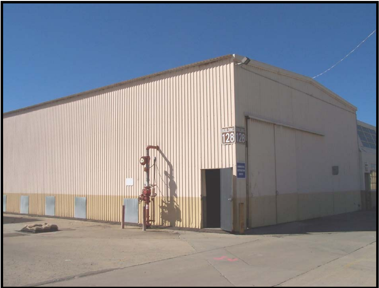
Figure 51: Building 128, a non-contributing element.
