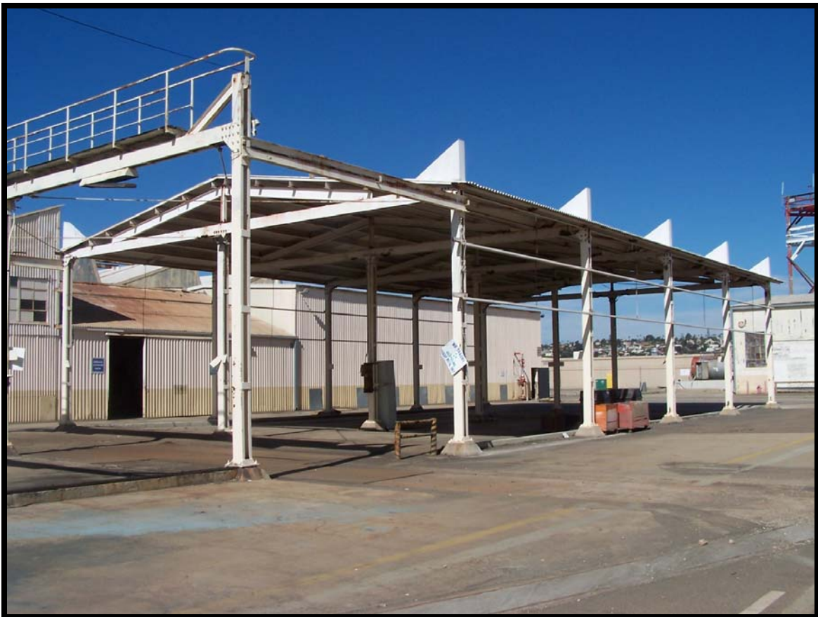
Figure 65: Building 167, a non-contributing element.
