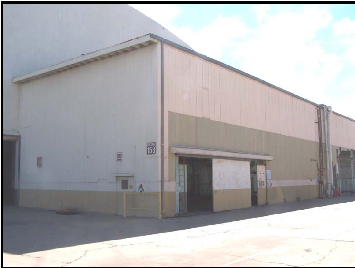
Figure 61: Building 158, a non-contributing element.
