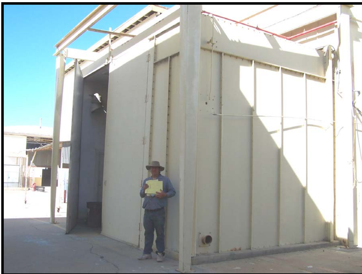
Figure 58: Building 153, a non-contributing element.
