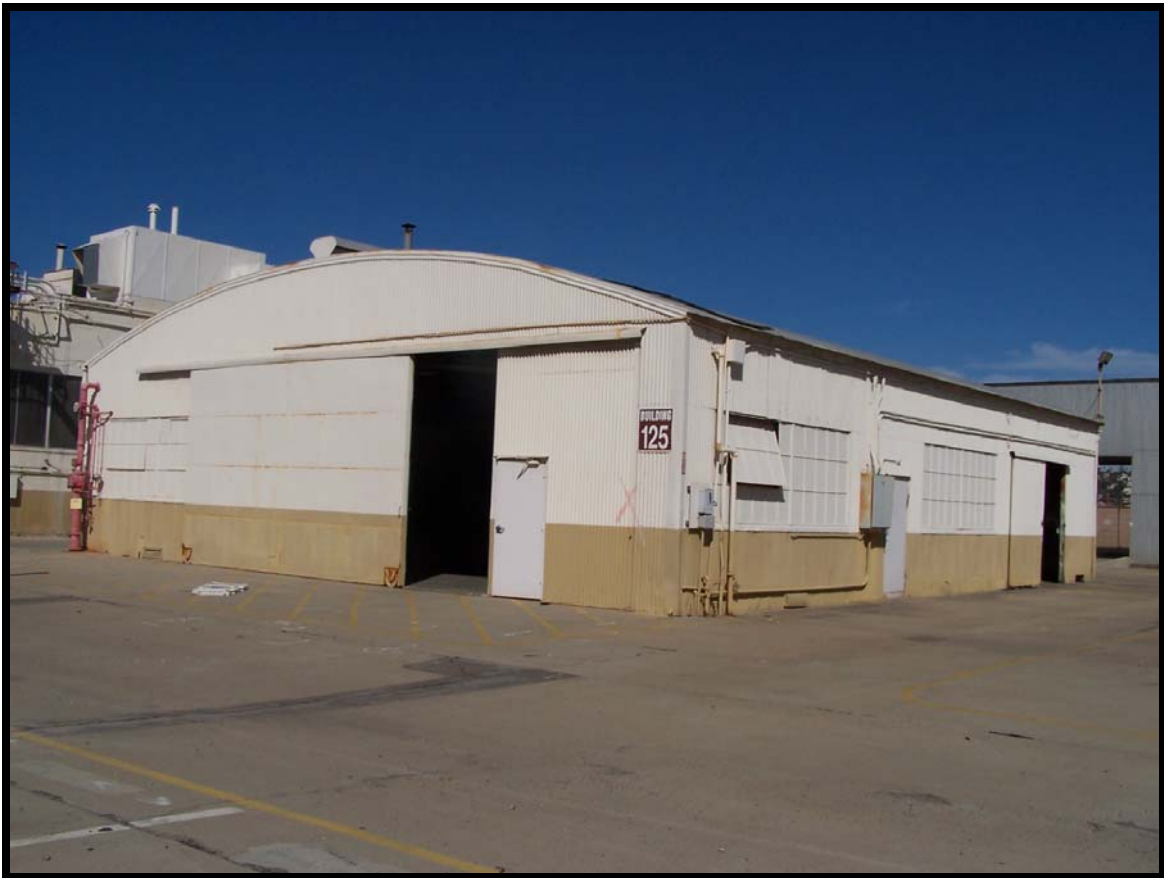
Figure 48: Building 125, a non-contributing element.
