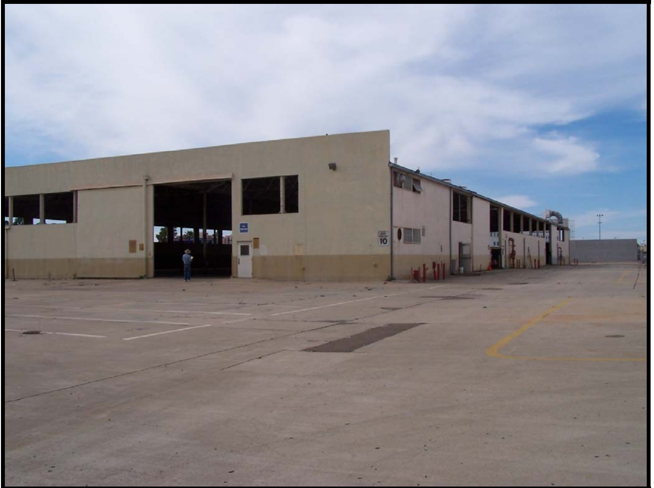
Figure 18: The northeast corner of building 131. Note the large hanging door on the east façade. The rows of steel framed windows have been removed.
