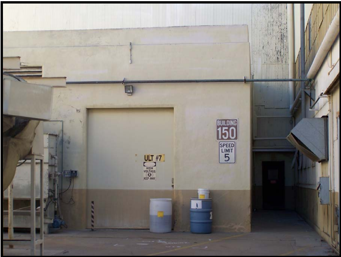
Figure 57: Building 150, a non-contributing element.
