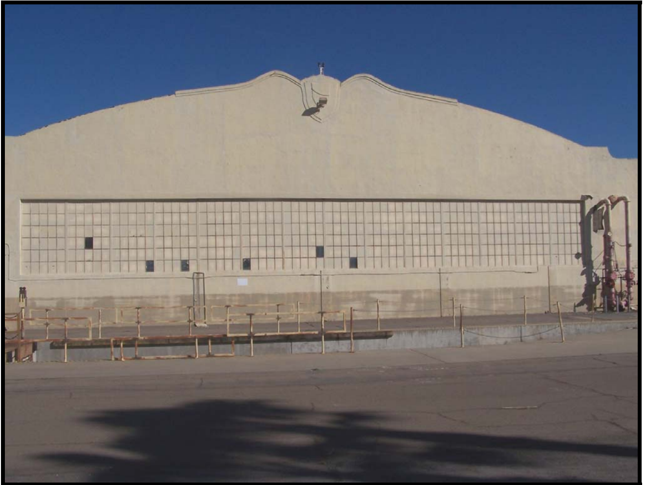
Figure 35: The south (back) side of Building 180. Note the continuous row of windows and the shield molded into the façade at the top of the roofline. This same motif also occurs on east wing addition to Building 180 and on Building 181 and can be seen in the historic photographs in Figures 29, 30, 32, and 33.
