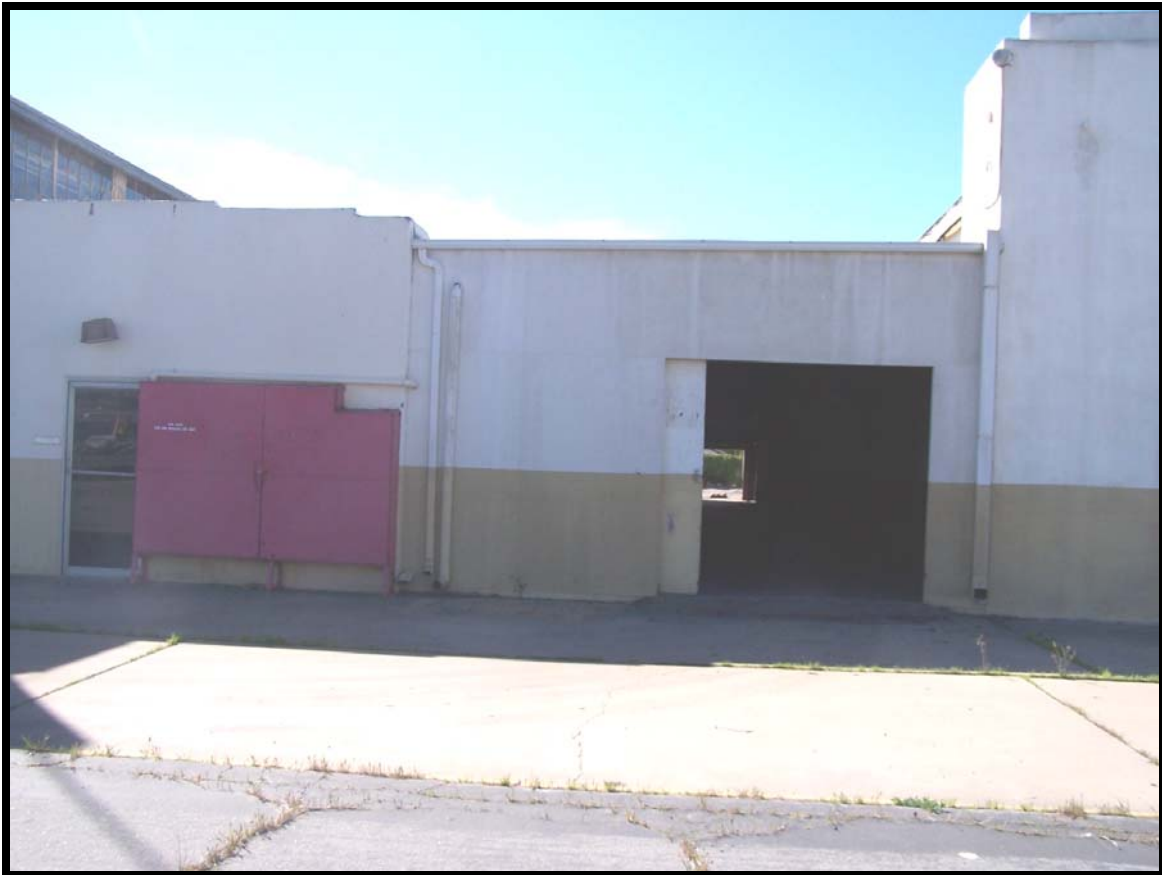
Figure 72: Building 236, located between buildings 180 and 181, is a non-contributing element.
