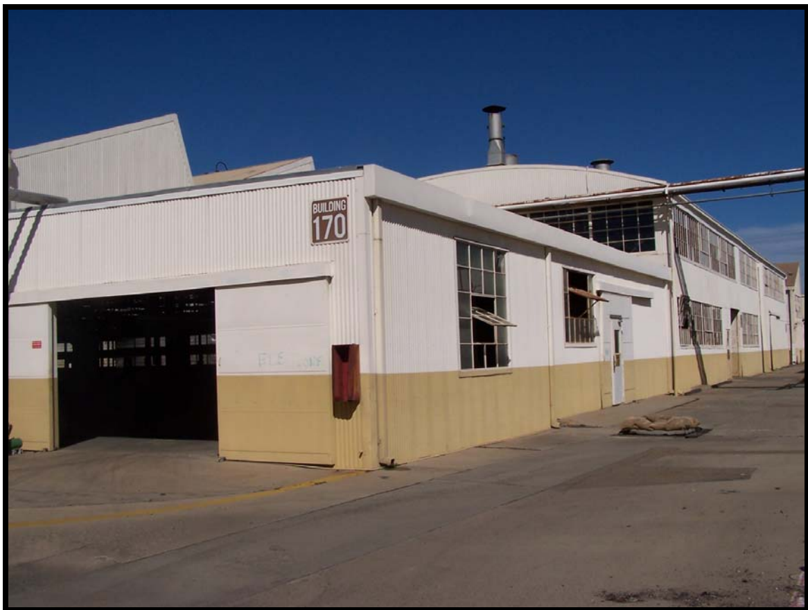
Figure 68: Building 170, a non-contributing element.
