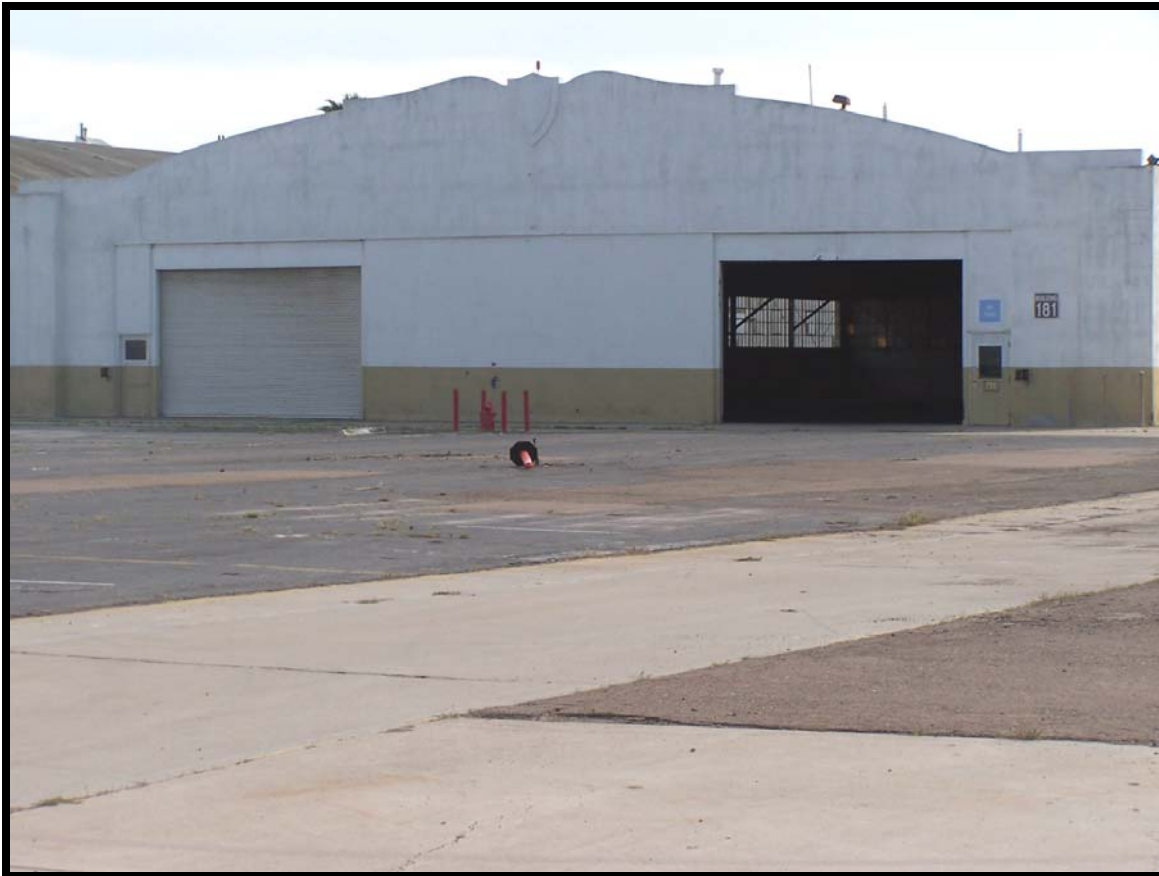
Figure 38: The front (north) side of Building 181. This was the third hangar built at Ryan's Pacific Highway facility sometime between 1936 and 1939. Note the shield at the crest of the roofline.
