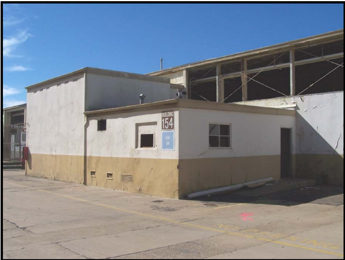
Figure 59: Building 154, a non-contributing element.
