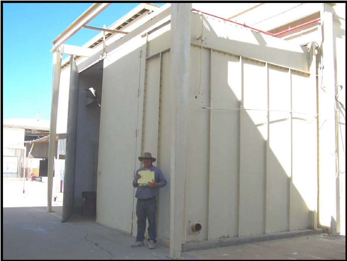
Figure 58: Building 153, a non-contributing element.
