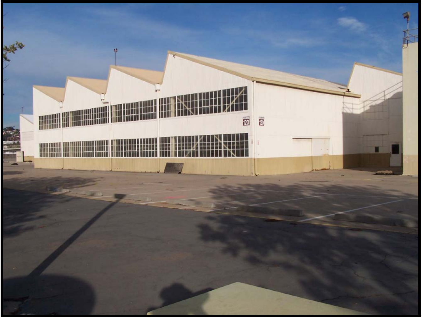
Figure 13: The southwest corner of Building 120, giving another view of the saw tooth profile roof and continuous rows of steel framed windows.
