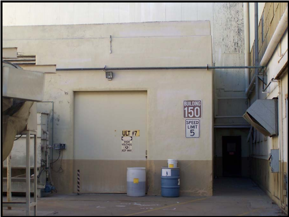
Figure 57: Building 150, a non-contributing element.
