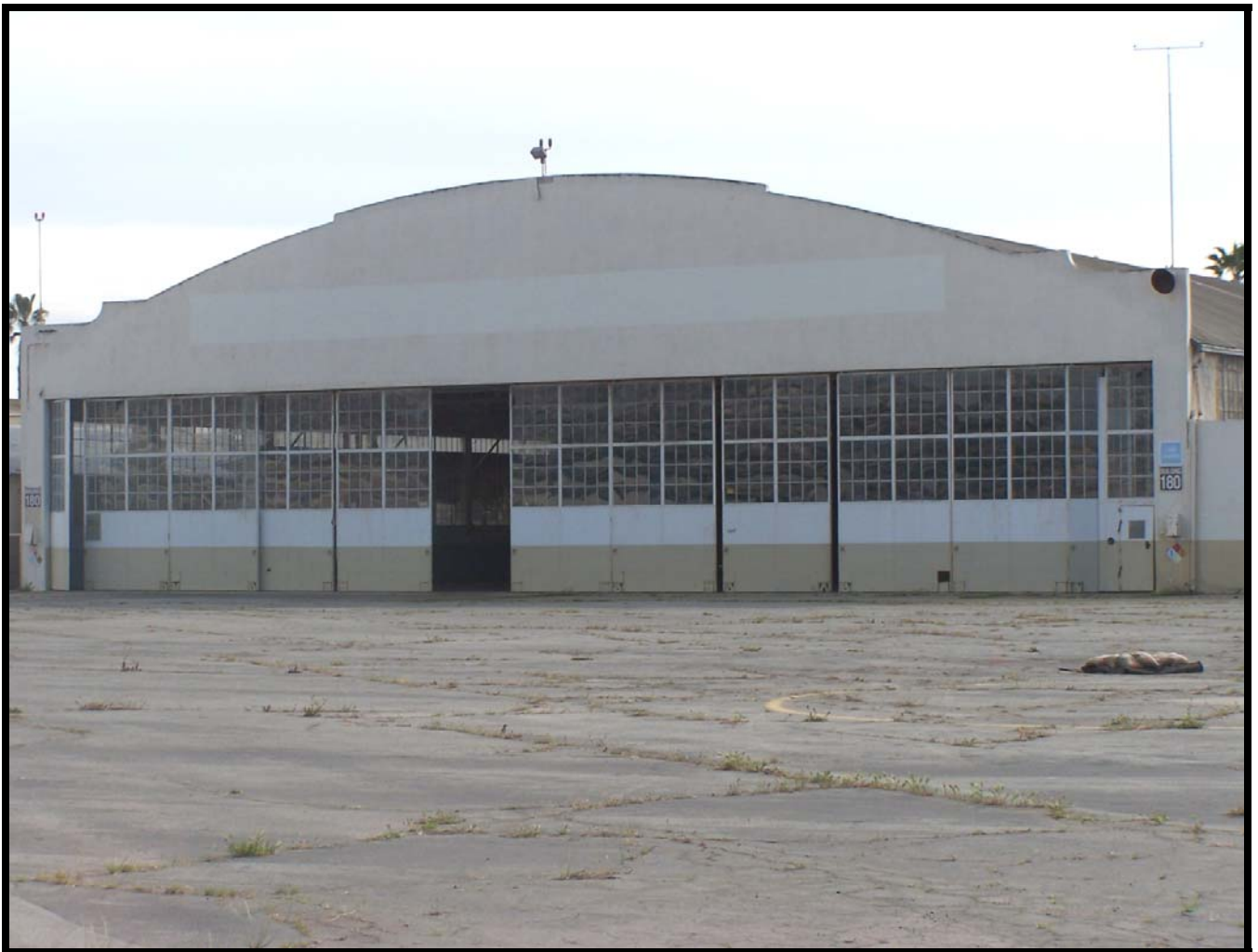
Figure 34: The front (north) façade of Building 180 showing the steel and glass hangar doors. This was the first hangar built at Ryan’s Pacific Highway Plant in 1932. These doors were originally on the south side of the building, where the shield crest is located (see Figures 29, 30, 32, 33, and 35). They were changed to this side when the building was moved to its present location on the early 1940s.
