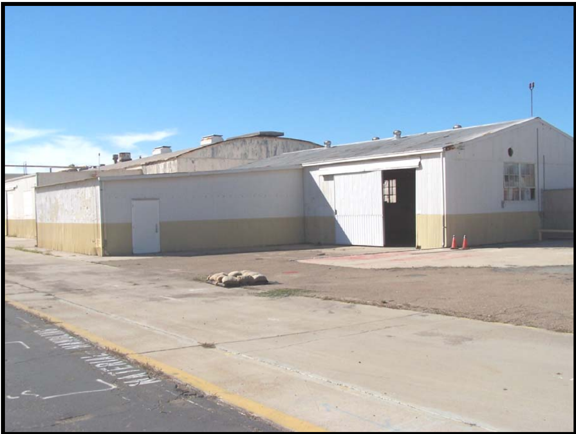
Figure 63: Building 161, a non-contributing element.
