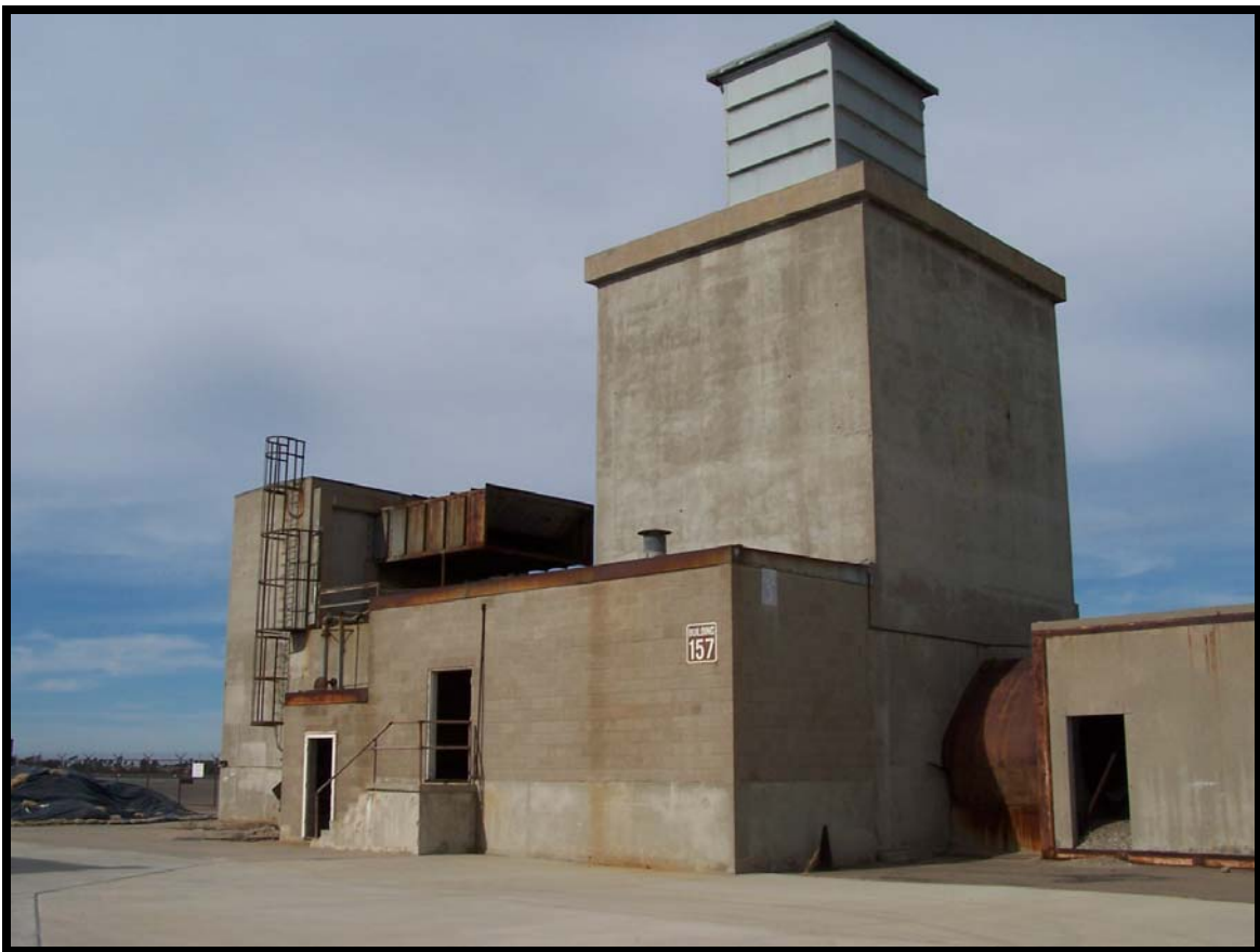
Figure 60: Building 157, a non-contributing element.
