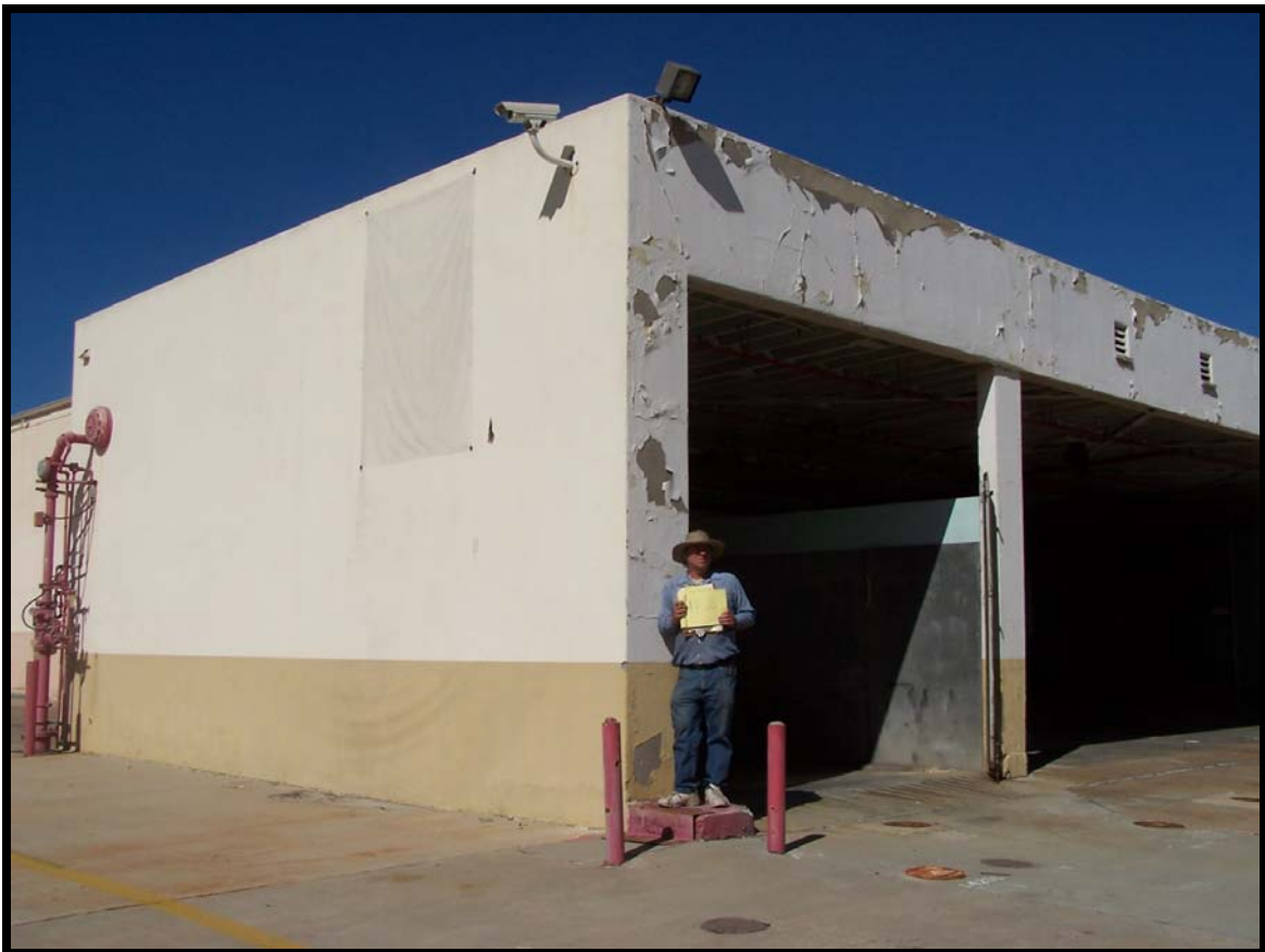
Figure 54: Building 142, a non-contributing element.
