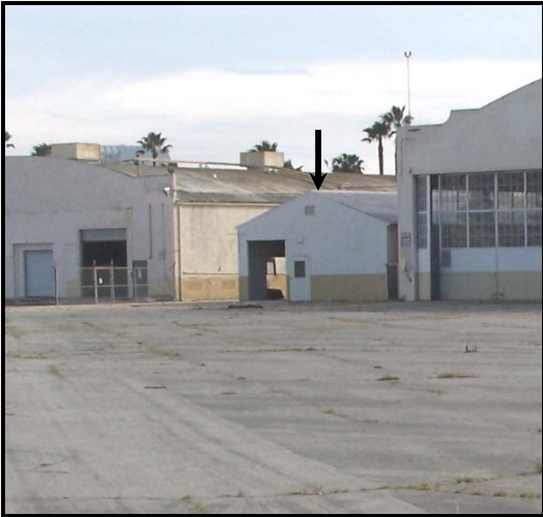
Figure 69: Building 182, a non-contributing element.
