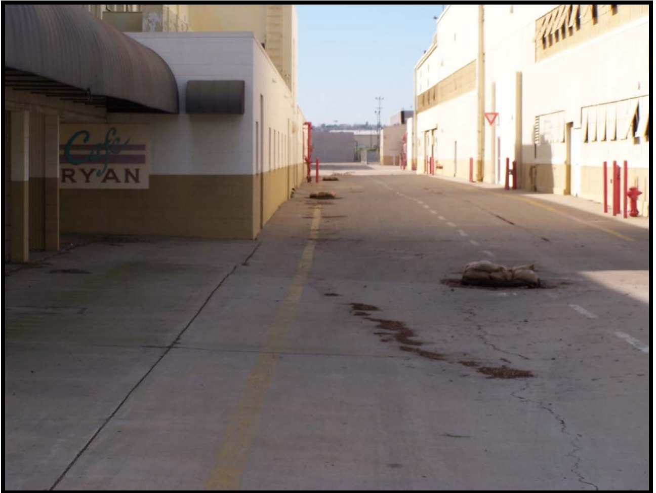
Figure 40: This narrow paved passage between Buildings 102 and 146 characterizes the setting in the eastern portion of the Ryan Aeronautical company complex.
