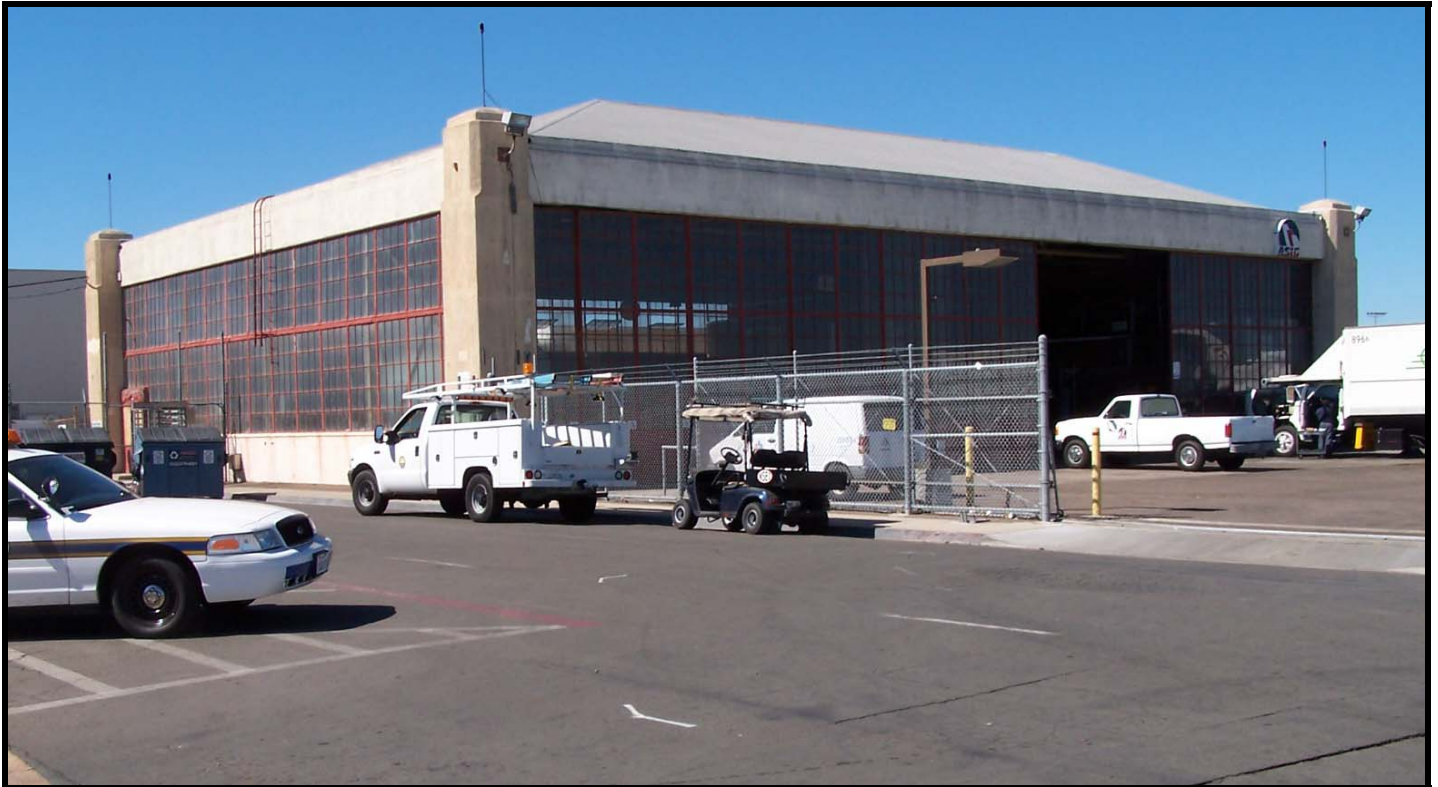
View of the east and north (front) sides of the 1931 United Airlines Hangar, looking southwest. Note how little the stuccoed exterior, glass curtain walls, corner pillars, and roofline have changed from their appearance in the 1931 photographs of the building that precede these photos.
