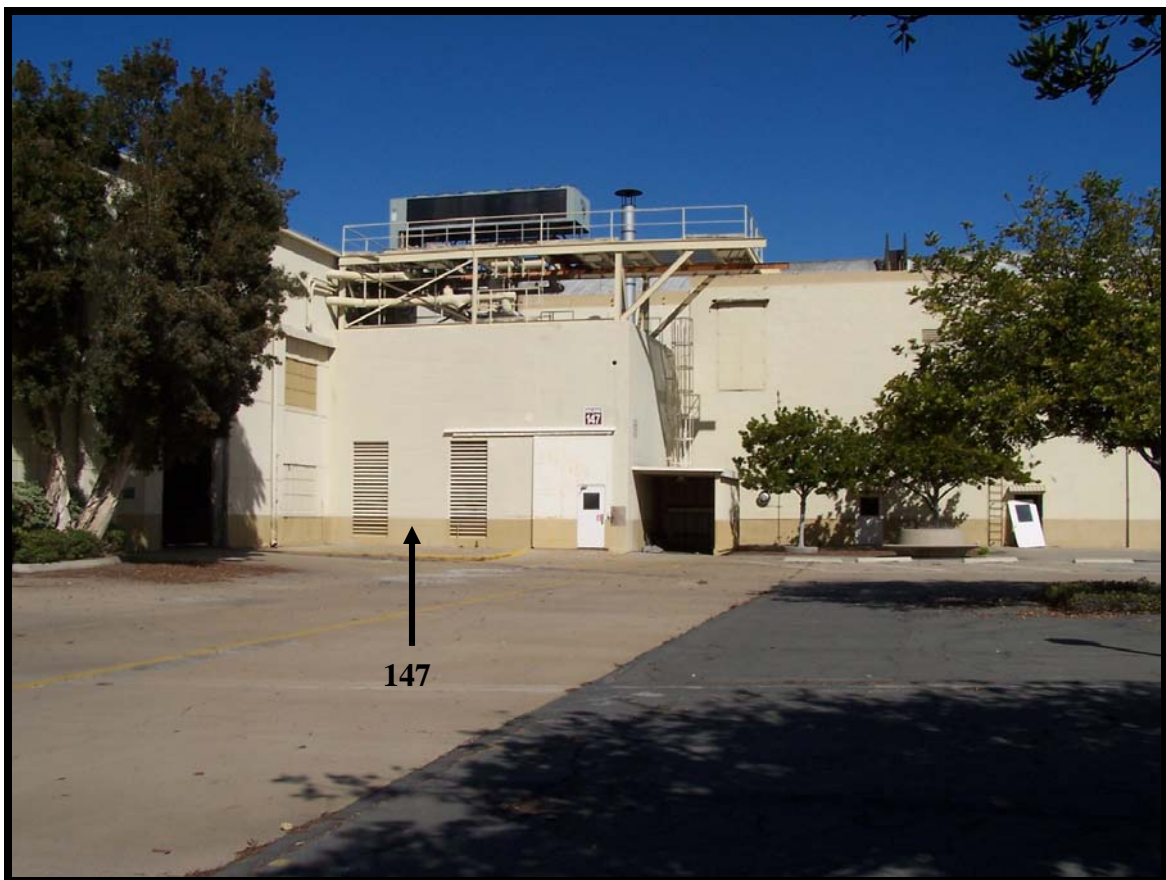
Figure 1: Building 147, a non-contributing element.
