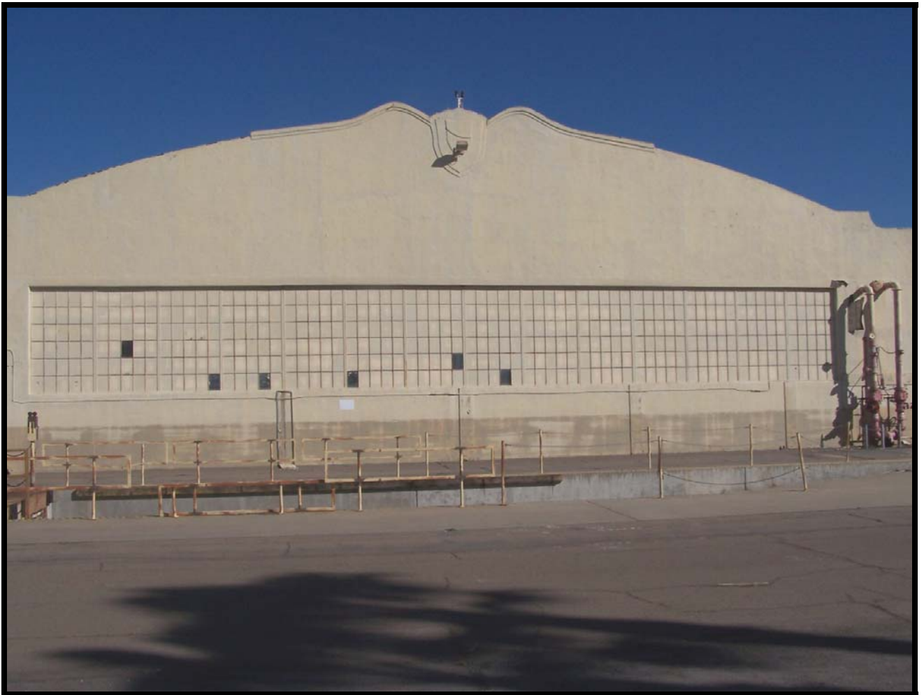
Figure 35: The south (back) side of Building 180. Note the continuous row of windows and the shield molded into the façade at the top of the roofline. This same motif also occurs on east wing addition to Building 180 and on Building 181 and can be seen in the historic photographs in Figures 29, 30, 32, and 33.
