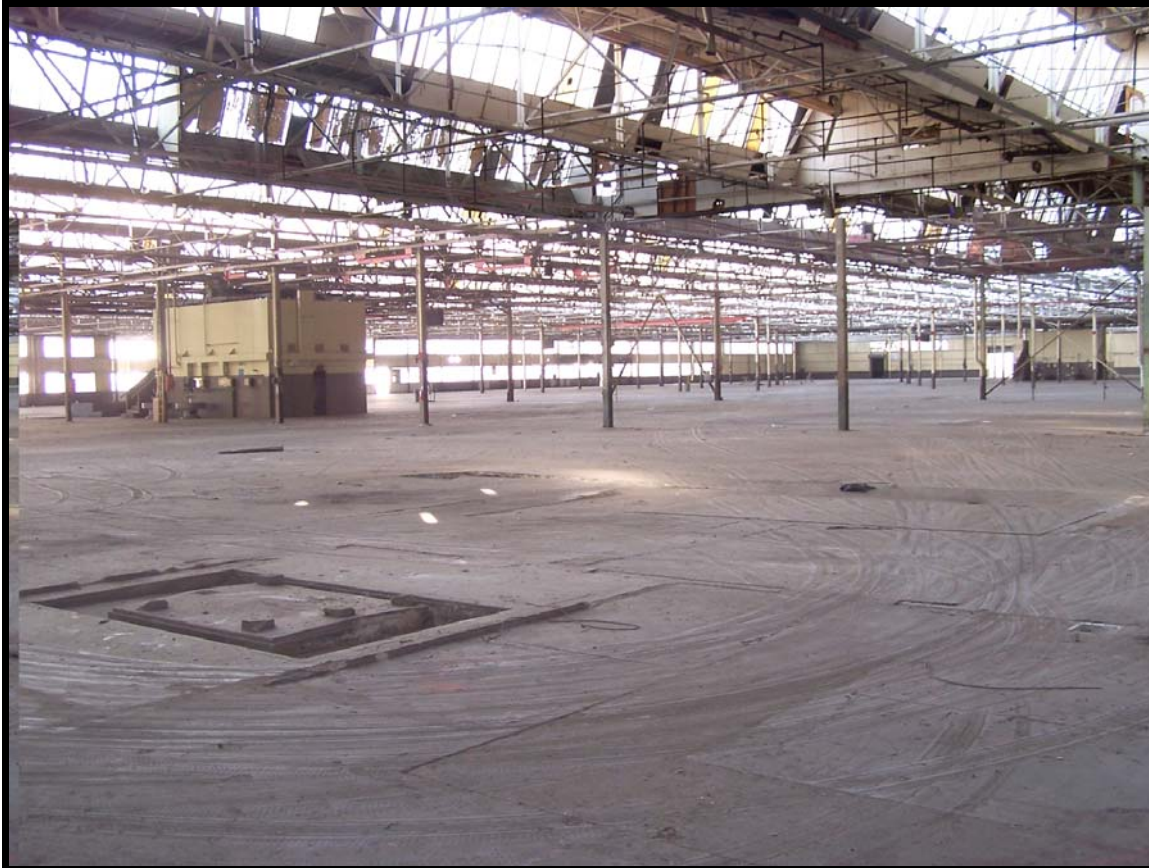
Figure 14: The large open interior of Building 120 illustrating the amount of light provided by the combination of monitor windows in the saw tooth profile roof and rows of continuous rows of windows along the building's sides.
