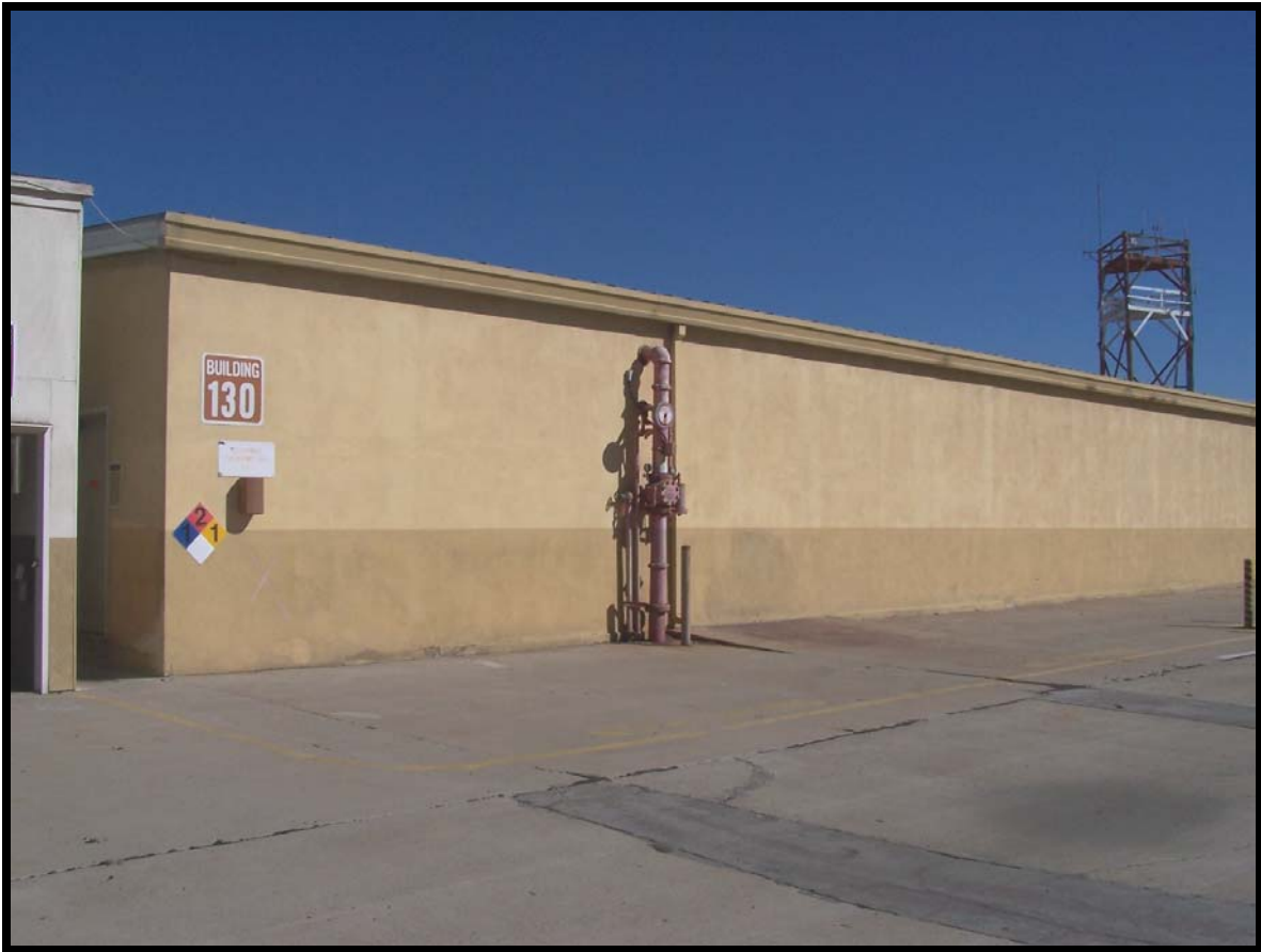
Figure 53: Building 130, a non-contributing element.
