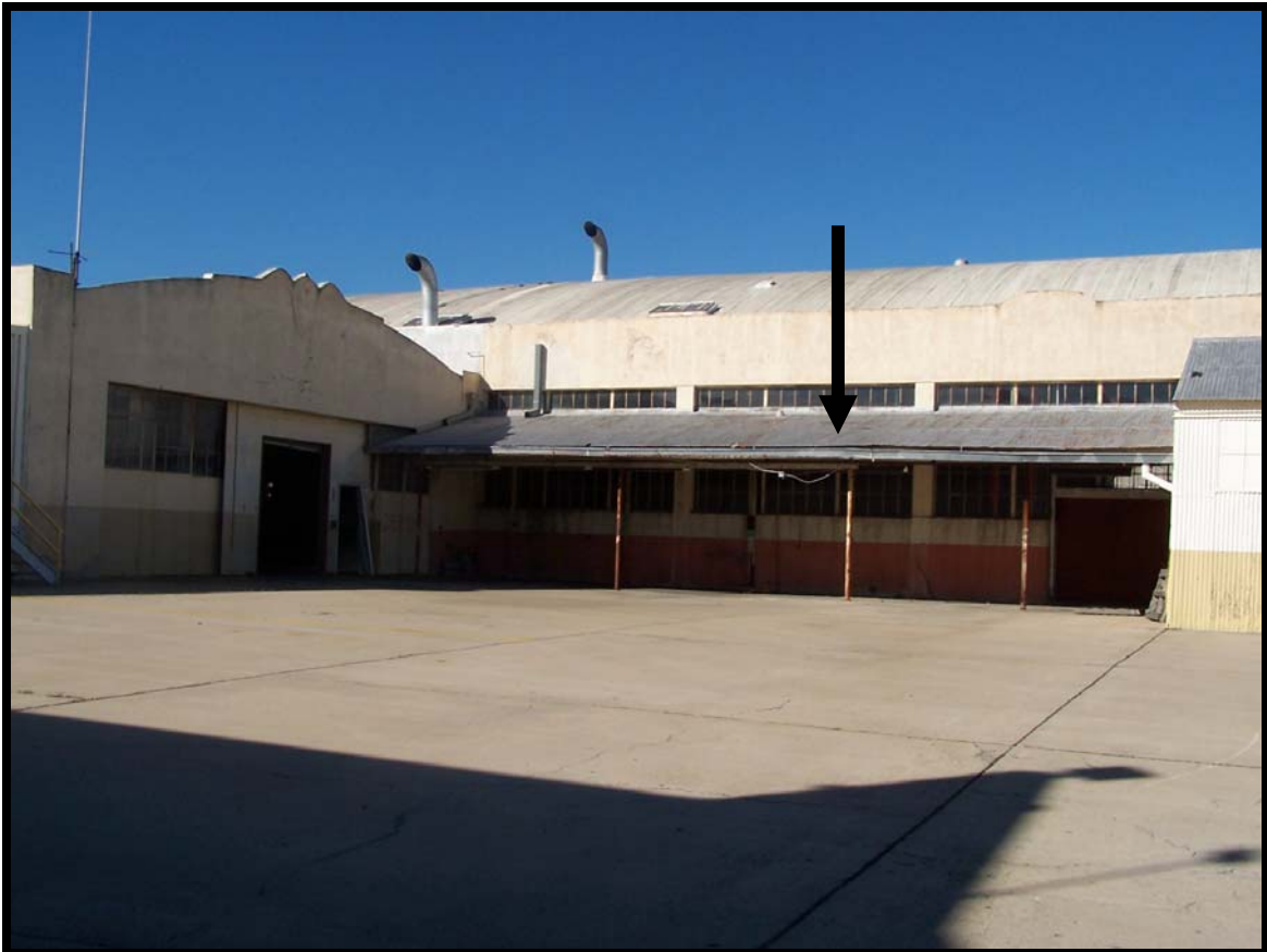
Figure 70: Facility 221, a covered walkway, is not a contributing element.
