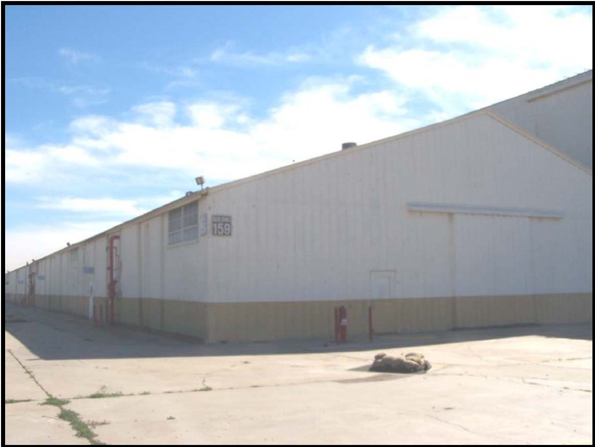
Figure 62: Building 159, a non-contributing element.
