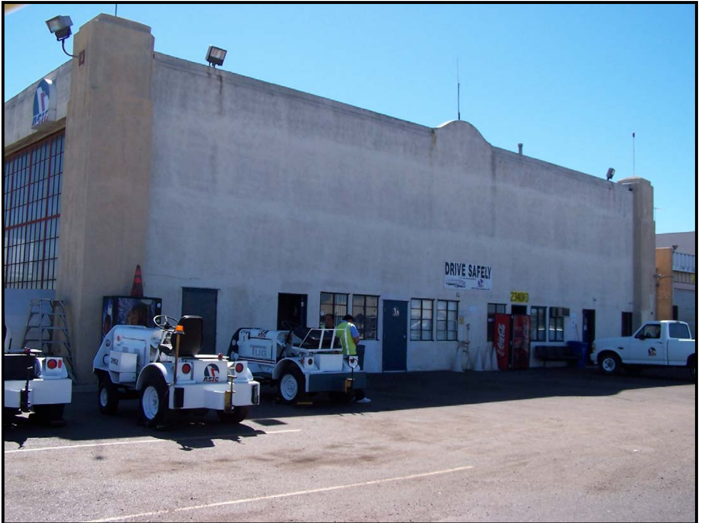
Current (2005) view of the west façade of the 1931 United Airlines Hangar and Terminal, looking southeast.
