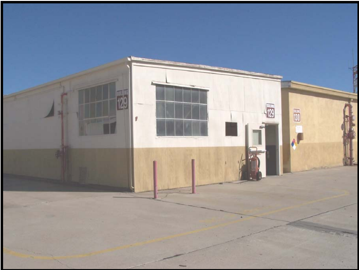
Figure 52: Building 129, a non-contributing element.
