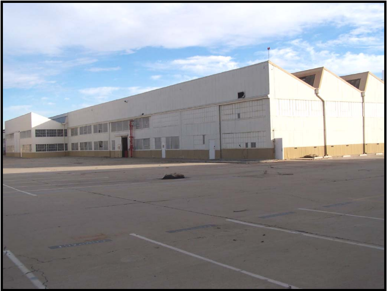
Figure 12: The northwest corner of the Main Factory Building (#120), showing the rows of continuous steel frame windows and saw tooth roof profile characteristic of many aircraft manufacturing plants during World War II.
