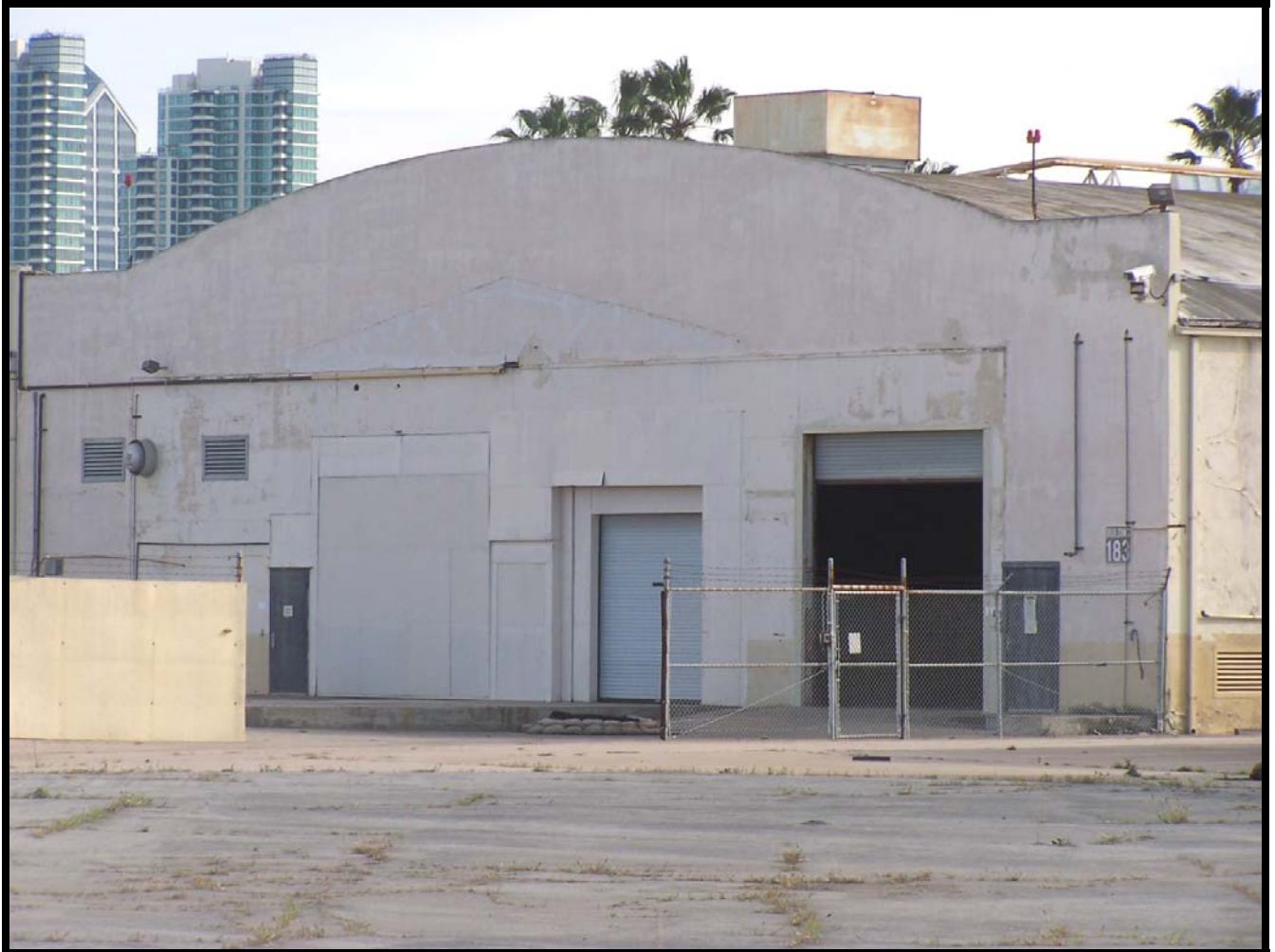
Figure 39: The front (north) side of Building 183.
