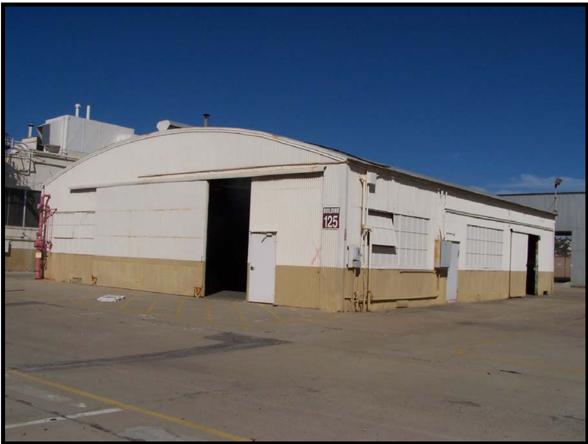
Figure 48: Building 125, a non-contributing element.
