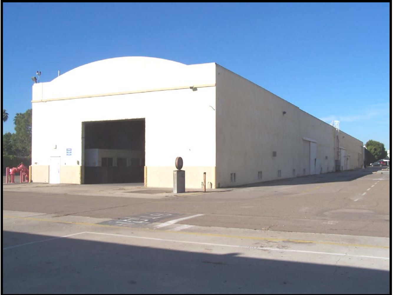
Figure 16: The northeast corner of Building 121. This large warehouse has no windows.
