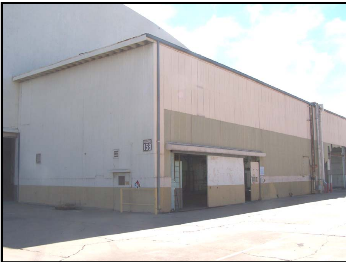
Figure 61: Building 158, a non-contributing element.
