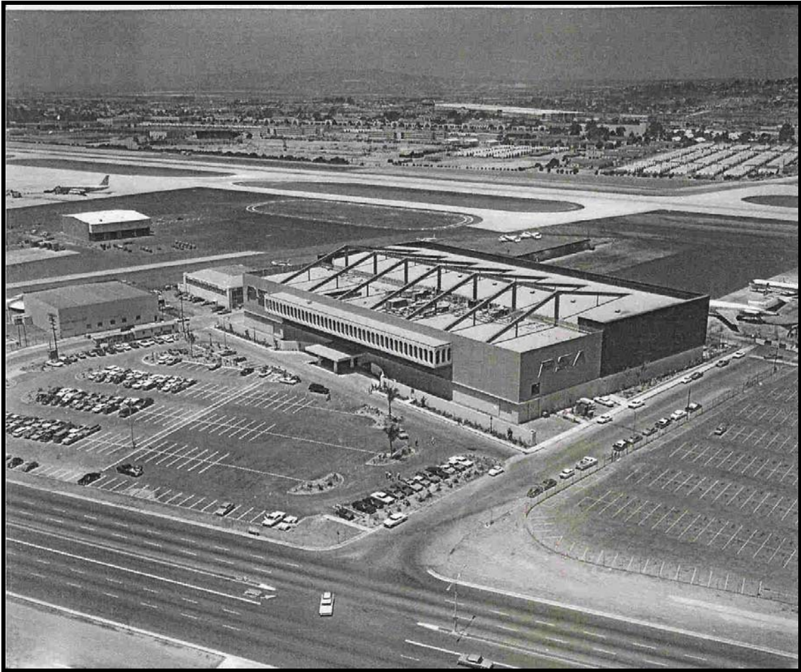
Figure 38: The PSA Headquarters Building completed along Harbor Drive in 1967. It is now (2005) used as the Commuter Terminal (San Diego Historical Society).
