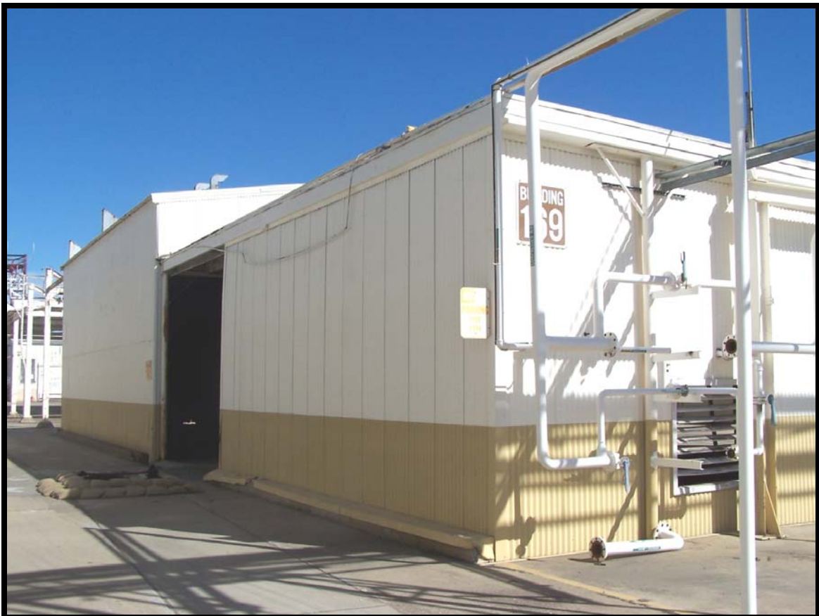
Figure 67: Building 169, a non-contributing element.
