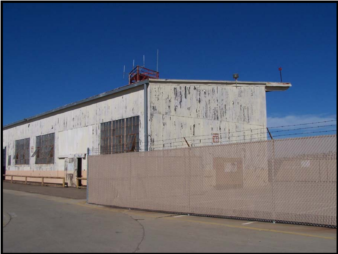
Figure 64: Building 166, a non-contributing element.
