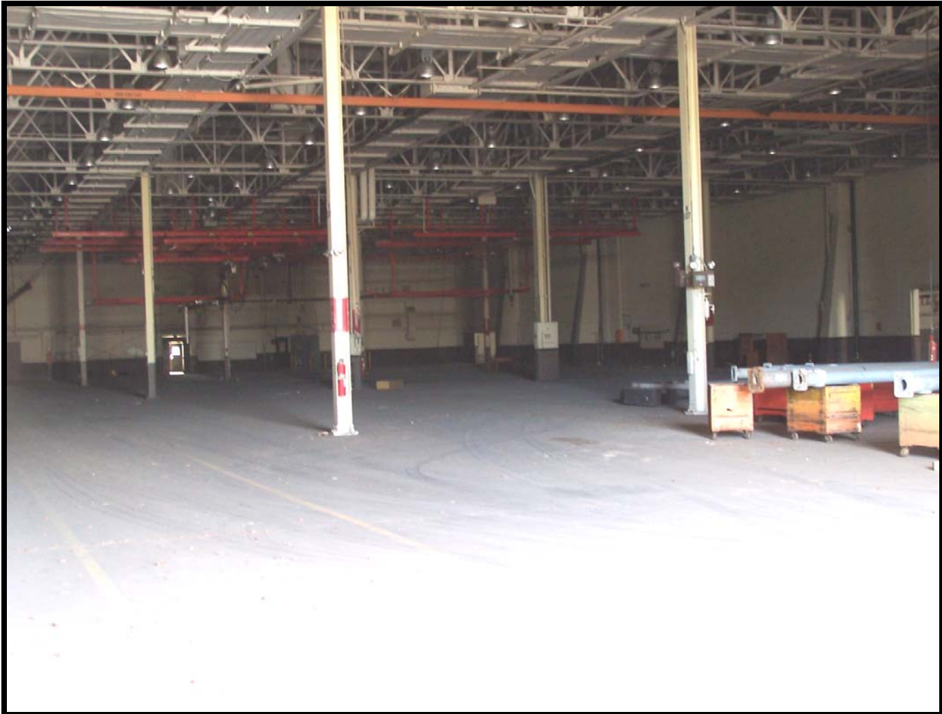
Figure 23: Large open manufacturing plant interior in the north half of Building 146.
