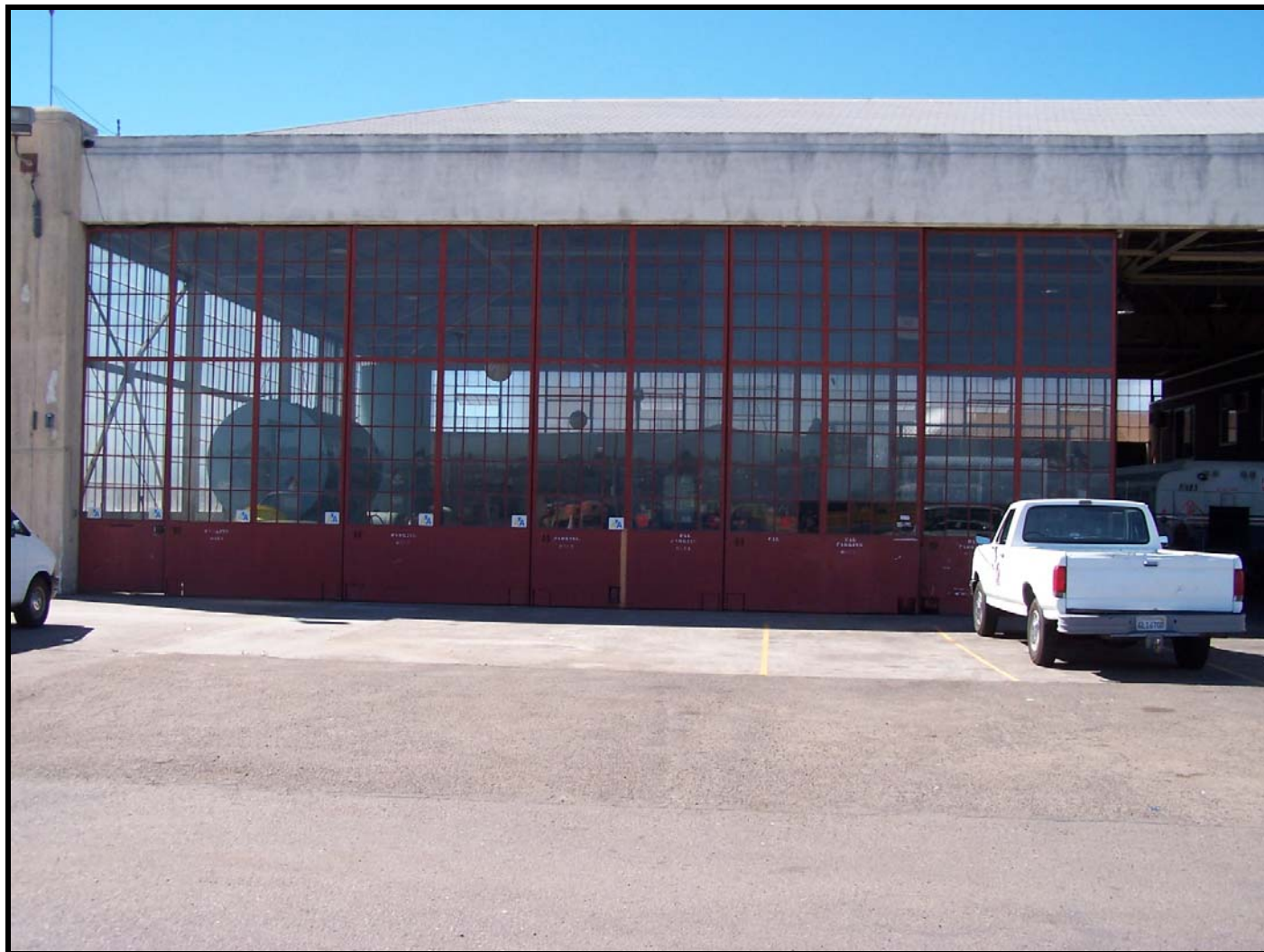
Current (2005) view of the front (north) side of the 1931 United Airlines Hangar, showing the sliding glass curtain wall hangar doors.
