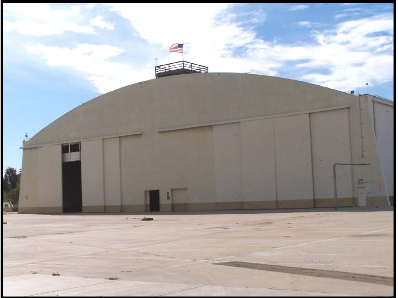
Figure 19: East façade of Building 140, showing the immense hanging wooden doors.
