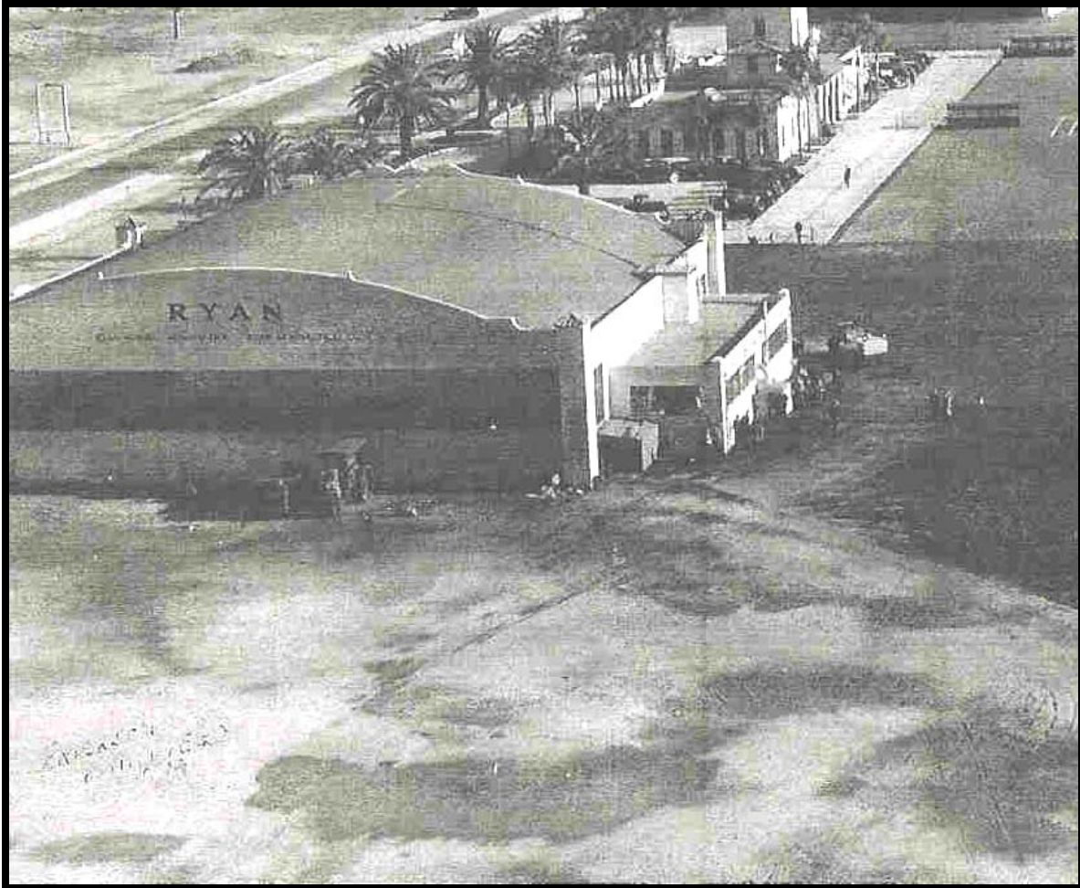
Figure 30: Aerial photograph overview of the Lindbergh Field Administration Area circa 1933 – 1934, showing the east side of the original Ryan hangar that is now the west wing of Building 180. This view shows the original east façade, which is now the north side of the building (San Diego Historical Society).
