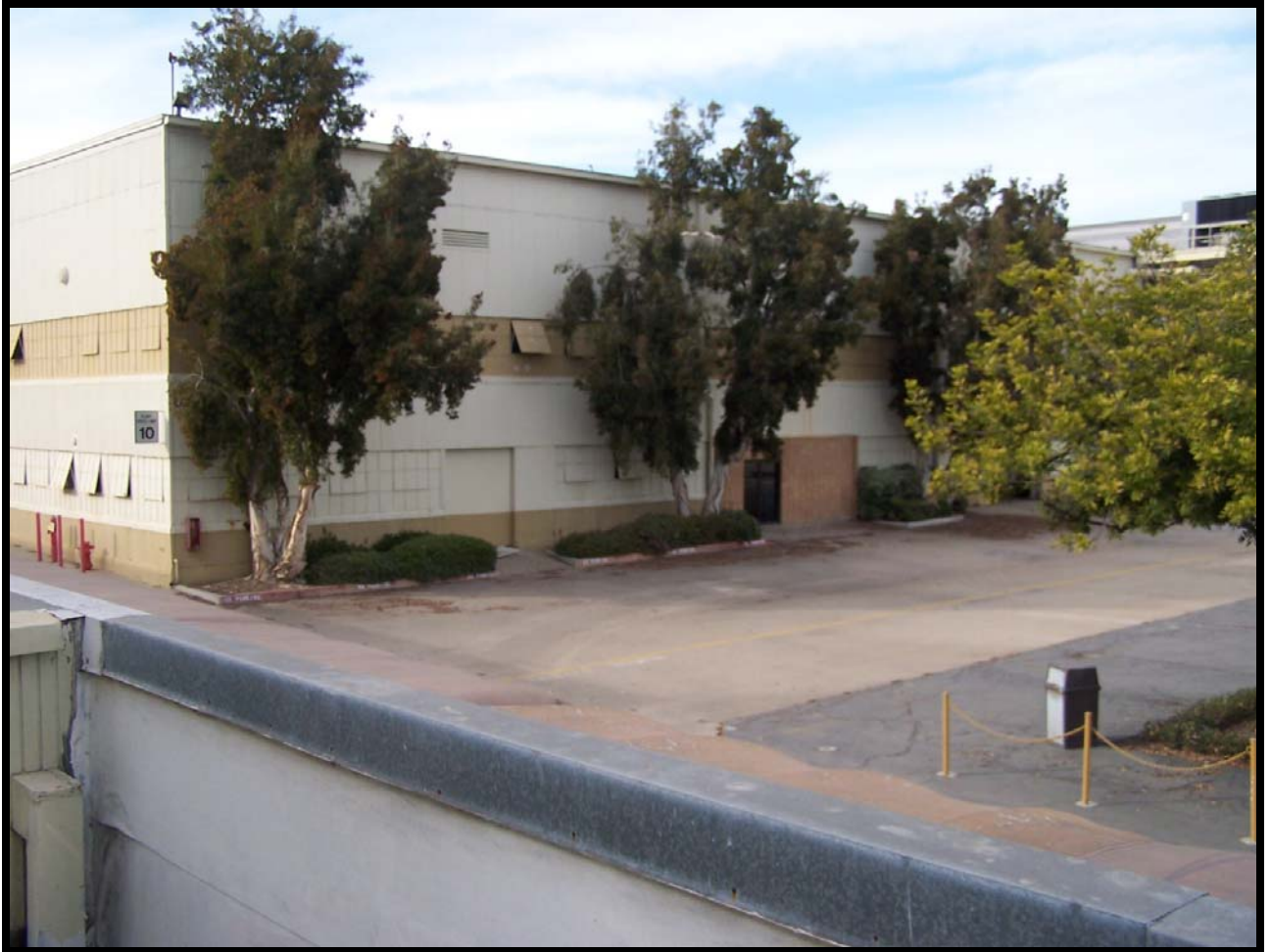
Figure 21: The southeast corner of Building 146.
