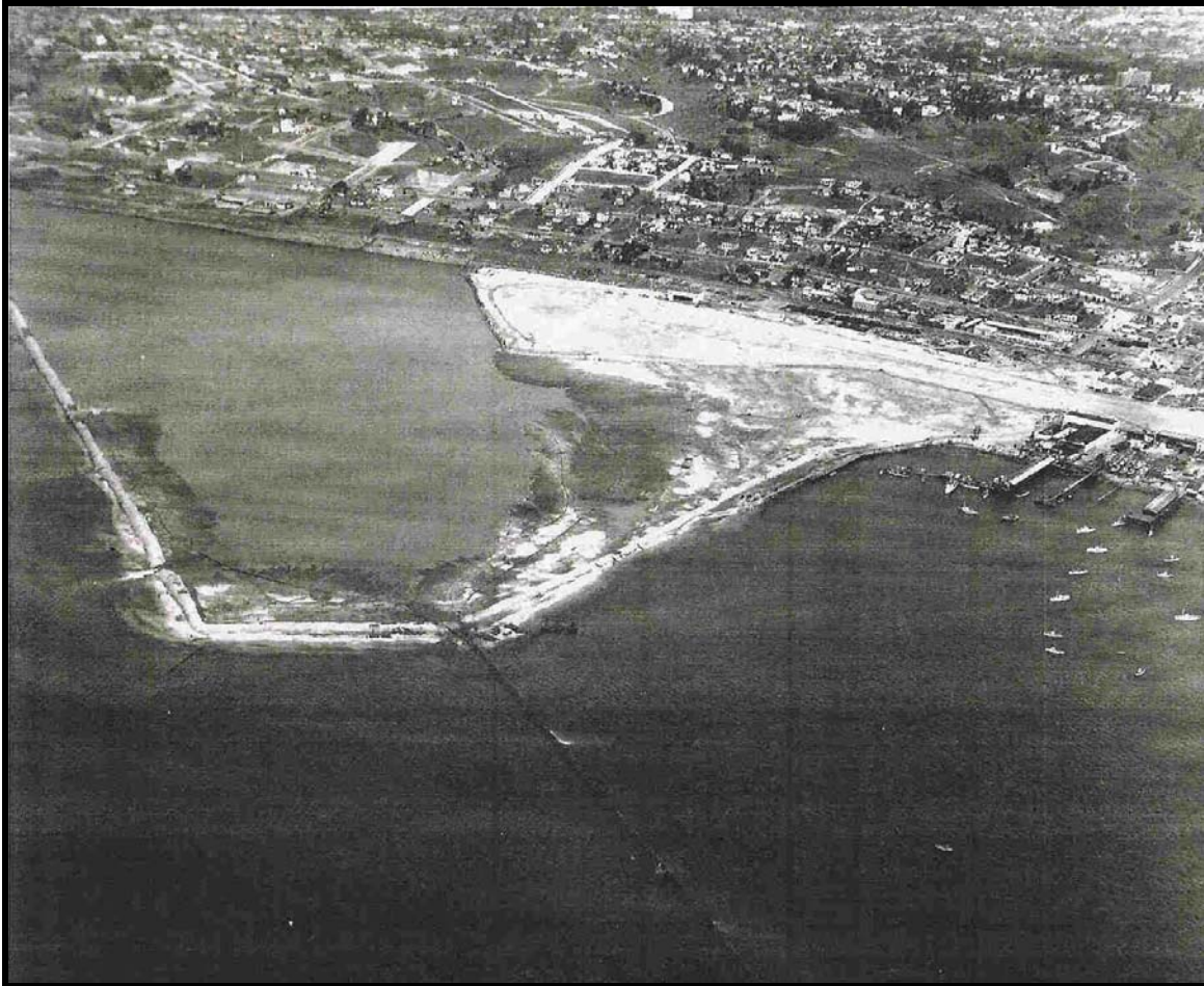
Figure 9: This March 1929 photograph shows dredging operations continuing to reclaim tidelands on the west side of the airport (San Diego Aerospace Museum).
