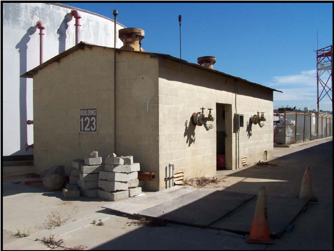
Figure 47: Building 123 (pump station and water tank), a non-contributing element.
