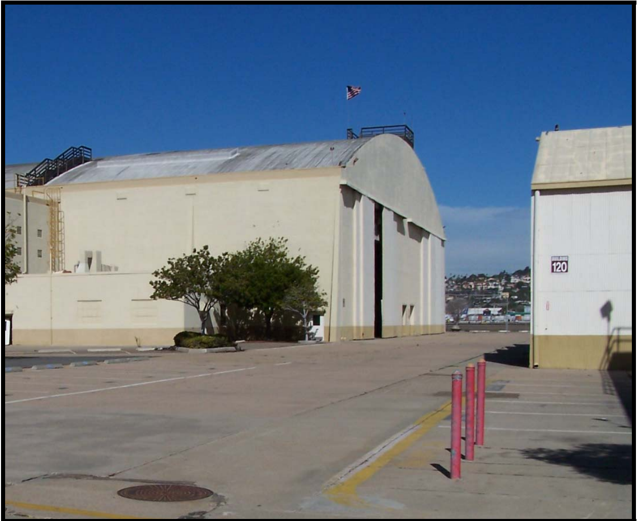
Figure 42: This narrow paved passage on the north side of the lunch area leads between Buildings 140 (on the left) and 120.
