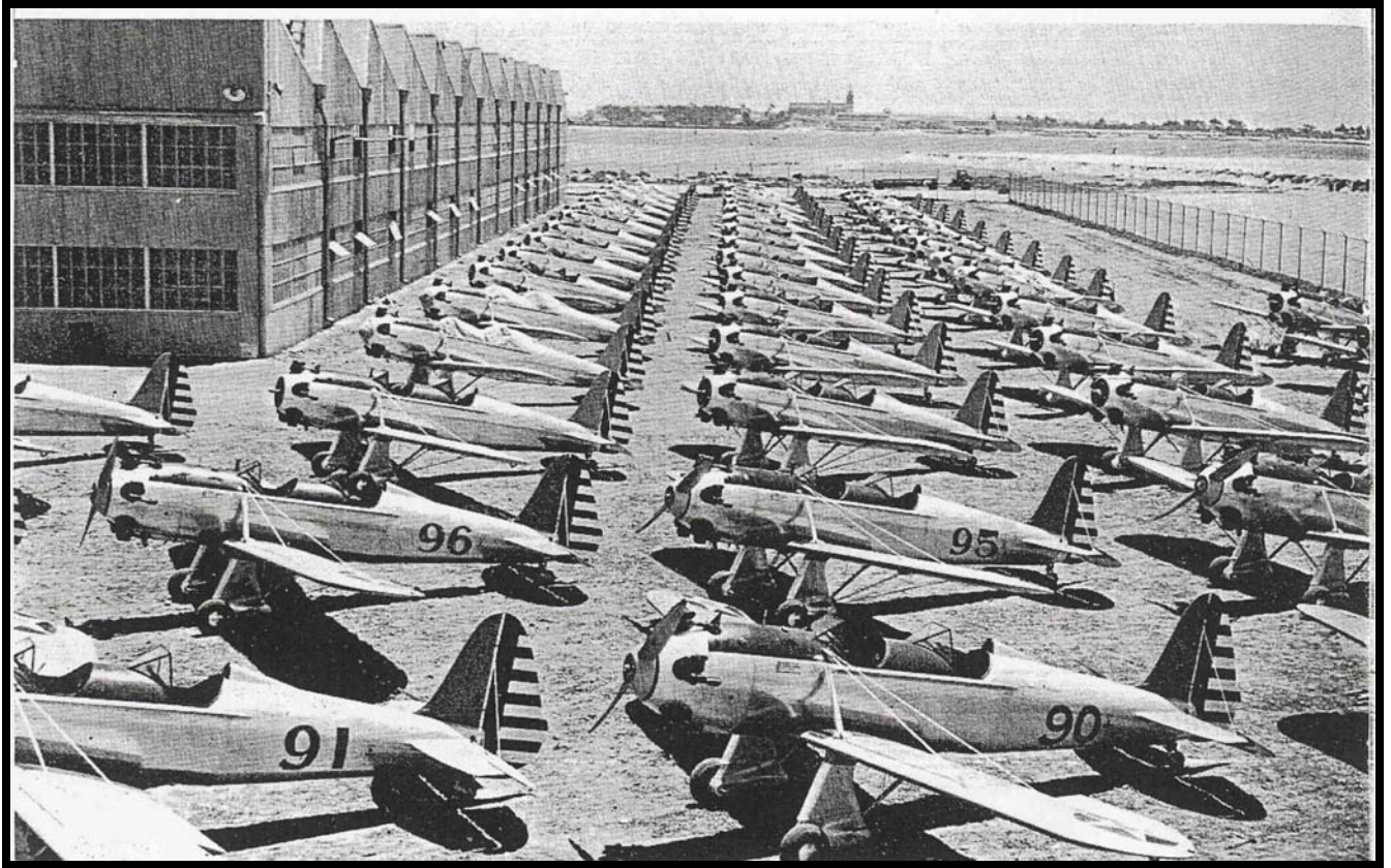
Figure 11: Newly manufactured Ryan P.T. Trainers adjacent to recently completed Building 120 circa 1939 - 40 (Port District 1940).
