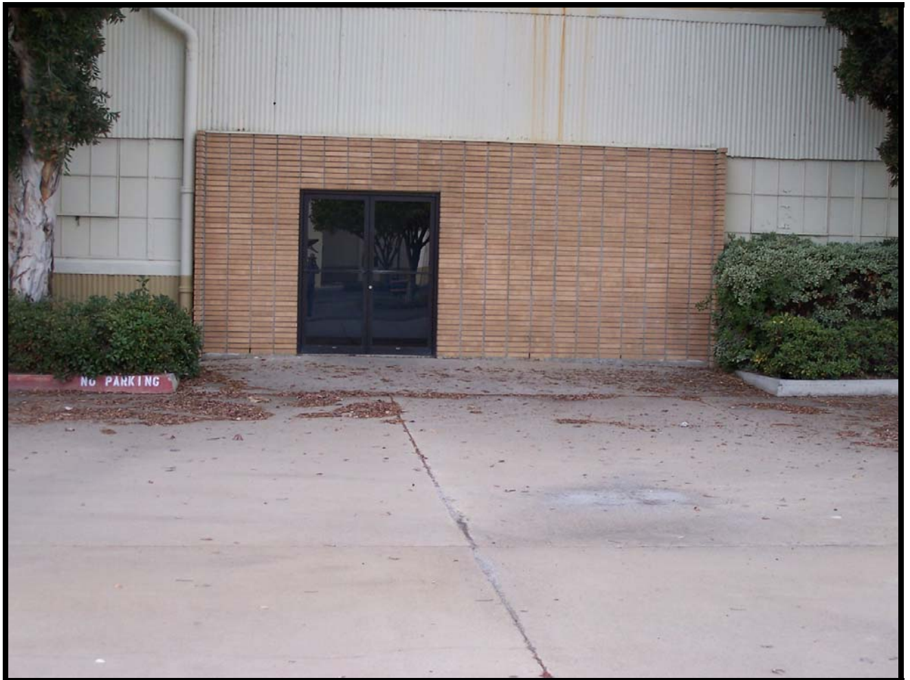
Figure 22: The formal office entrance on the east side of Building 146.
