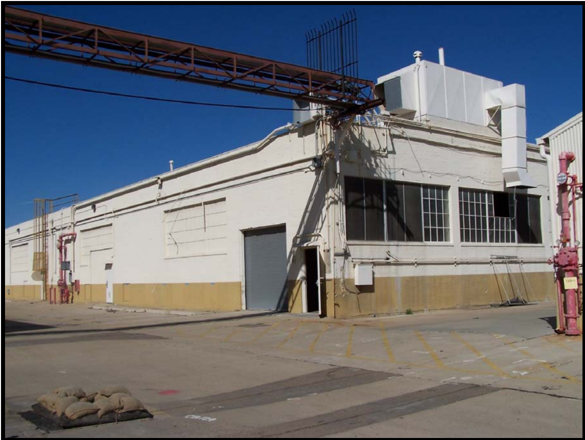
Figure 49: Building 126, a non-contributing element.
