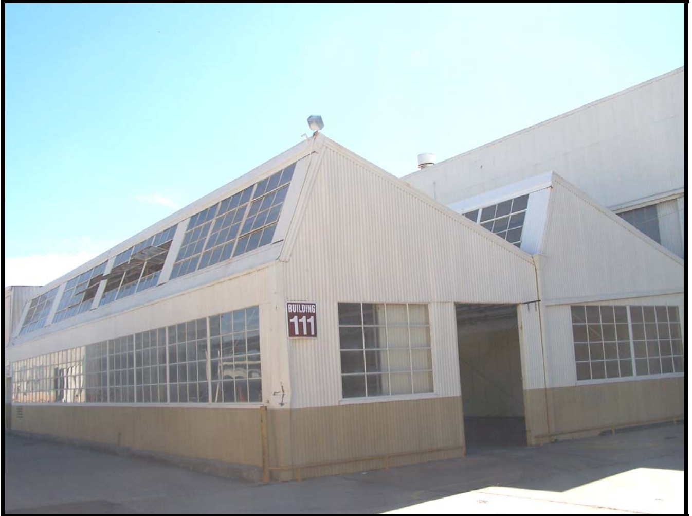
Figure 10: The northeast corner of Building 111, showing the character defining saw tooth roof profile and continuous rows of multi-paned windows.
