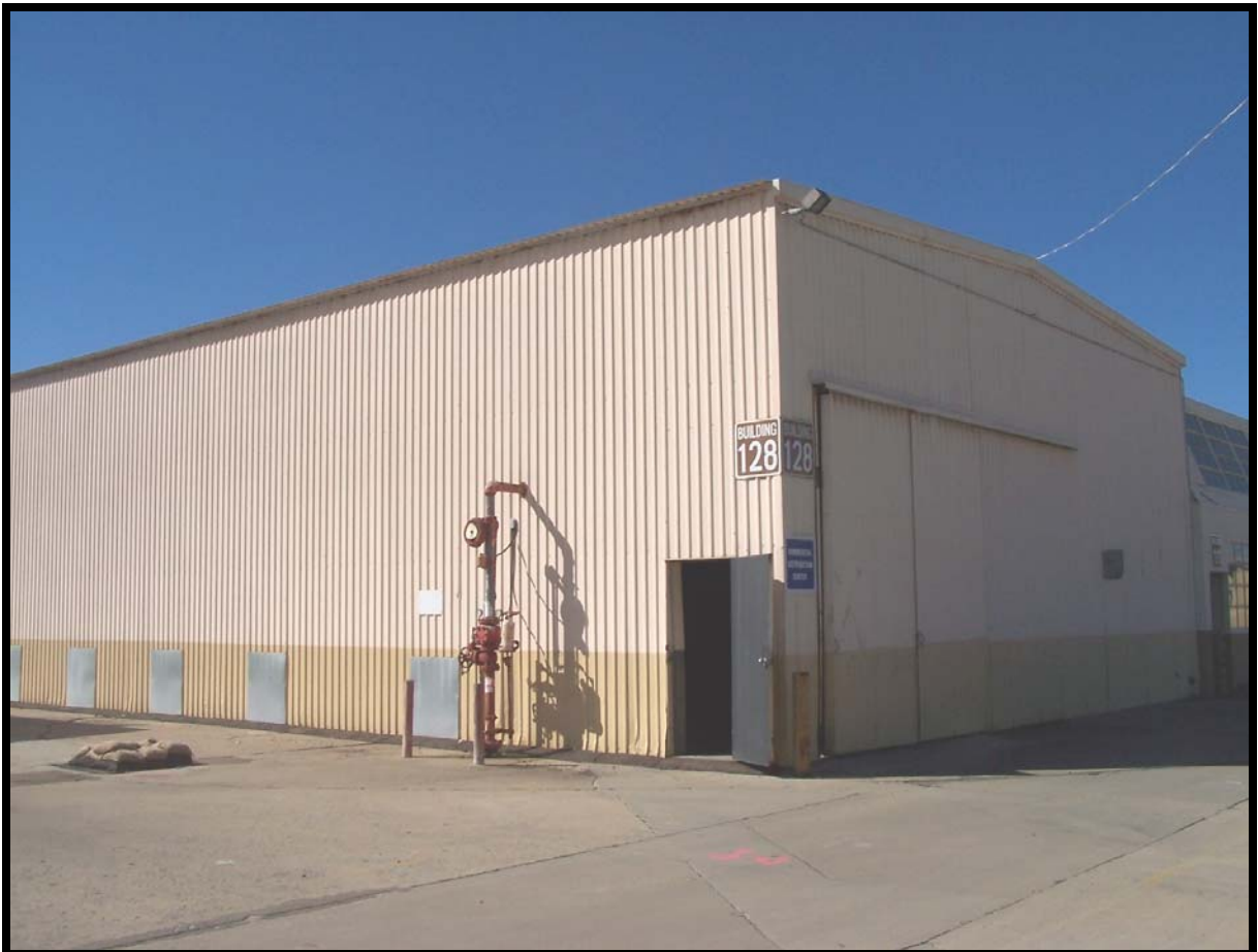
Figure 51: Building 128, a non-contributing element.
