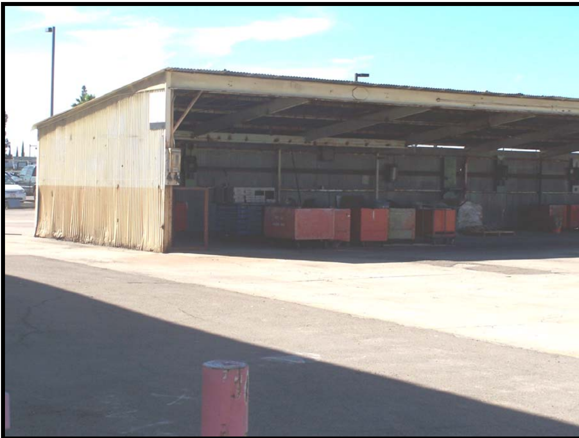
Figure 74: Building 242, a non-contributing element.
