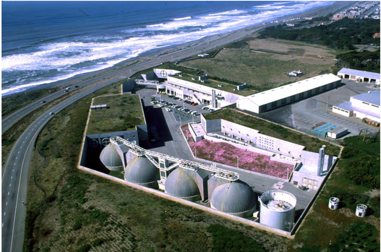
Oceanside Pollution Control Plant
