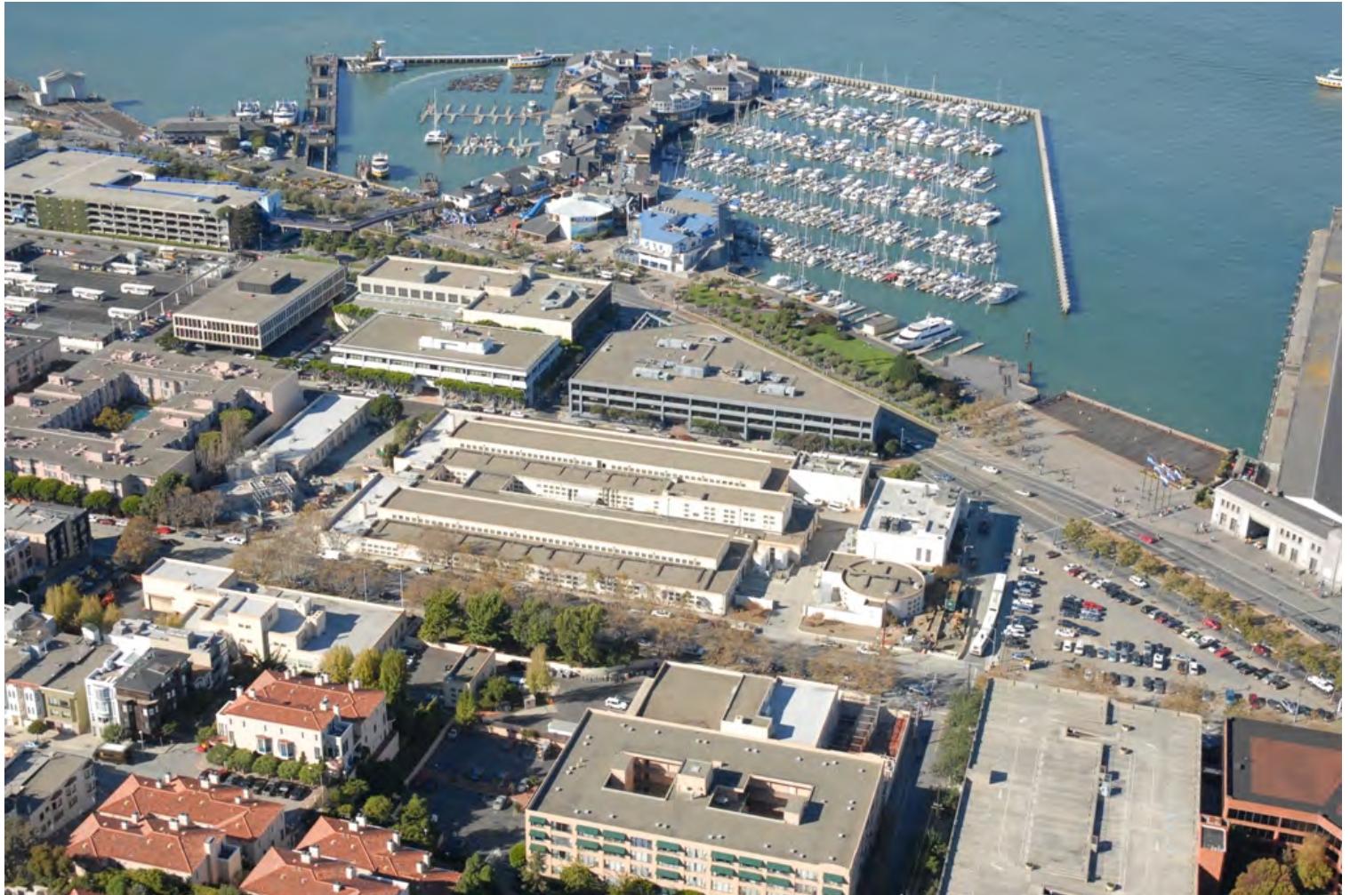
Typical architecture of Treatment Facility located elsewhere
