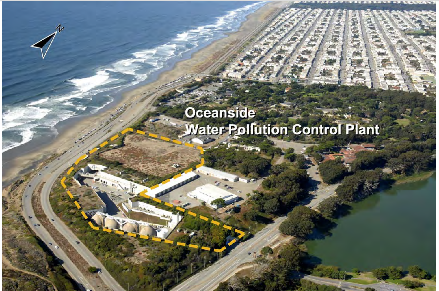
Oceanside Pollution Control Plant
