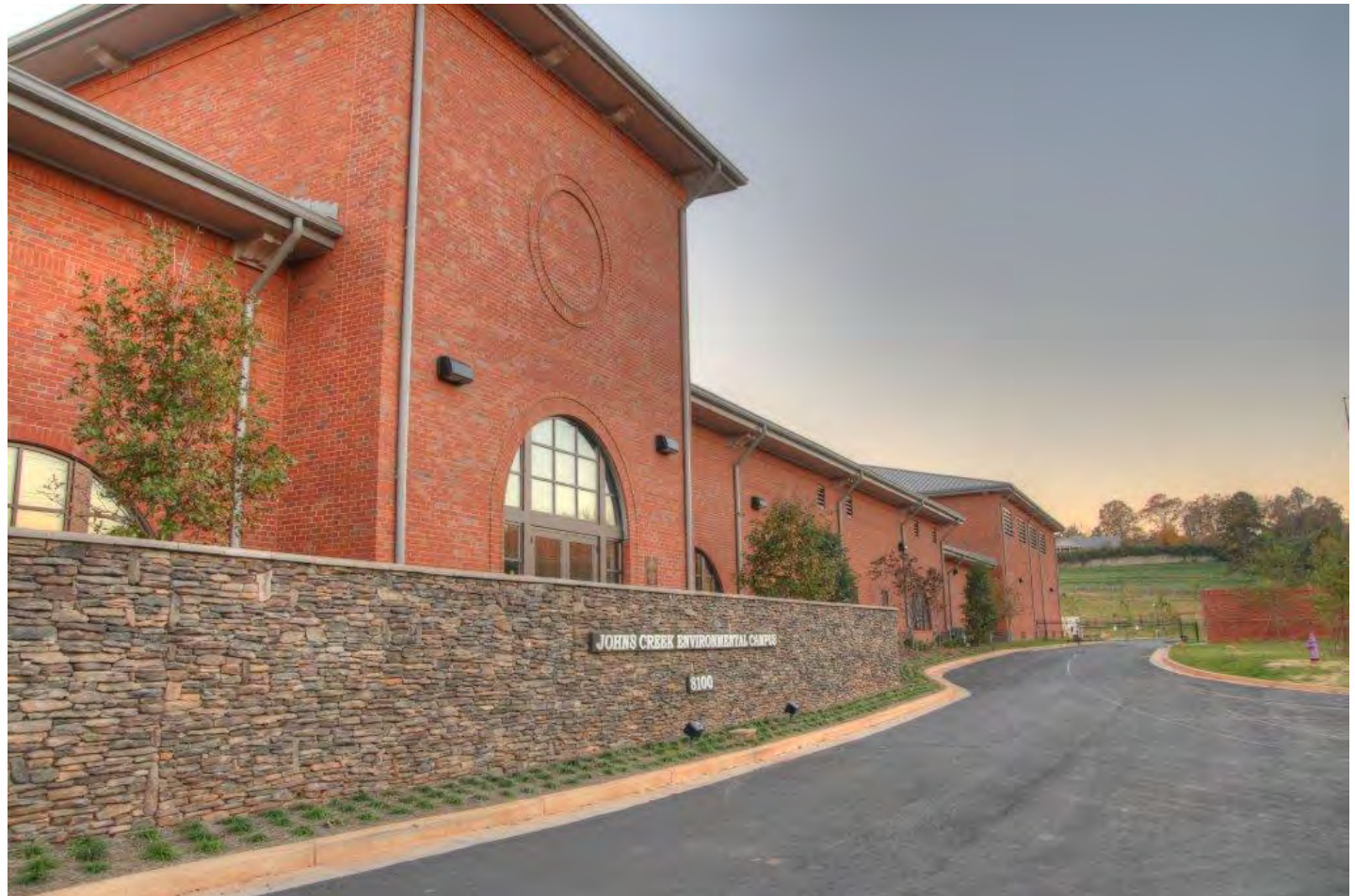
Typical architecture of Treatment Facility located elsewhere
