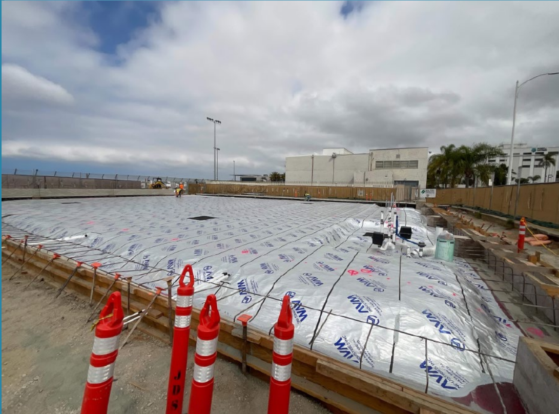
UAHT Vapor Barrier Installed
