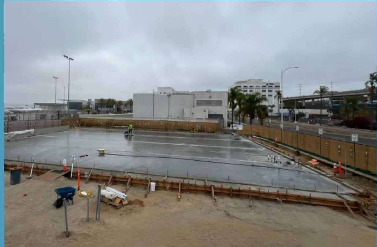
UAHT Slab Being Sawcut
