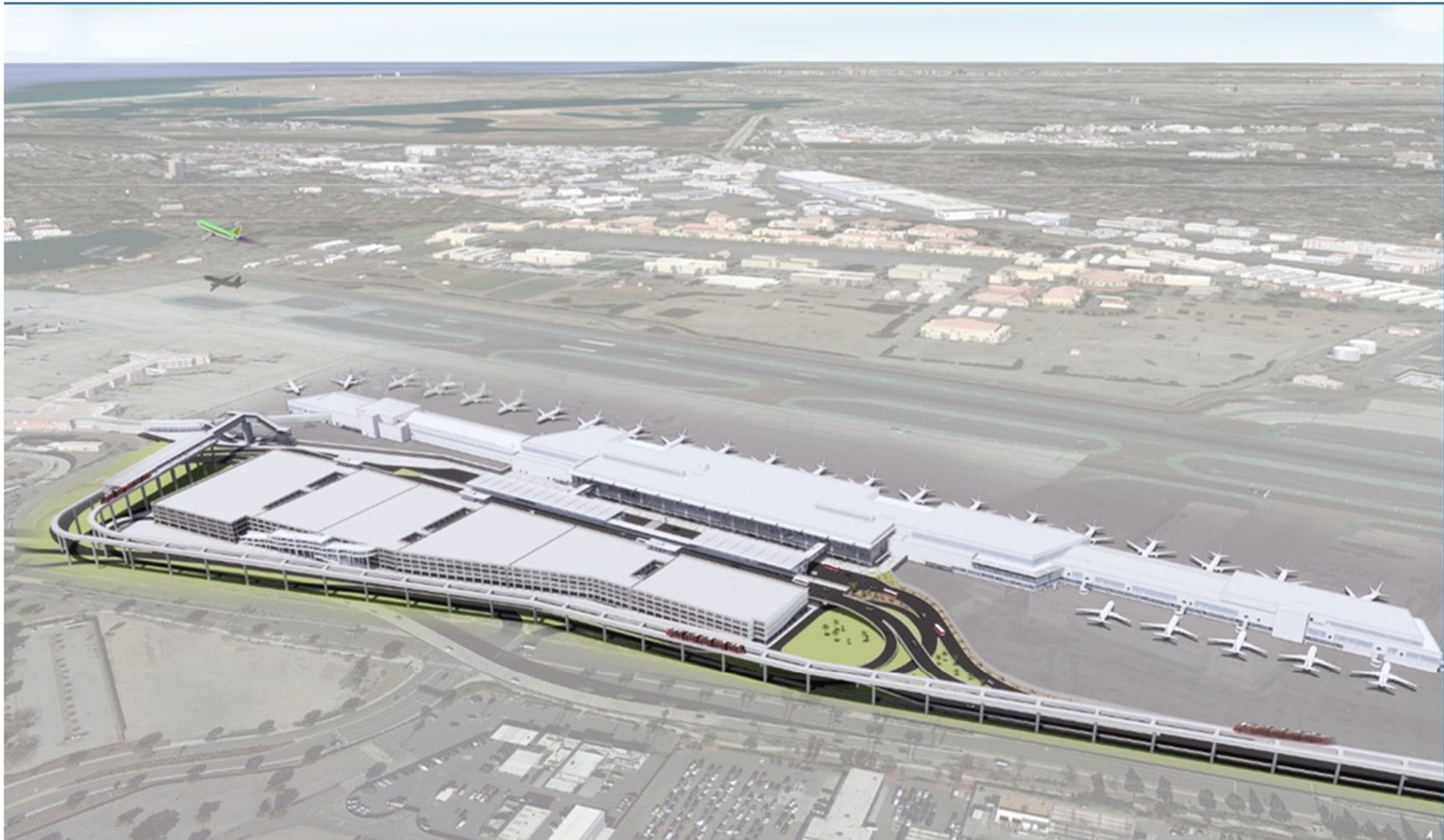
Figure 2 | Aerial View of New Terminal 1 and Associated Facilities
