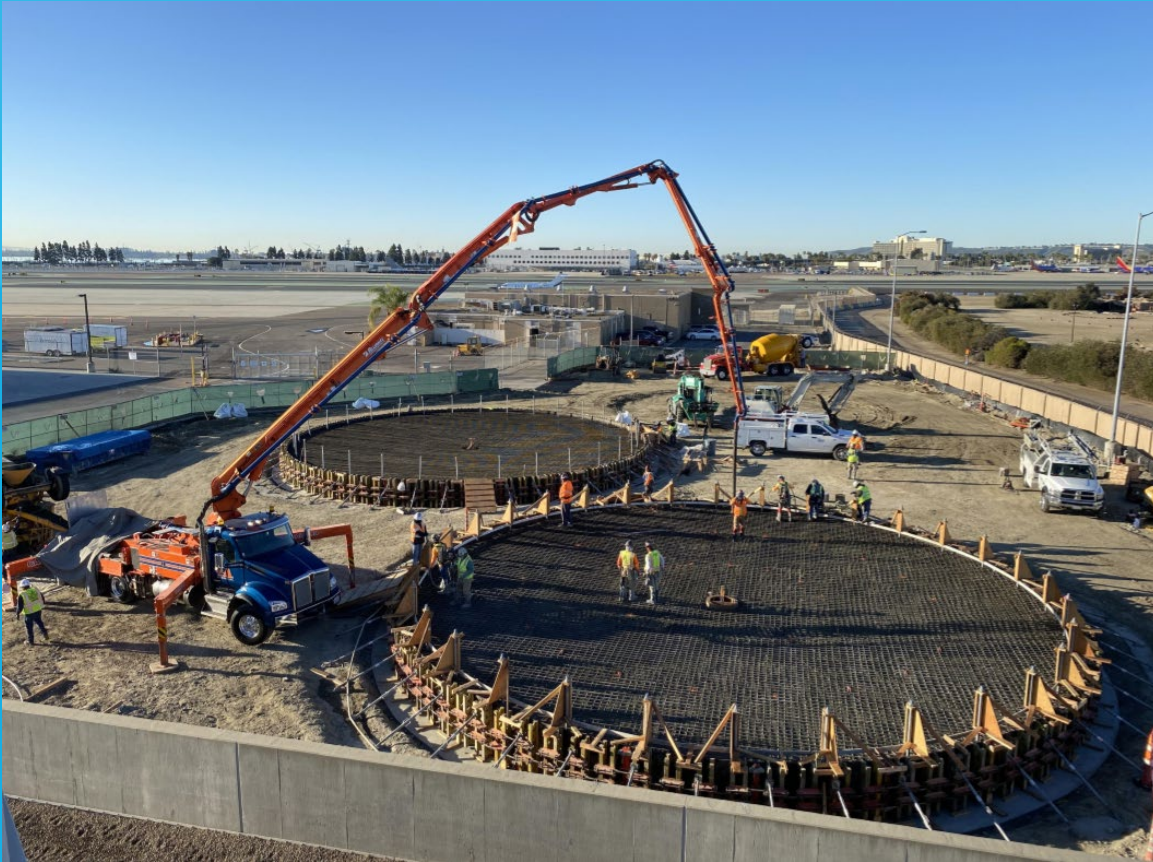
Steel Reinforcements in Place
