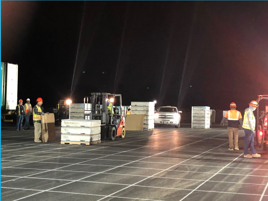
Unloading New EMAS Blocks
