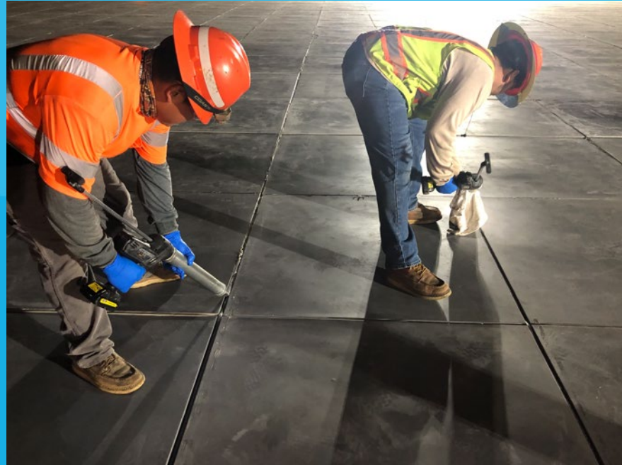
Sealing Joints between EMAS Blocks
