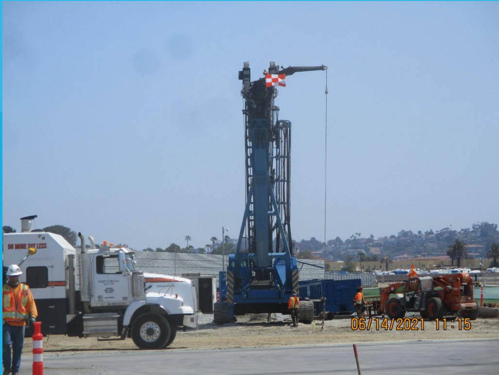
Setting up drill rig
