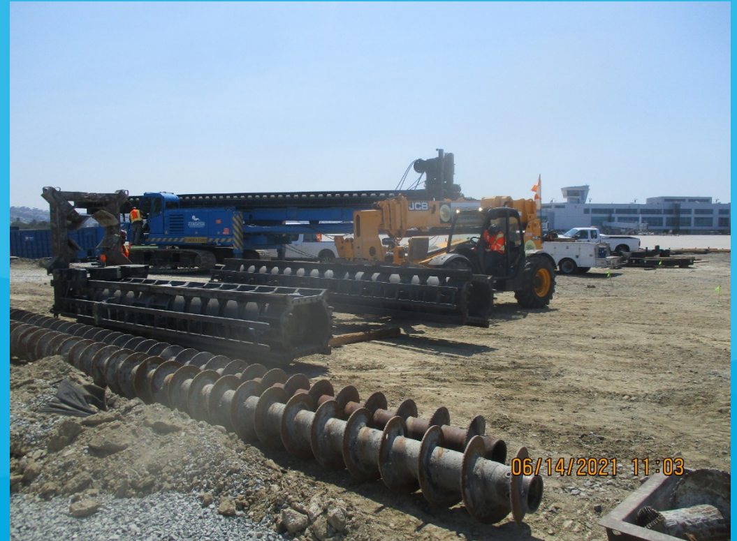
Unloading pile drilling equipment
