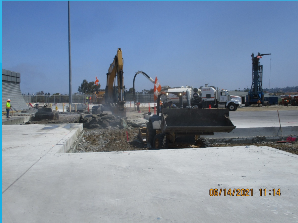
Demolishing concrete apron
