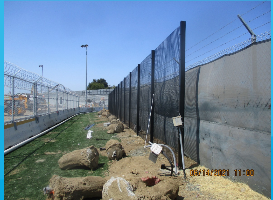
Installing new perimeter fence
