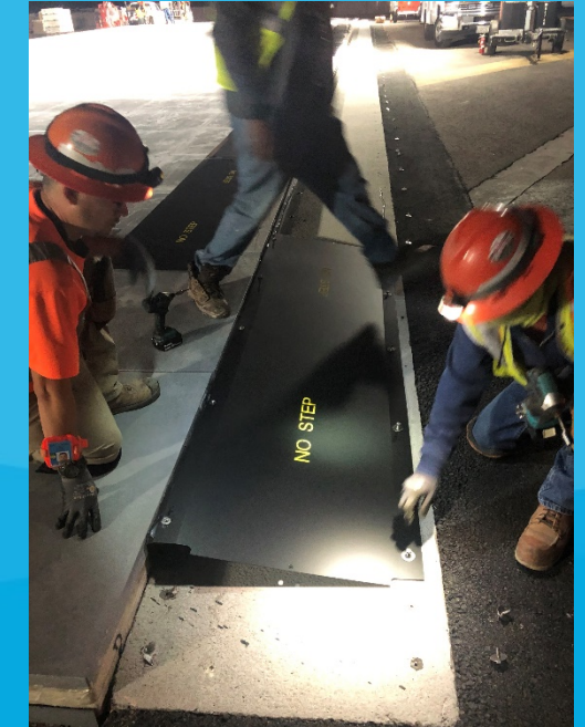
Deflector Shield Installation
