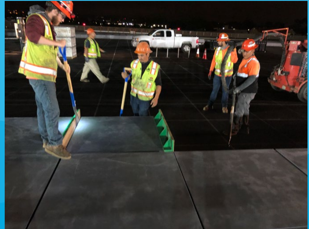
Adjusting New EMAS Block Spacing
