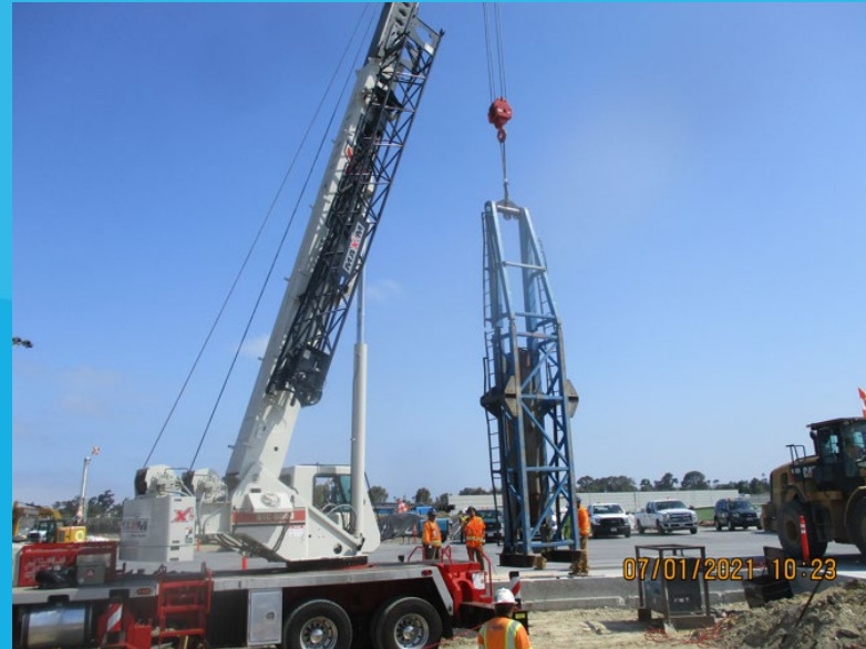
Placing Pile Testing Hammer
