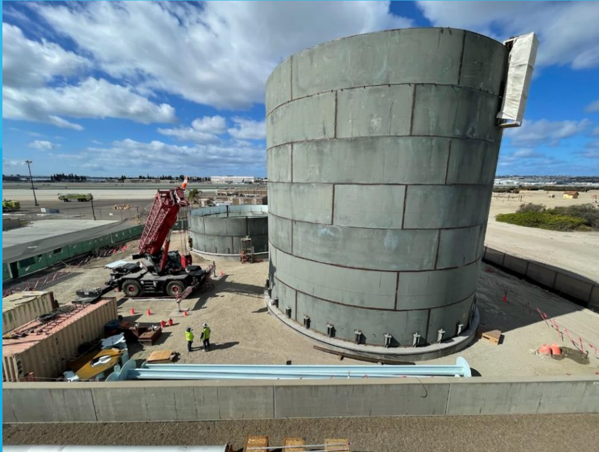
Steel Rings at Tanks 3 & 4
