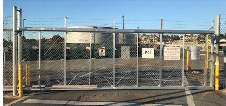
Existing P-01 Gate – sliding gate
