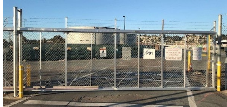
Existing P-01 Gate – sliding gate
