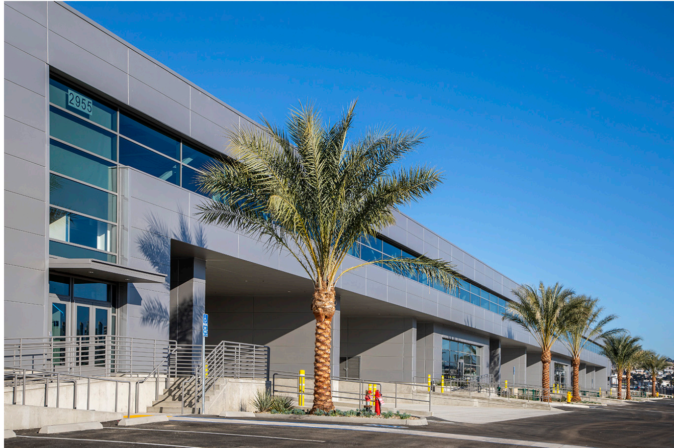
Landside Truck Bays
