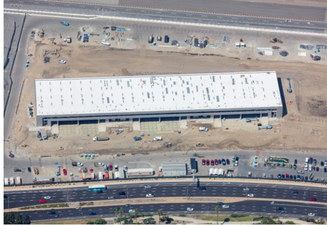
Construction Progress September 2020 Aerial
