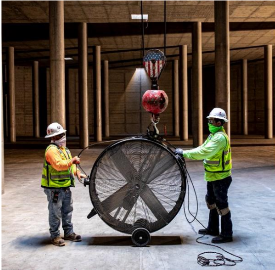
Temp Ventilation Removal
