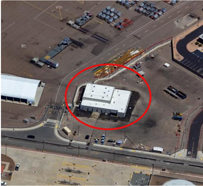
Aerial View of AFO Site September 2020
