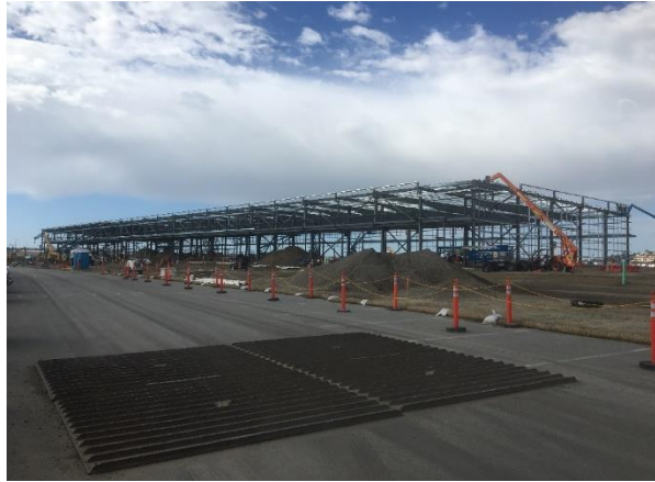
Construction Progress March 2020
