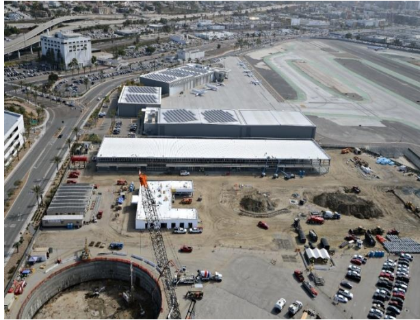
Construction Progress January 2020
