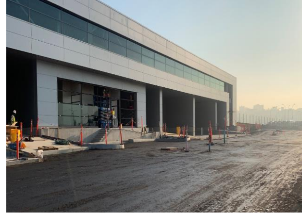
Construction Progress September 2020 Elevation
