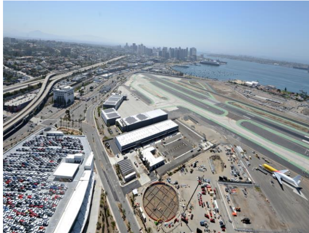
Construction Progress May 2020
