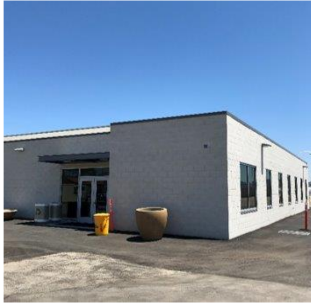
Administrative Building Entry
