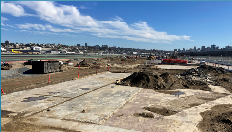
Existing Foundation Discovered During Excavation
