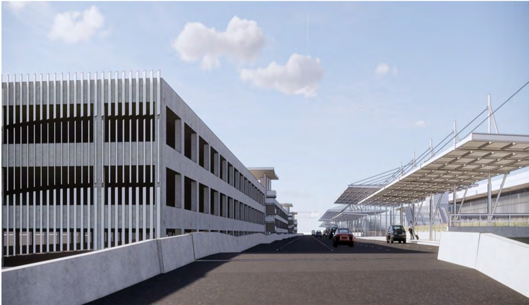
Figure 4 | New Terminal 1 Elevated Departures Roadway
