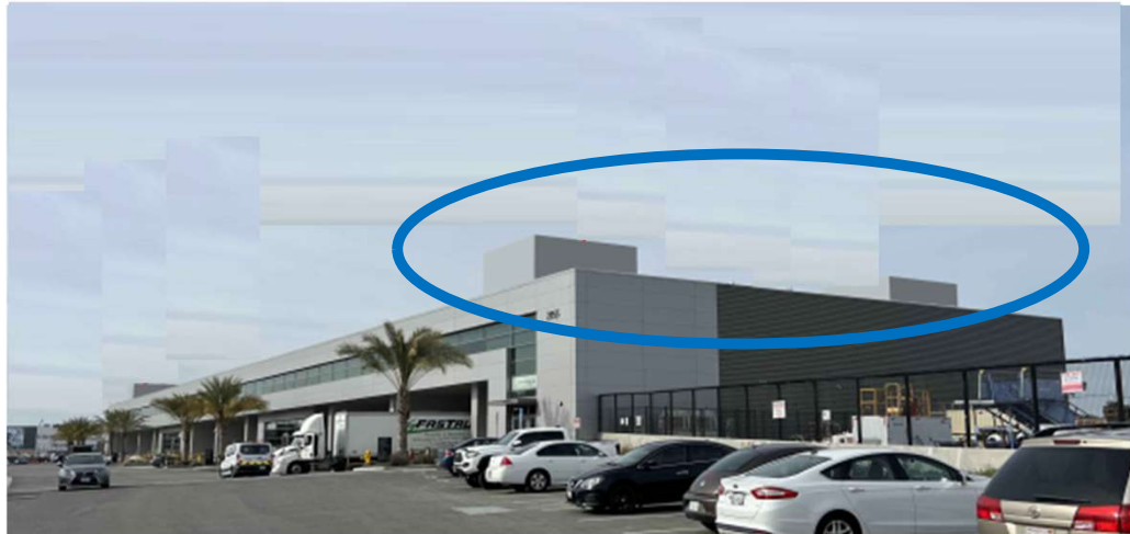
View Northwest in ASB Parking Lot area
