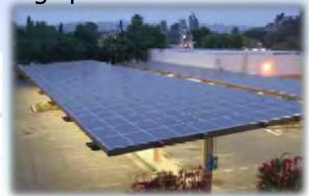
Typical T-structure Carport
