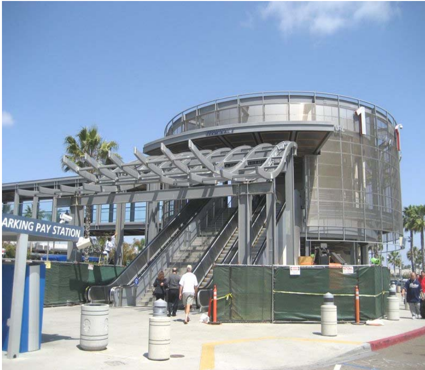
Replace/Protect Terminal 1 Escalators
