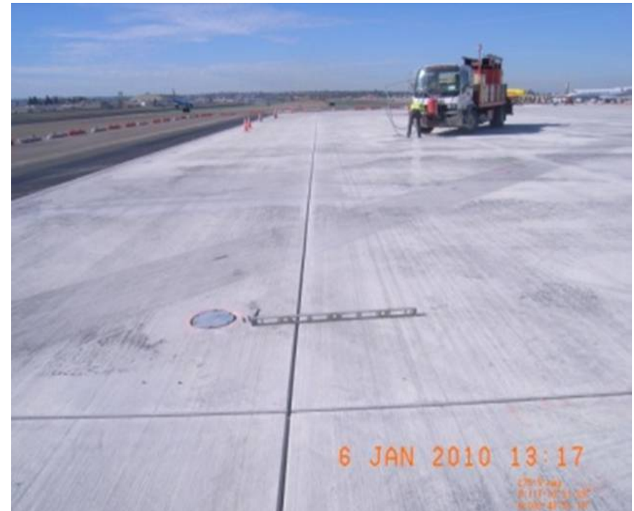
Rehabilitate Taxiway C Submitted for CMAA, ASCE, & APWA Awards
