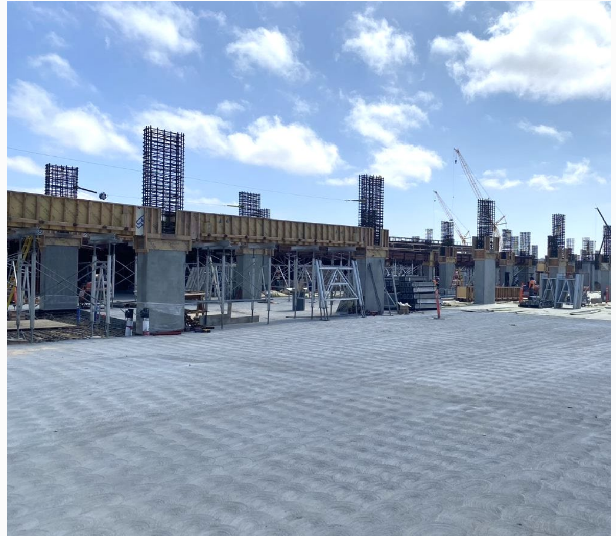
Parking Plaza Slab on Grade Placed
