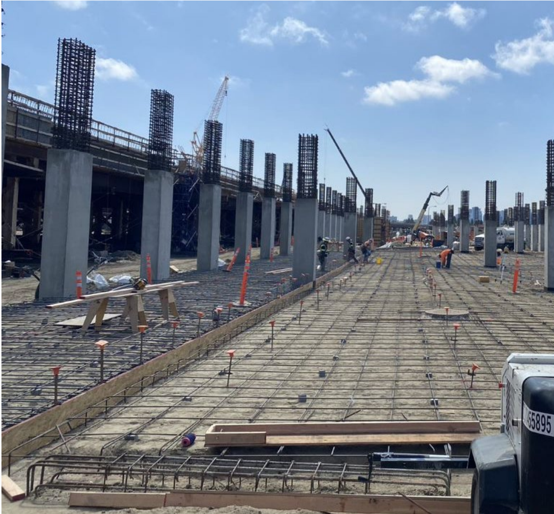
Parking Plaza Slab on Grade Placed
