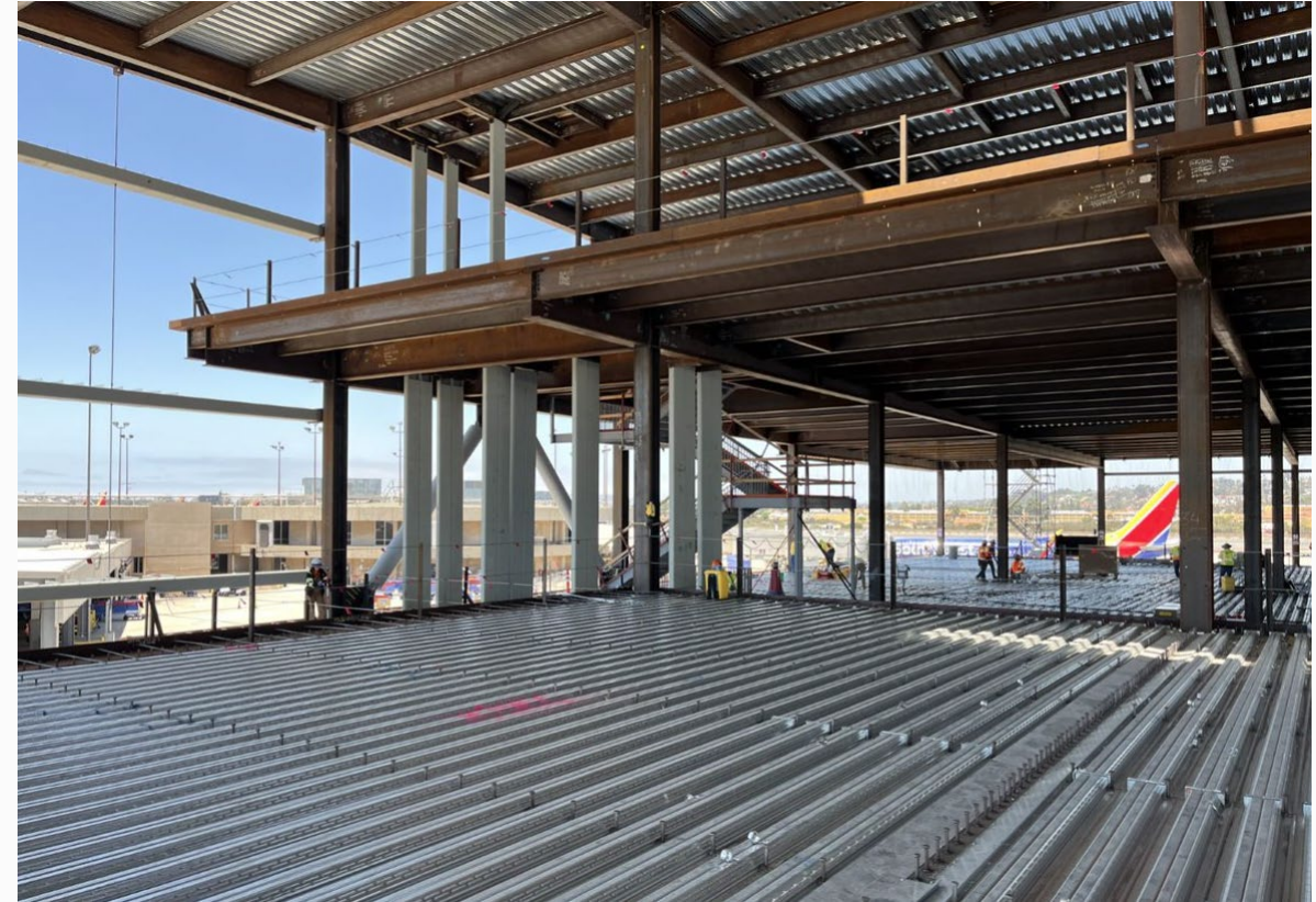
View of Diagonal Steel Bracing & Metal Deck in Progress
