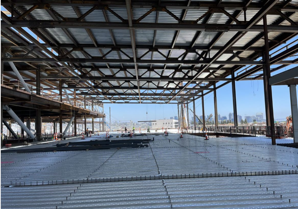
View of Diagonal Steel Bracing & Metal Deck in Progress
