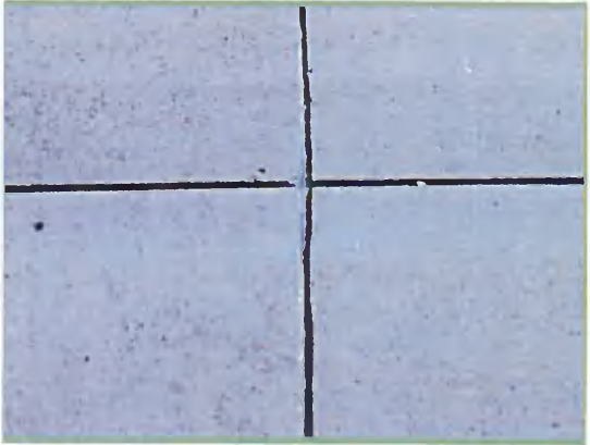
Taxilane B, Section 01 – Joint Seal Damage
