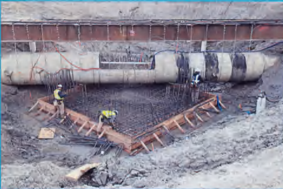
Storm Drain Construction Manhole #1
