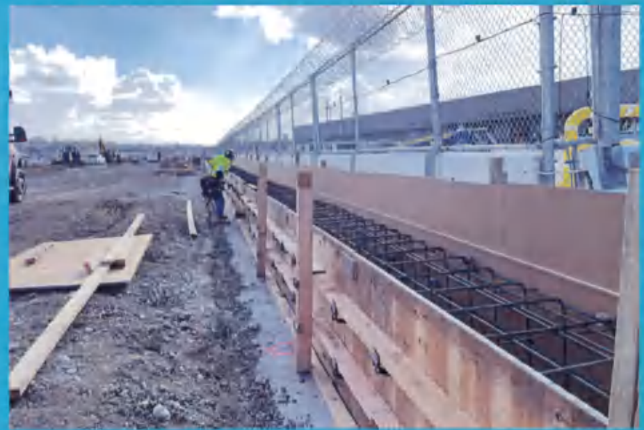
Phase 3A Jet Blast Barrier Construction
