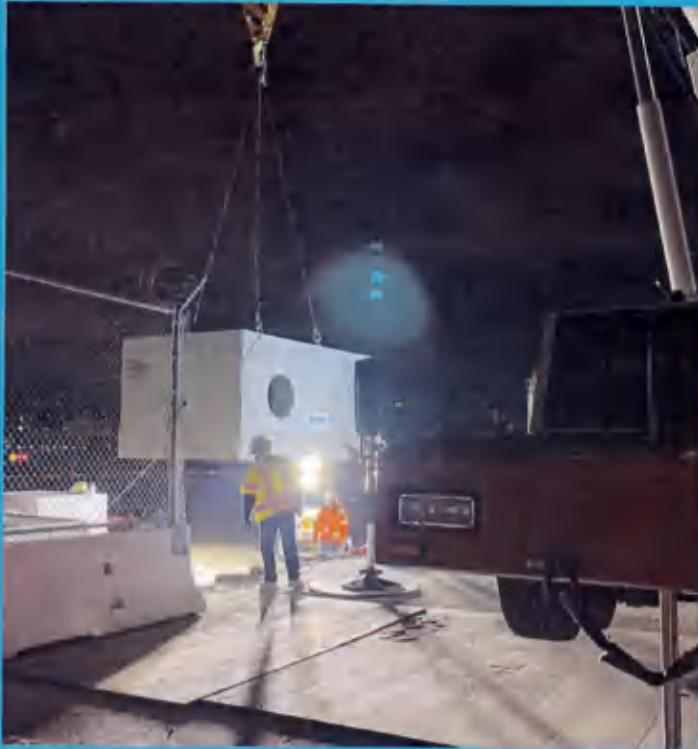
Setting of Infiltration Vault #8
