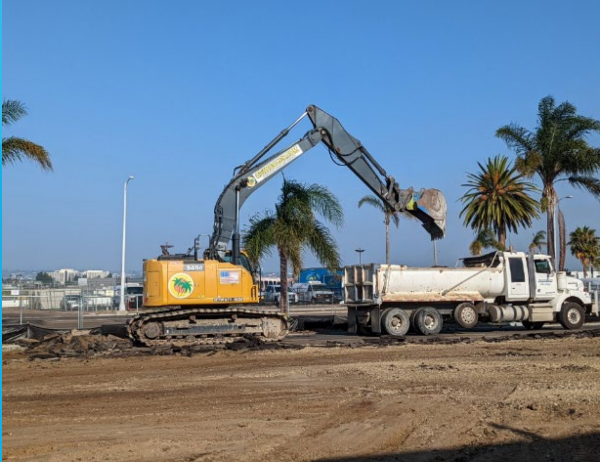
Pavement Demolition and Removal
