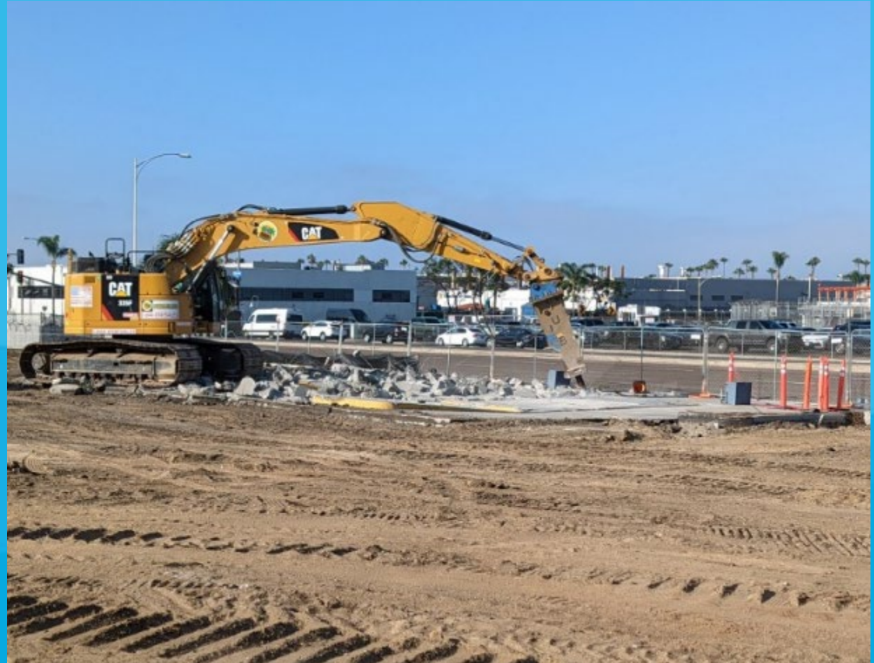
Pavement Demolition and Removal
