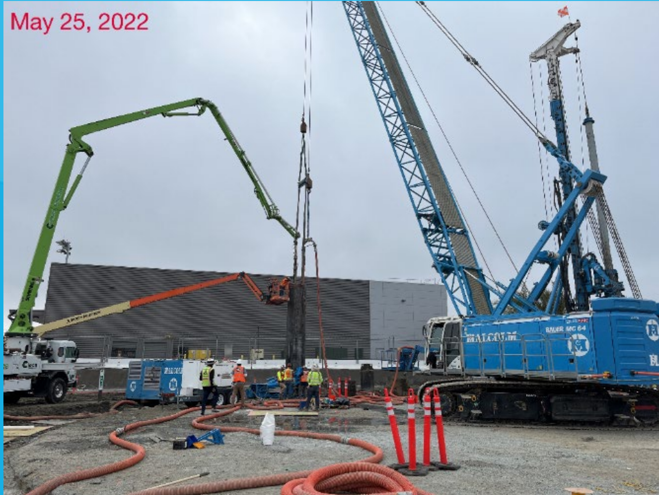
Cistern - Secant Pile Concrete Placement
