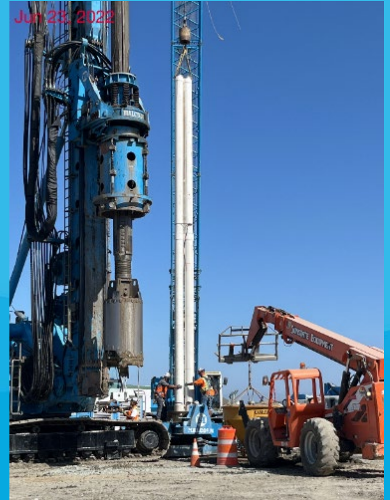
Cistern - Dewatering Well Installation
