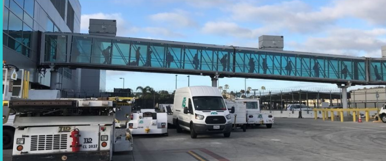
1/5/2021 More Bridge, More Sun
