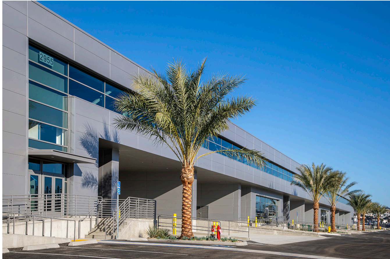
Landside Truck Bays
