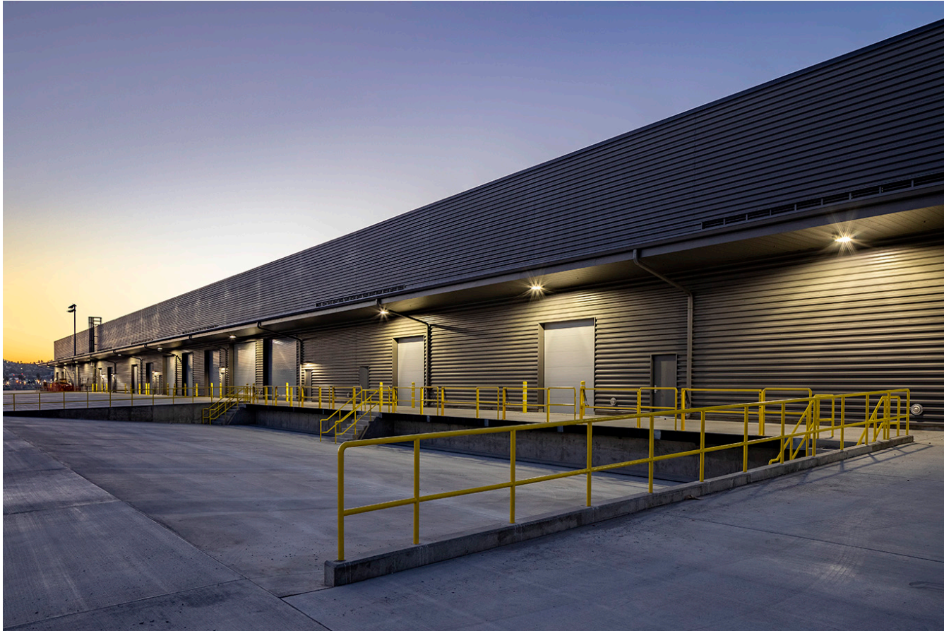
Airside Loading Dock
