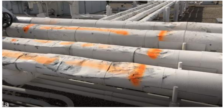
la Metal Jacket Damage & Corrosion
