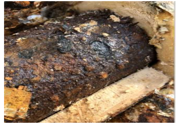
la Metal Jacket Damage & Corrosion
