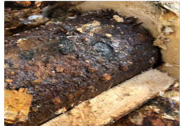
Metal Jacket Damage & Corrosion
