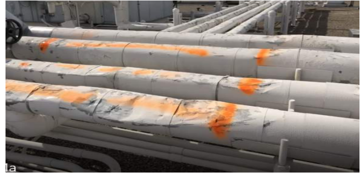
Metal Jacket Damage & Corrosion
