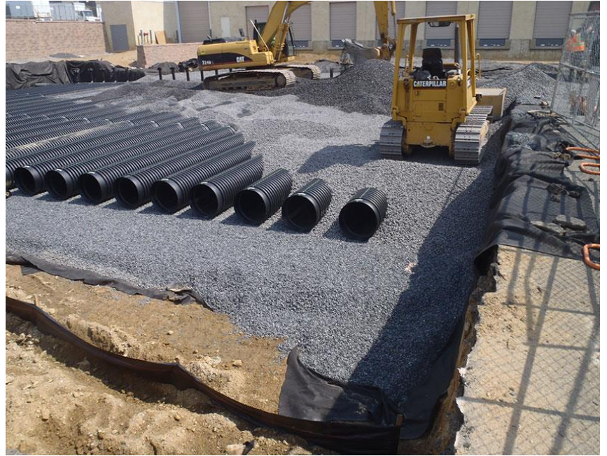
Example of an Infiltration Bed
