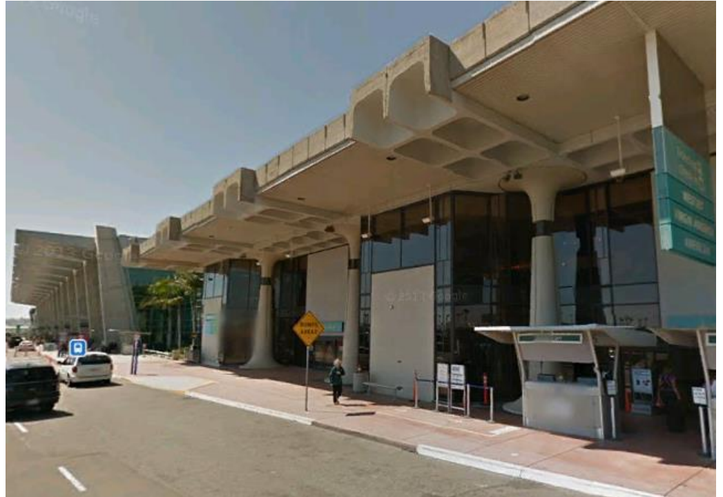
Existing Sidewalk at T2E
