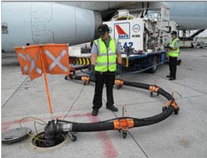
Example of Hydrant Fueling Pit
