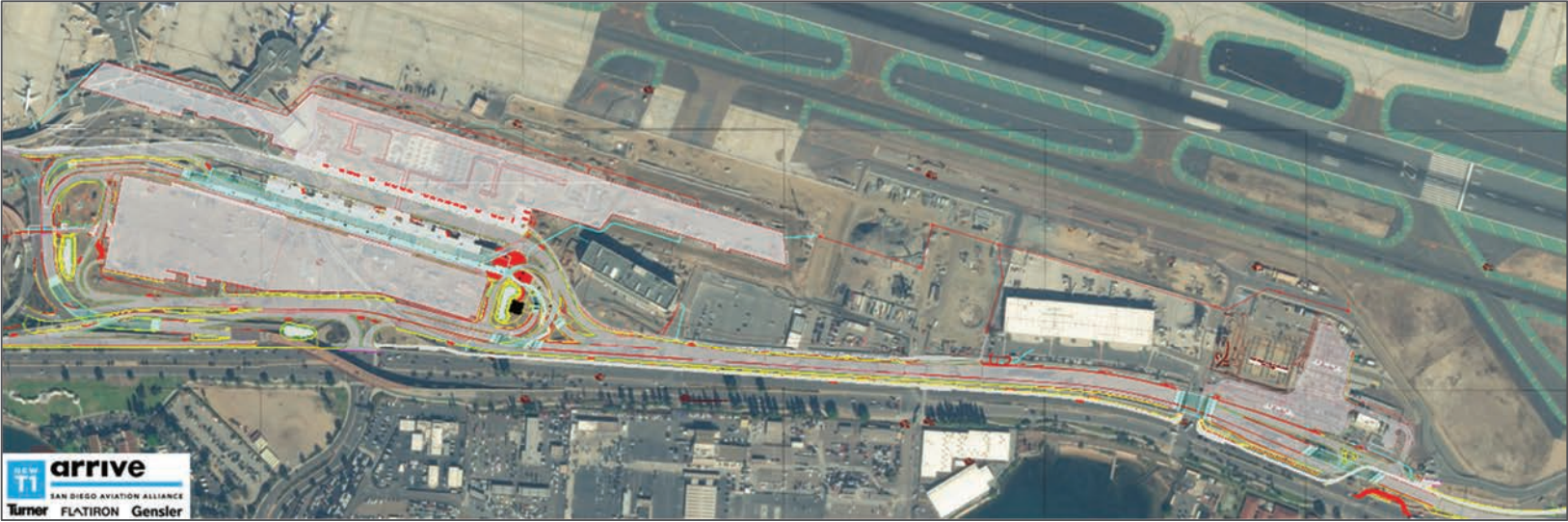
Figure 2 | New T1 Sitework
