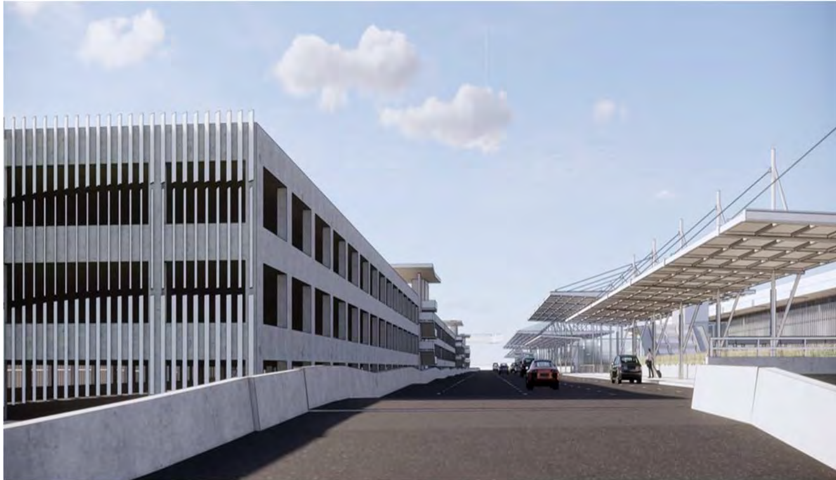
Figure 4 | New Terminal 1 Elevated Departures Roadway
