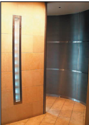
Image 2.3-2 Inside view of curved perforated wall panel at entry/exit
